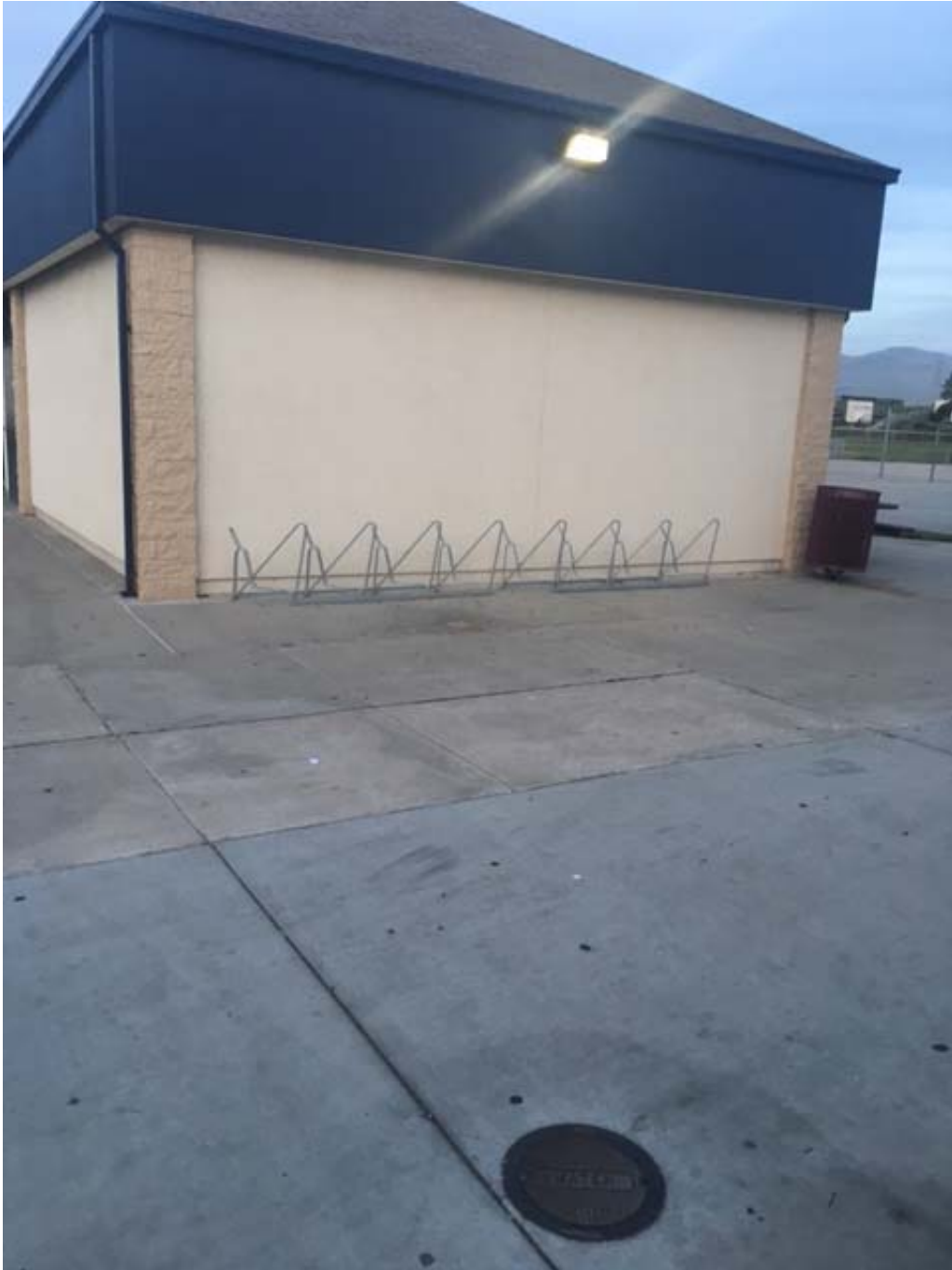
Figure 6 Everett Alvarez High School Bike Racks
