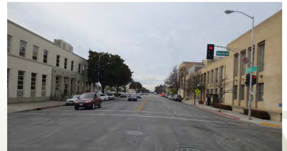
Existing conditions along West Alisal Street, looking west near Government Center. Protected bike lanes and transit islands are proposed for this segment.
