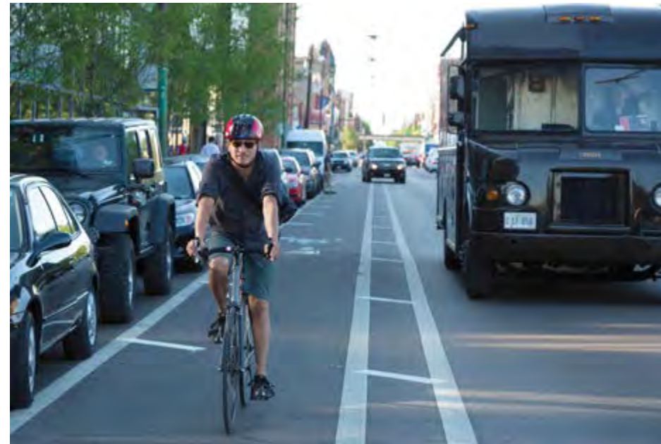
Enhanced bicycle facilities, like Buffered Bike Lanes, provide a more comfortable environment for bicyclists of varying ability levels.
