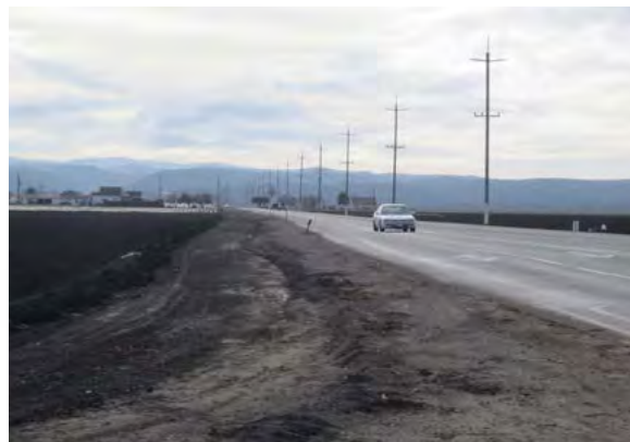
Existing conditions along Davis Road, looking south from Blanco Road. The road is proposed to be widened to 4 lanes, with a two-way cycle track on the east side of the road.
