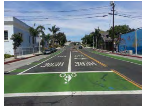
Bike Boxes provide bicyclists with a safe and visible way to get ahead of queuing traffic during the red signal phase
