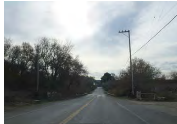
Existing conditions along Davis Road at the Salinas River. A new bridge is proposed along with the widening to four lanes. A two-way cycle track would be provided on the east side of the roadway.
