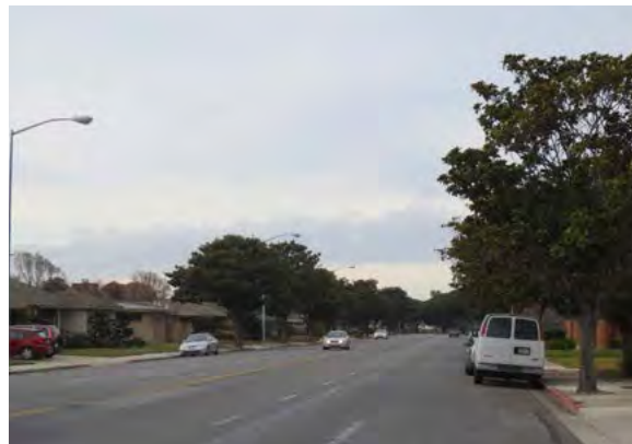
Existing conditions along West Alisal Street, looking west near Hartnell College. A road diet is proposed for this segment to provide bike lanes and a center turn lane.
