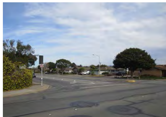
Existing conditions at the West Alisal Street and Blanco Road intersection. Enhanced treatments for transit and bicyclists are proposed at this intersection, including transit signal priority and a bike signal.
