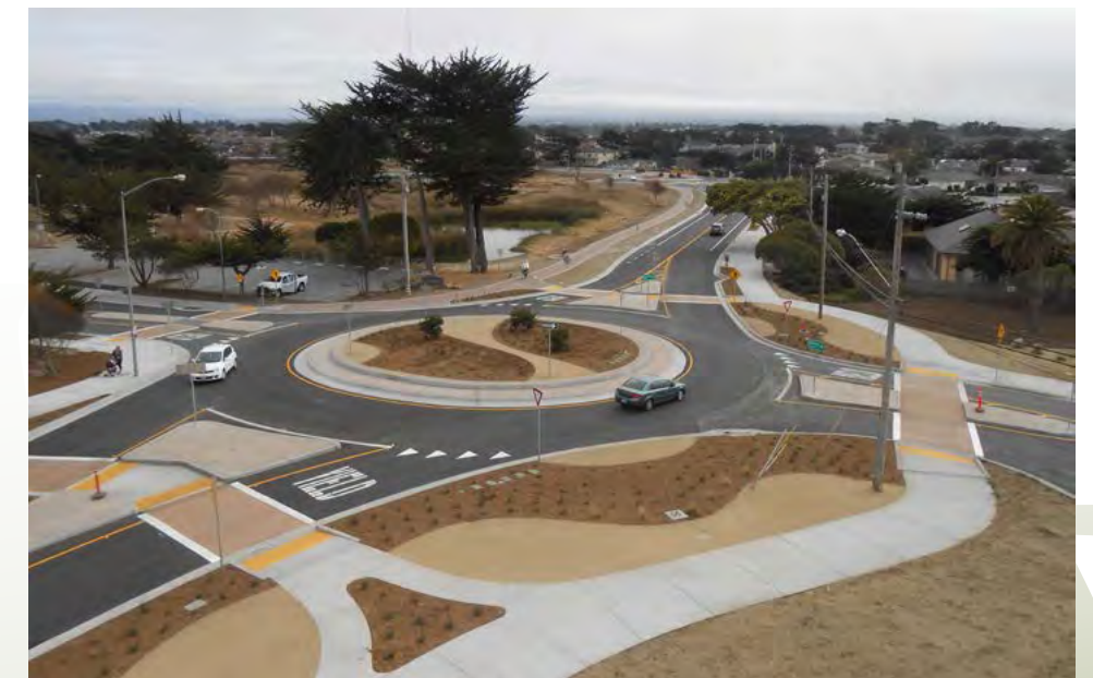
Two roundabouts have been recently constructed along Reservation Road in the City of Marina
