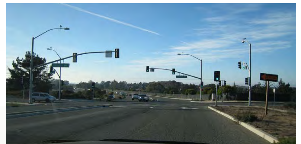
Existing conditions on Imjin Road near California Avenue. Bus-only lanes are proposed to be added in addition to a wider mixed-use path on the south side of the roadway.
