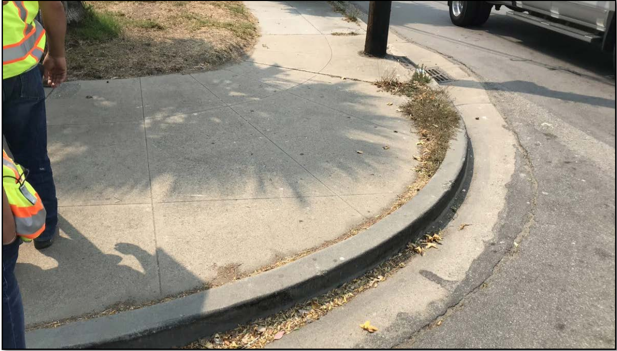
Before photo of Polk St JOC Sidewalk Repair
