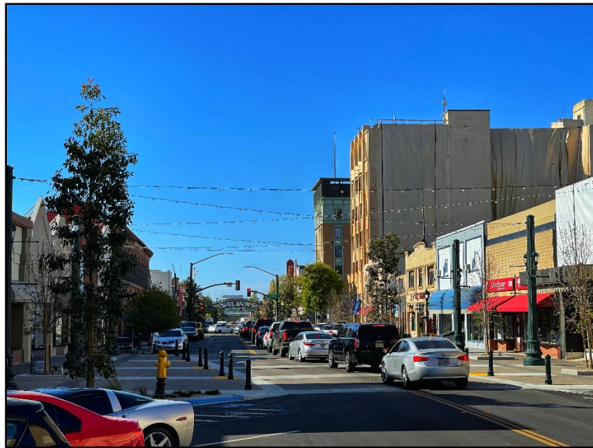
After: 300 Block Plaza Area Facing North
