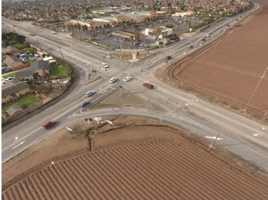
Existing Natividad/Boronda Intersection
