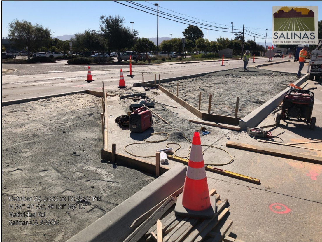
Construction Photo: Staking new pedestrian refuge island on Natividad Rd at Pacheco St
