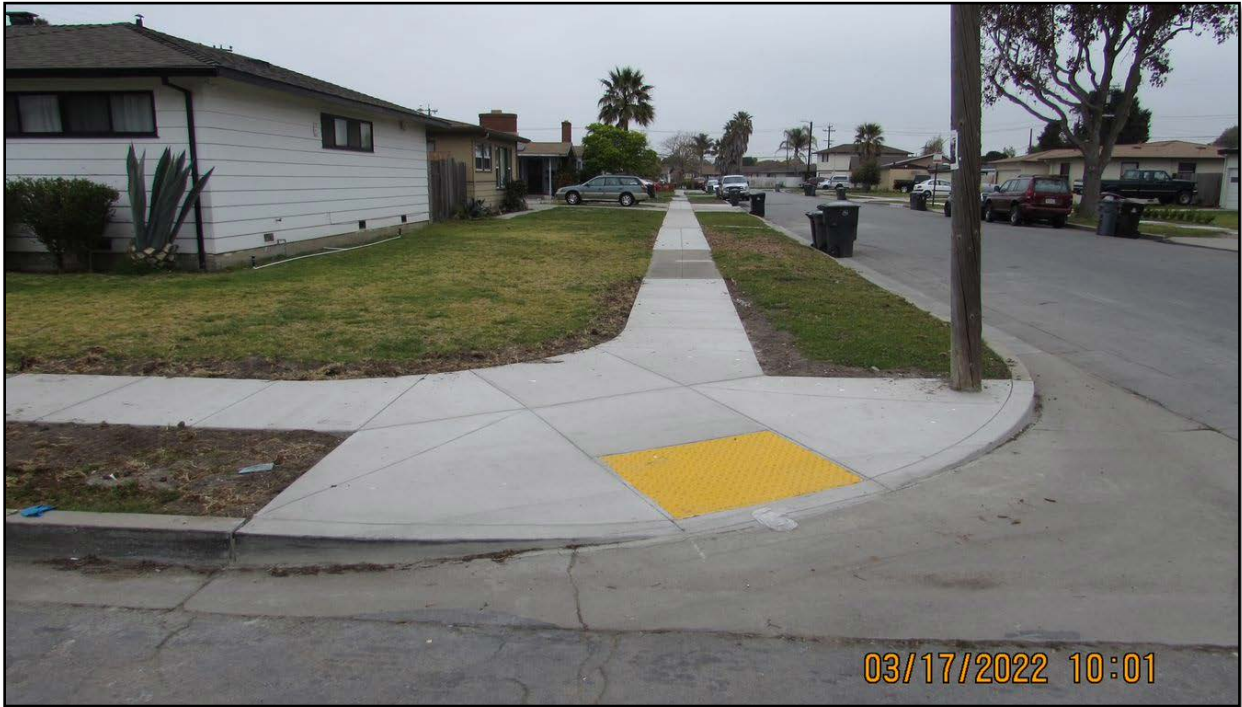
After photo of Polk St JOC Sidewalk Repair
