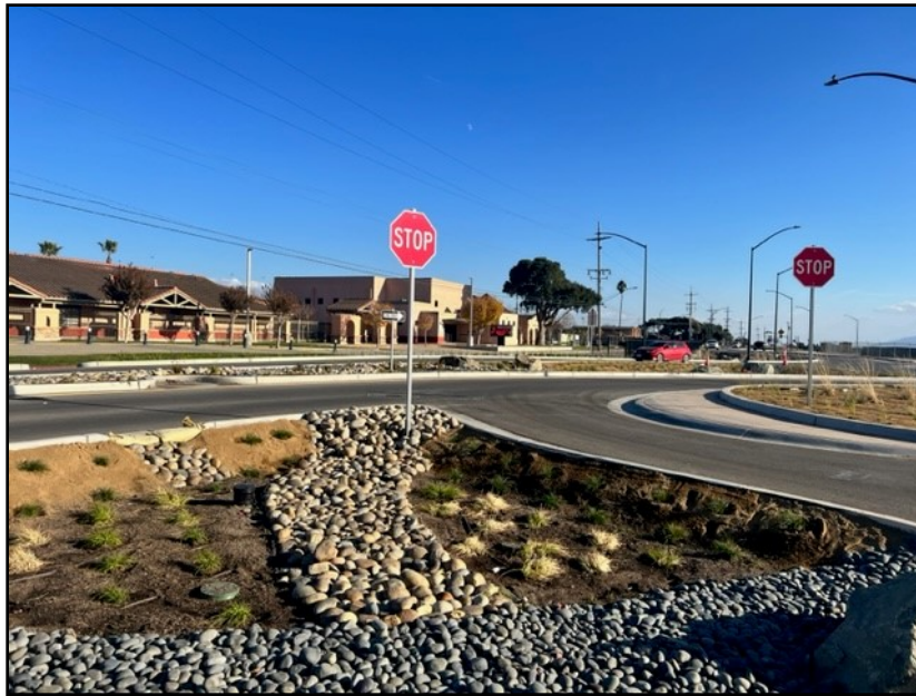
Bardin Road/Alisal St/Alisal Road intersection
