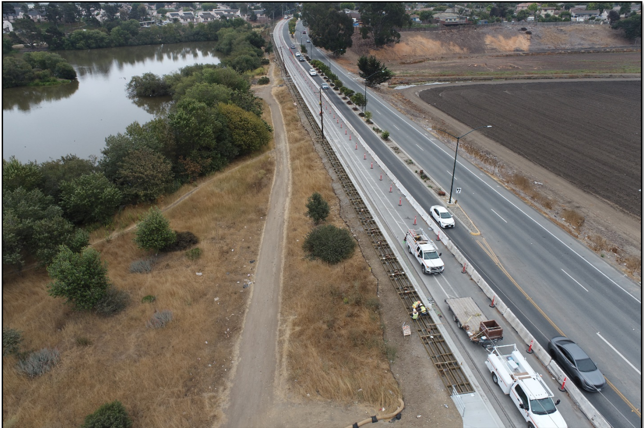
Laurel Boardwalk construction
