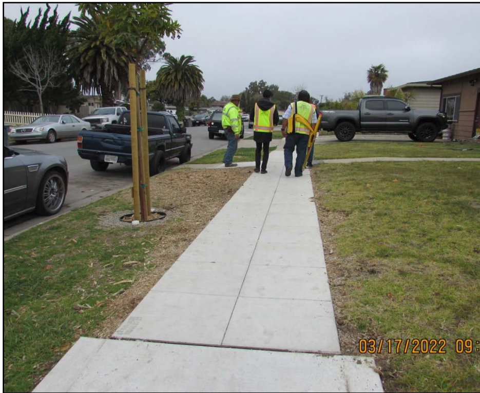
After photo of Polk St JOC Sidewalk Repair
