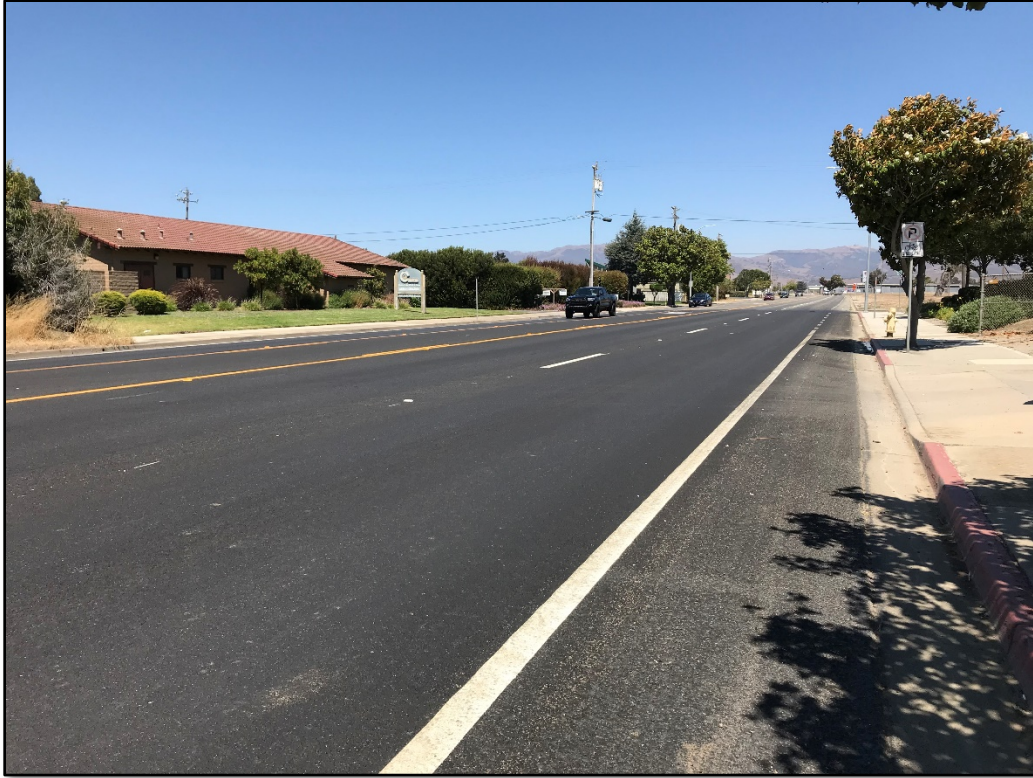
After photo of Airport Blvd.
