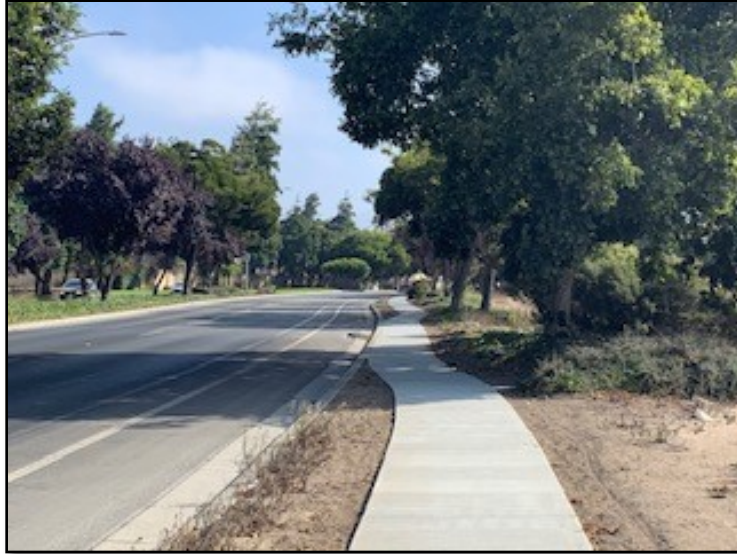
Constitution Blvd looking North – New sidewalk
