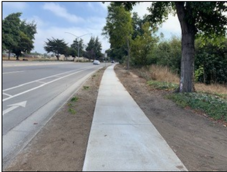
Constitution Blvd looking North – New sidewalk
