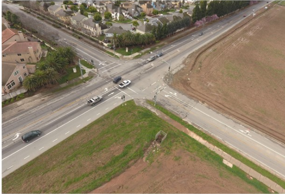
Existing McKinnon/Boronda Intersection
