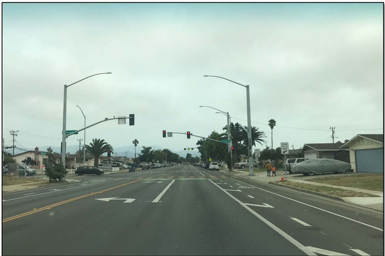
After Photo: Eastbound Alvin Dr at El Dorado: new signal, road diet, and bike boxes
