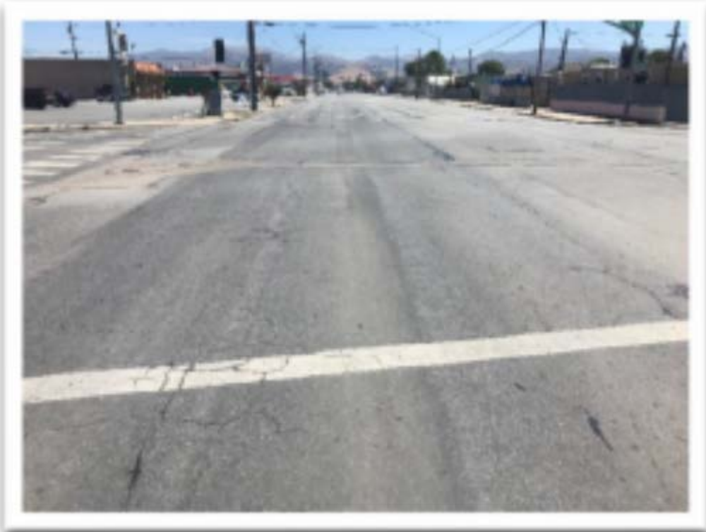
Williams Road @ E. Market Street West Bound facing East
