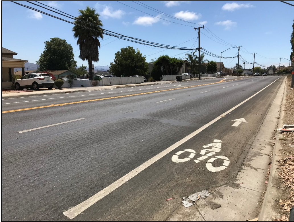
After photo of East Bernal Rd.
