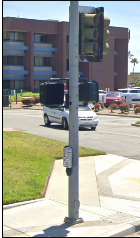
After Photo: Accessible Pedestrian Push Button at Northridge Main Entrance
