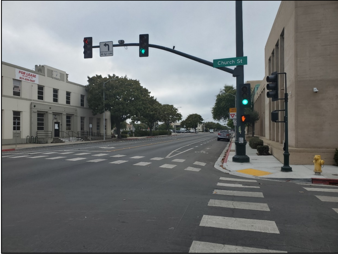
After Construction: New signal with protected left phasing at Alisal St and Church St
