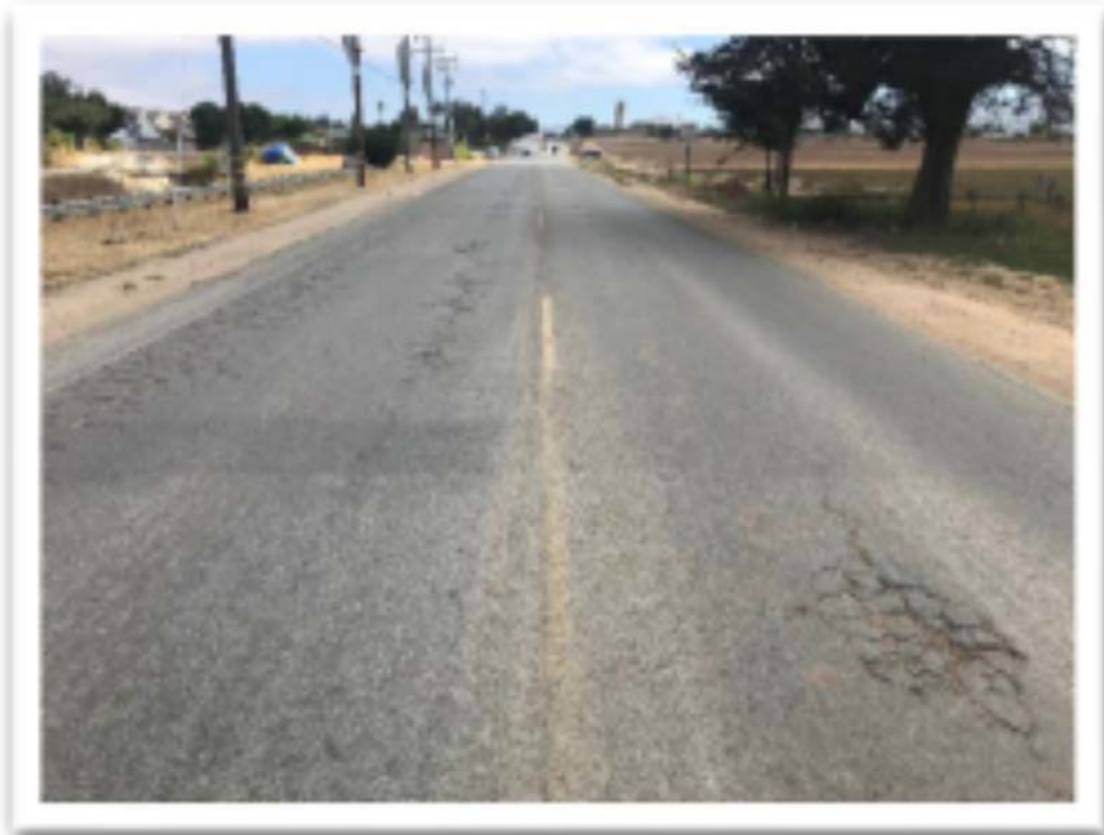
San Juan Grade Road @ ~1,500' North of Van Buren Avenue facing North
