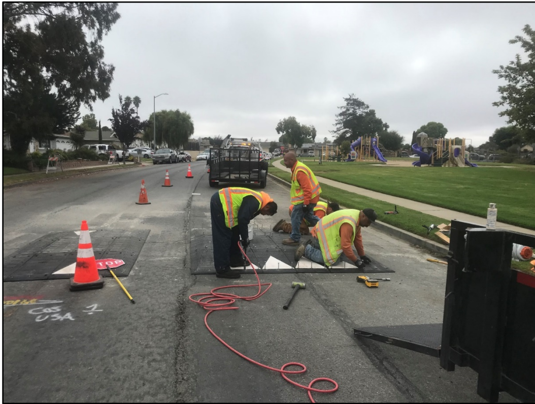
Construction Photo: East Bolivar Street traffic calming installation
