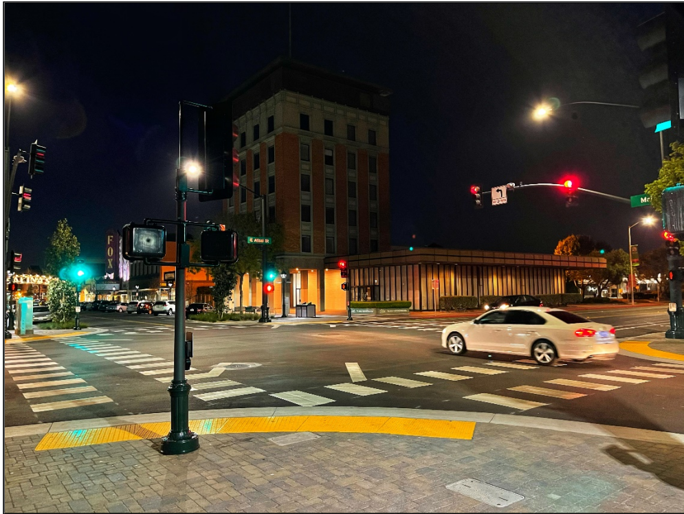
After Construction: New signal with a pedestrian scramble at Alisal St and Main St
