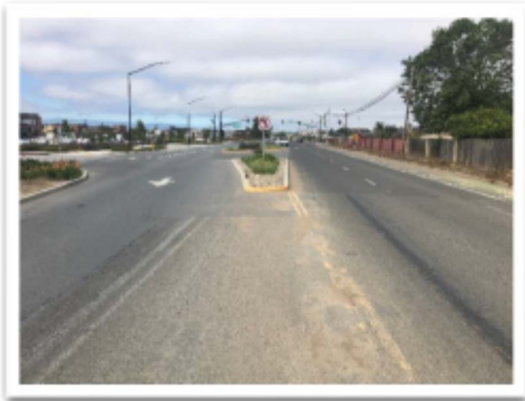
San Juan Grade Road @ 120' N/O Northridge Drive facing South
