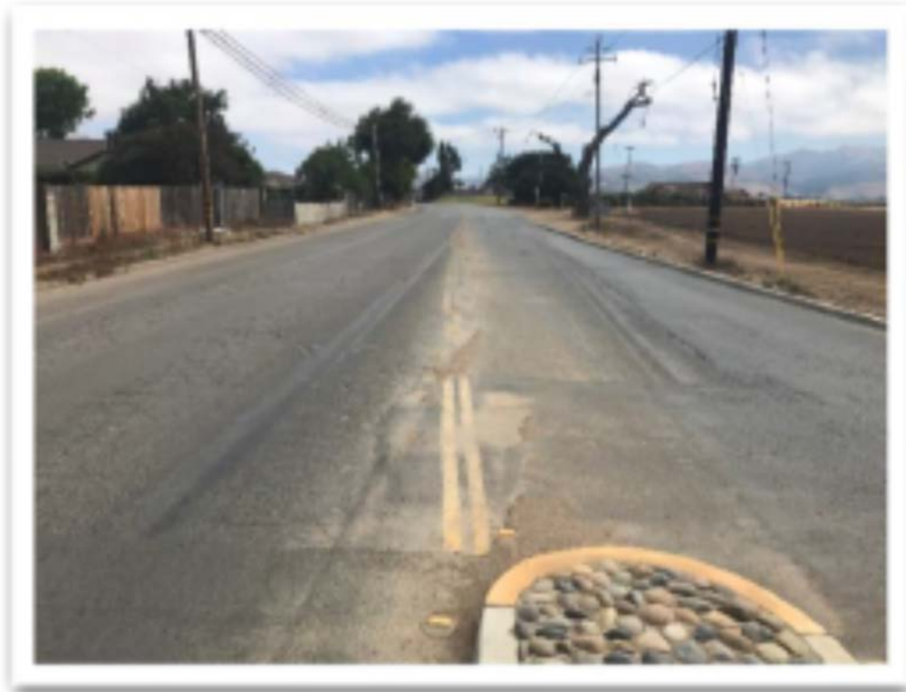
San Juan Grade Road @ 120' N/O Northridge Drive facing North
