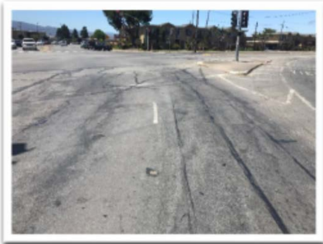
Williams Road @ E. Alisal Street West Bound facing West
