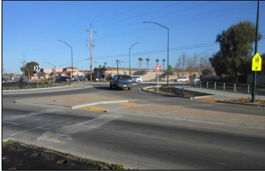
During Contrsution: Alisal Road near Sconberg Parkway
