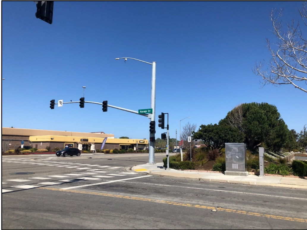
After Construction Photo: New signal facing northbound
