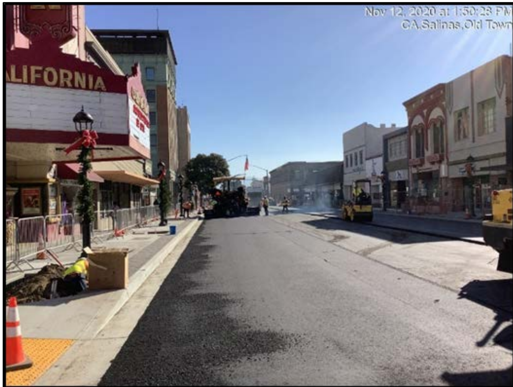
Construction Photo: 200 Block – Placing New Pavement
