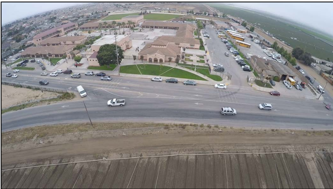
2017 Aerial view of Bardin Road/Alisal St/Alisal Road intersection
