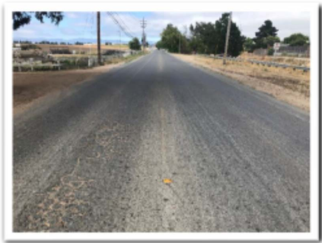
San Juan Grade Road @ ~1,500' North of Van Buren Avenue facing South
