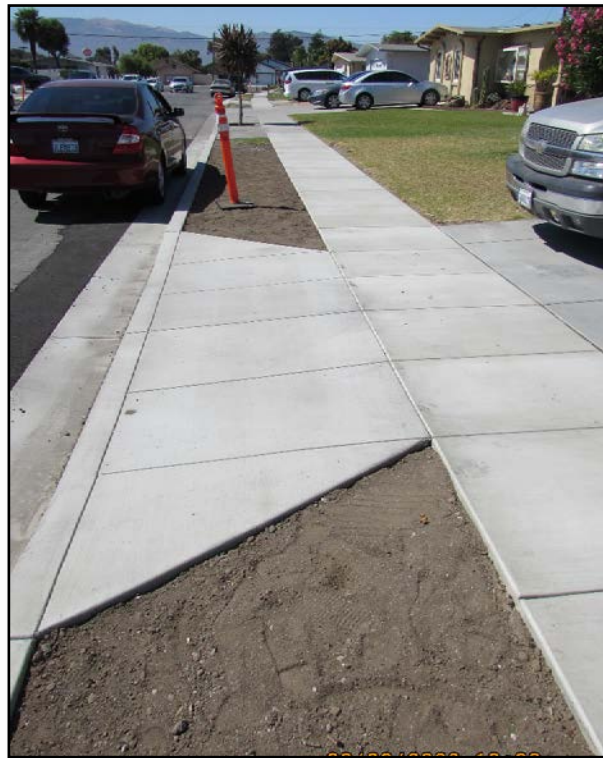
After photos of S Filice St JOC Sidewalk Repair
