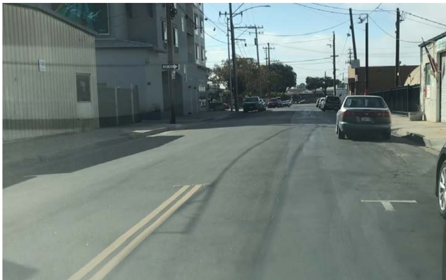
After Photo: Pavement Repair at E Lake Street
