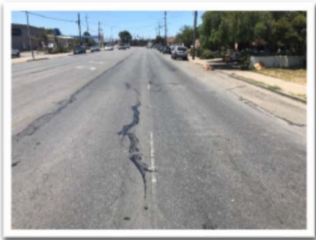
Williams Road @ Quilla Street West Bound facing West
