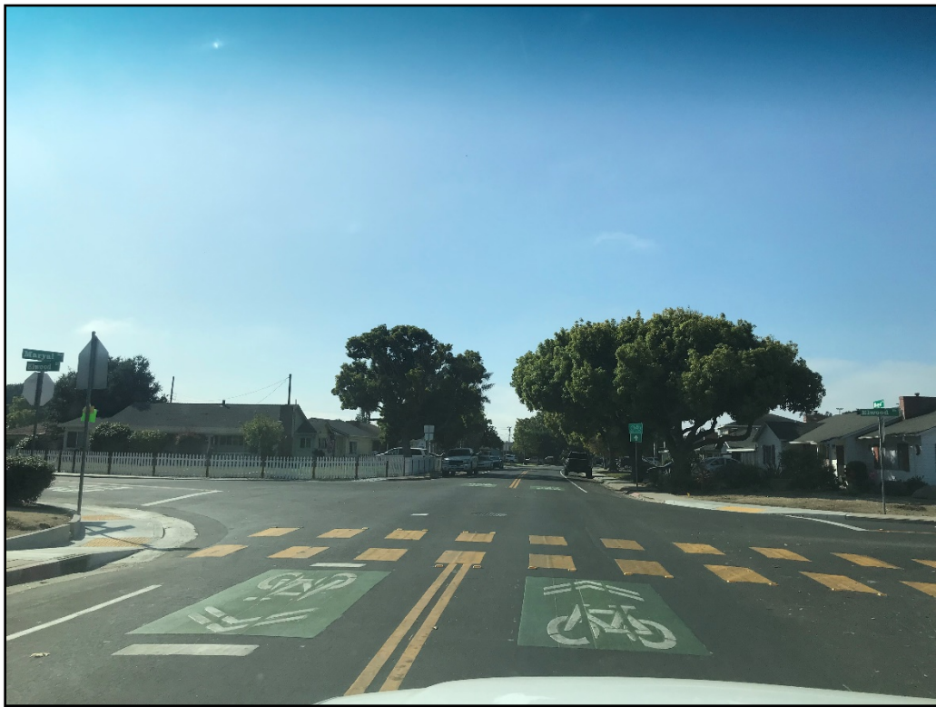
After Construction – New Striping on Maryal Dr
