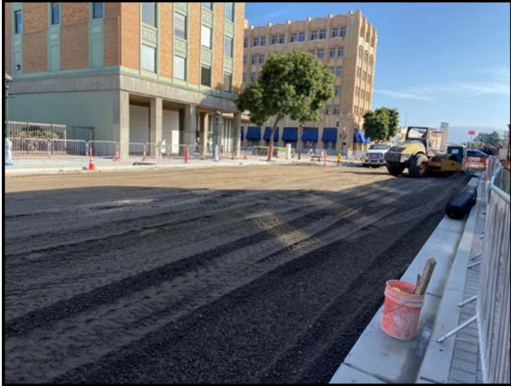
Construction Photo: Grading for New Roadway Pavement
