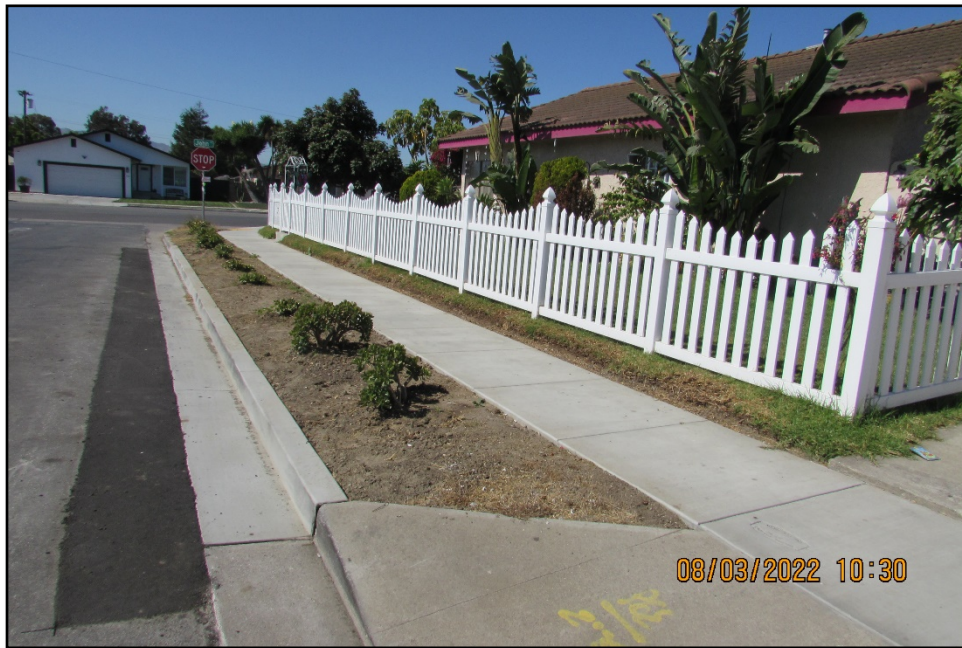
After photo of S Filice St JOC Sidewalk Repair
