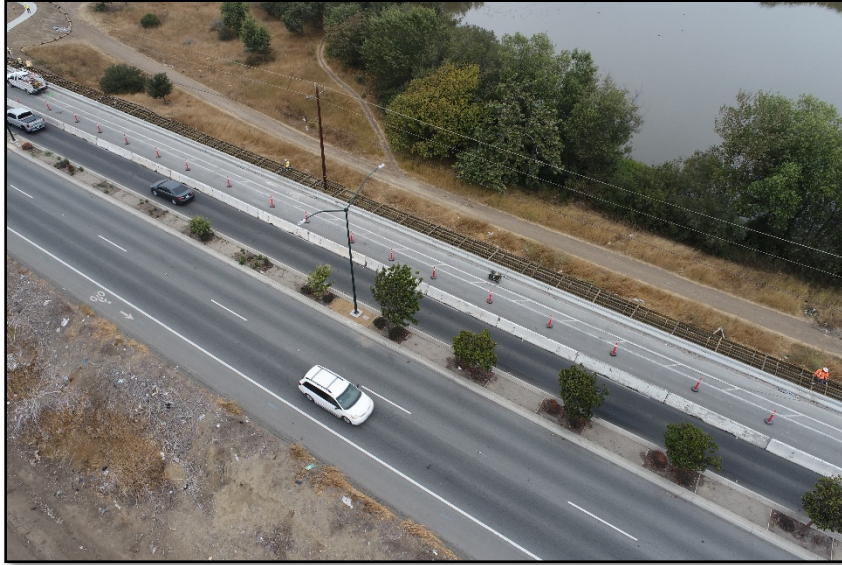
View of the pedestrian boardwalk under construction.
