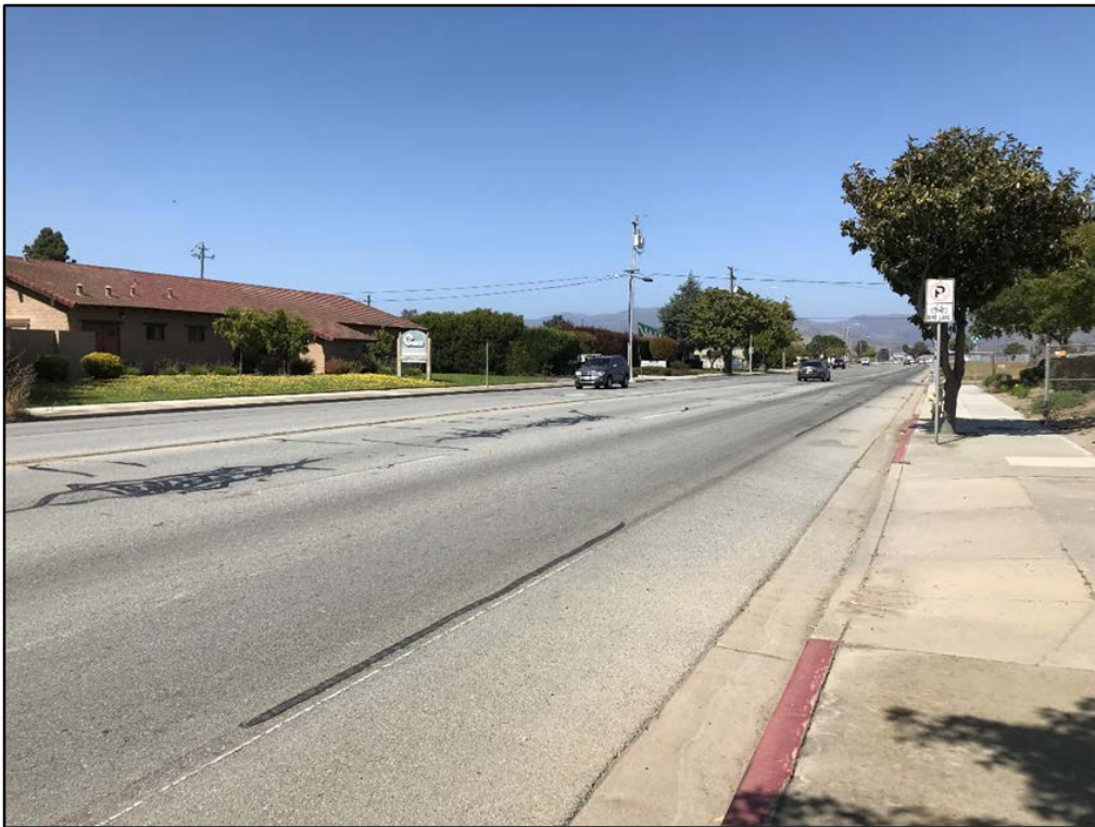
Before photo of Airport Blvd.
