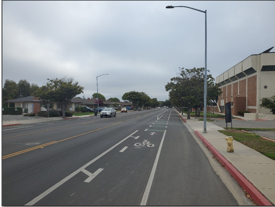
After Construction: New buffered bike lanes and road diet in front of Hartnell College
