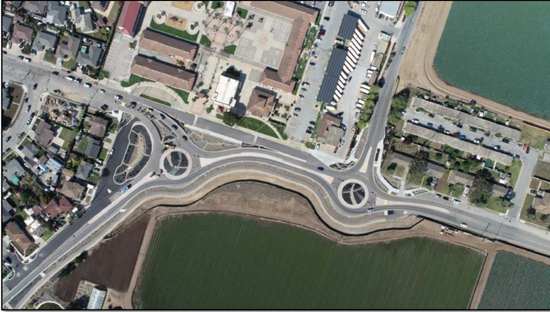
Bardin Road/Alisal St/Alisal Road intersection April 2022
