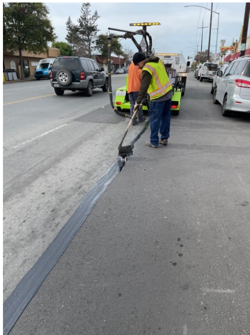
Crack Sealing along E. Alisal Street
