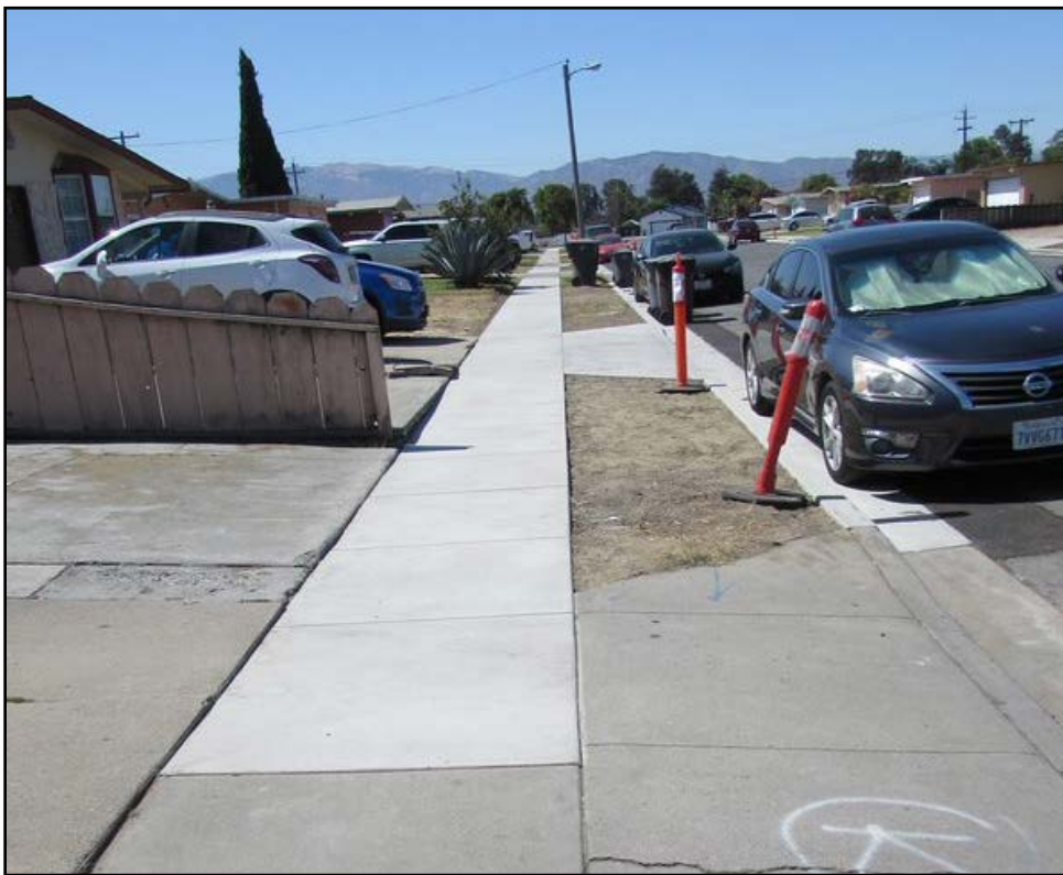
After photo of S Filice St JOC Sidewalk Repair
