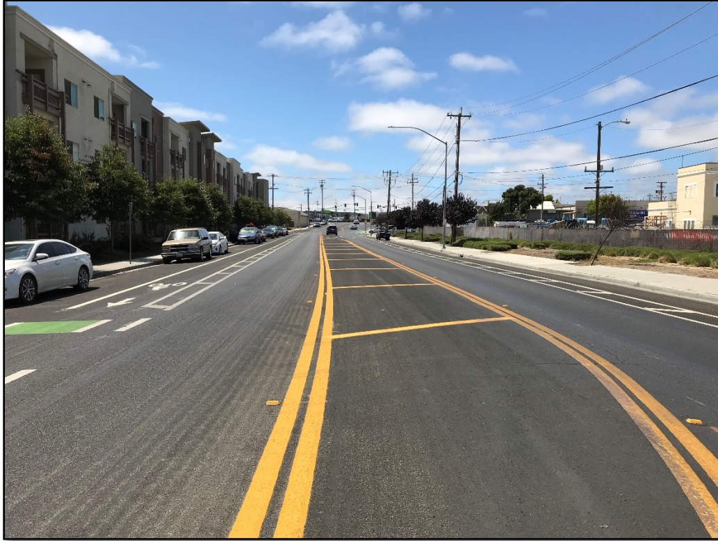
After photo at East Rossi St.
