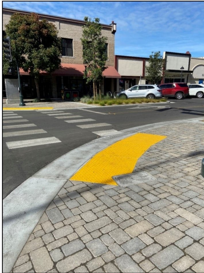
Main St at San Luis St: After Completion
