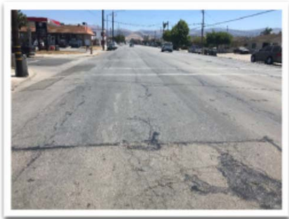
Williams Road @ Grandhaven Street West Bound facing East
