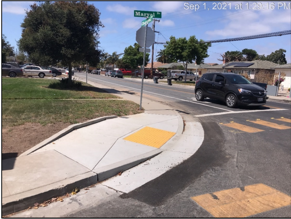
After Construction – New ADA ramp at Maryal Dr and Chaparral St
