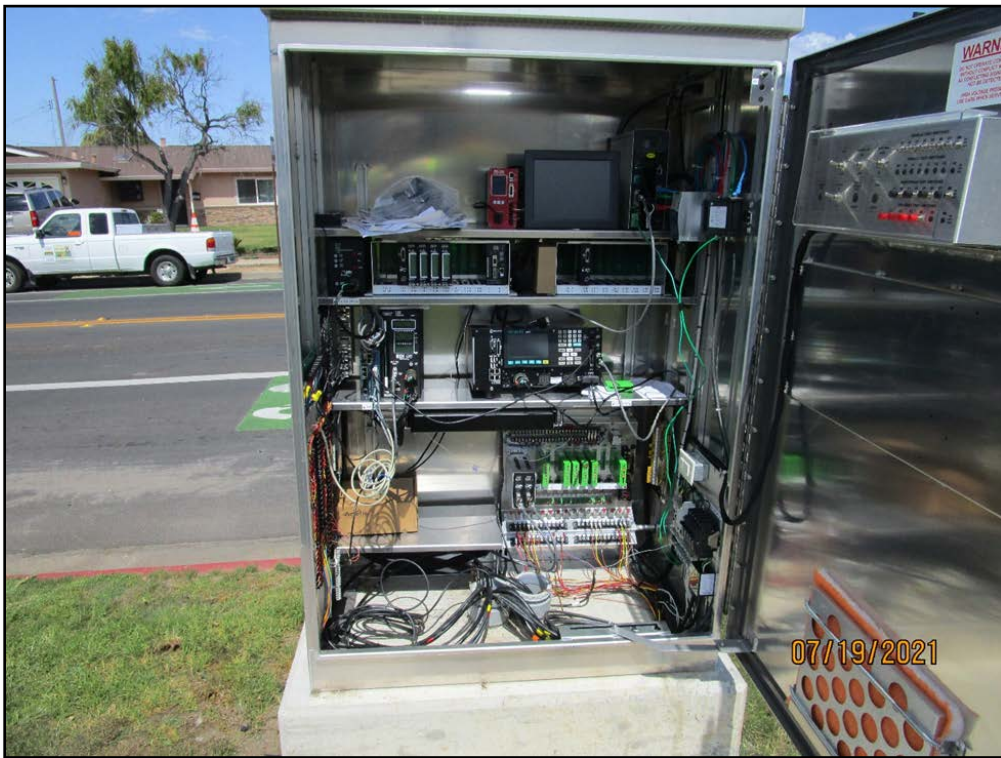
Construction Photo: New controller cabinet at Alvin Dr and Linwood Dr
