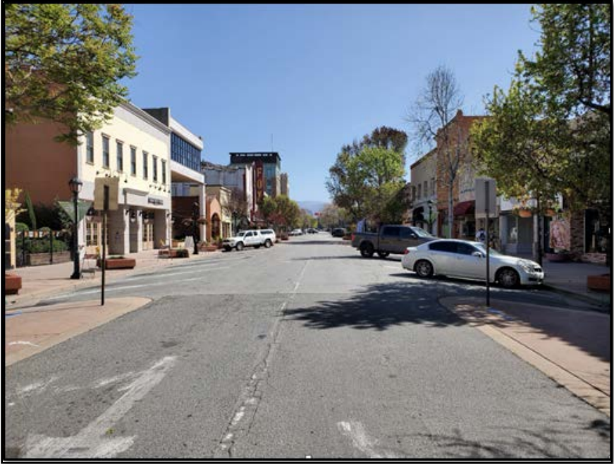
Before: 200 Block Facing South
