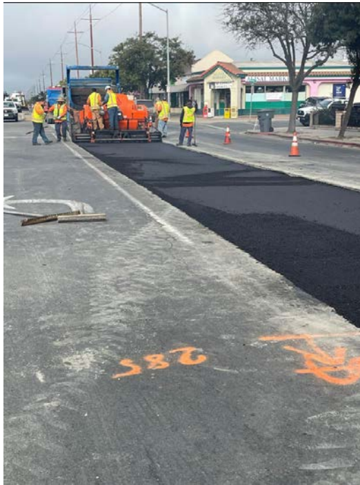
Pavement Maintenance at E. Alisal Street
