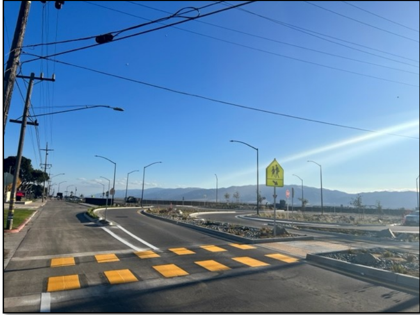
Bardin Road/Alisal St/Alisal Road intersection
