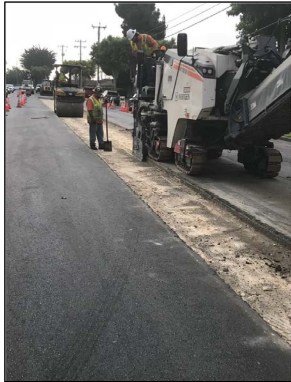
Pavement maintenance at E. Romie Lane near San Marino Way
