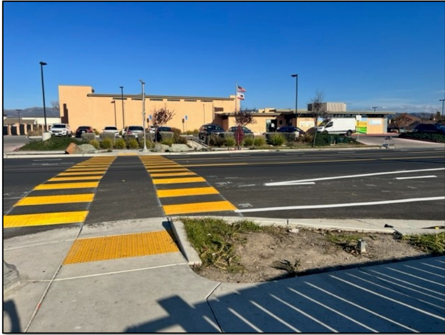
After: Bardin Road @ Toro Ave facing West
