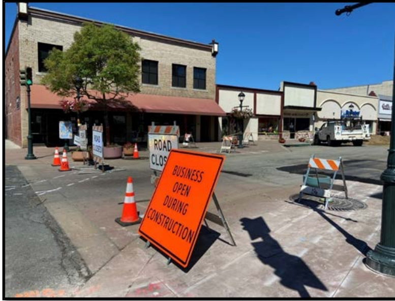
Main St at San Luis St: During Construction
