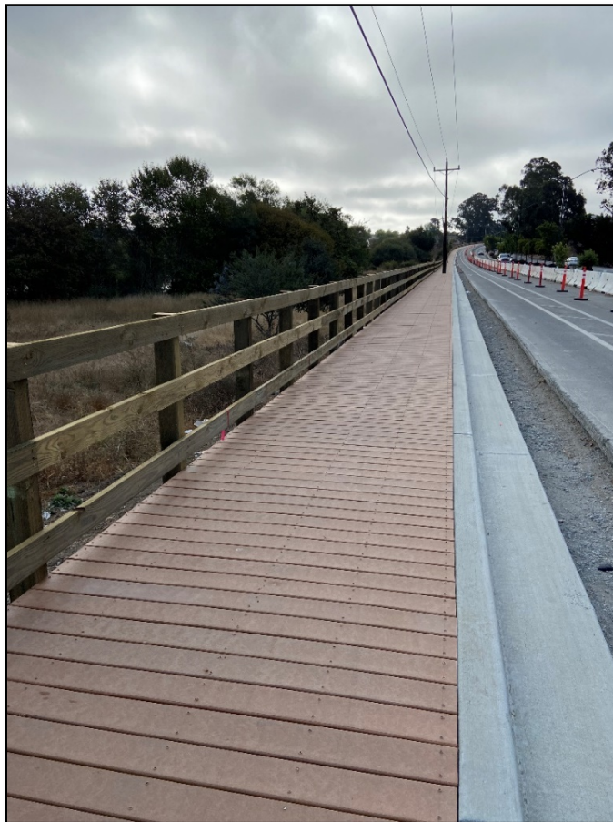
Pedestrian boardwalk completed.
