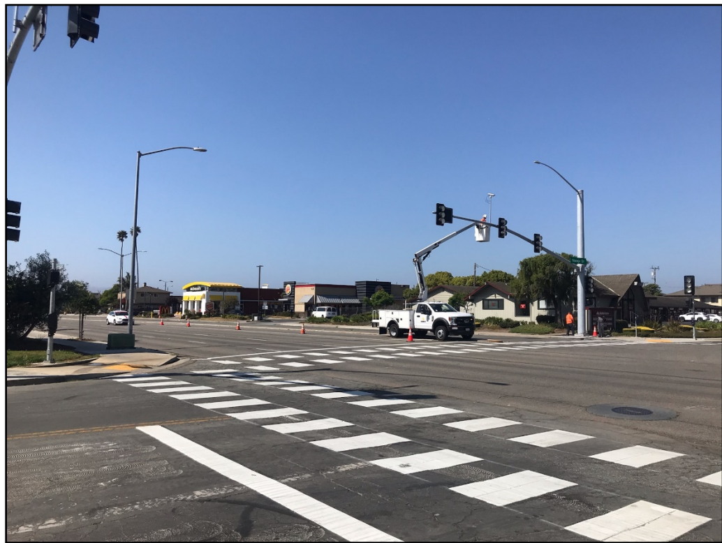
Construction Photo: Installing the Video Detection Cameras
