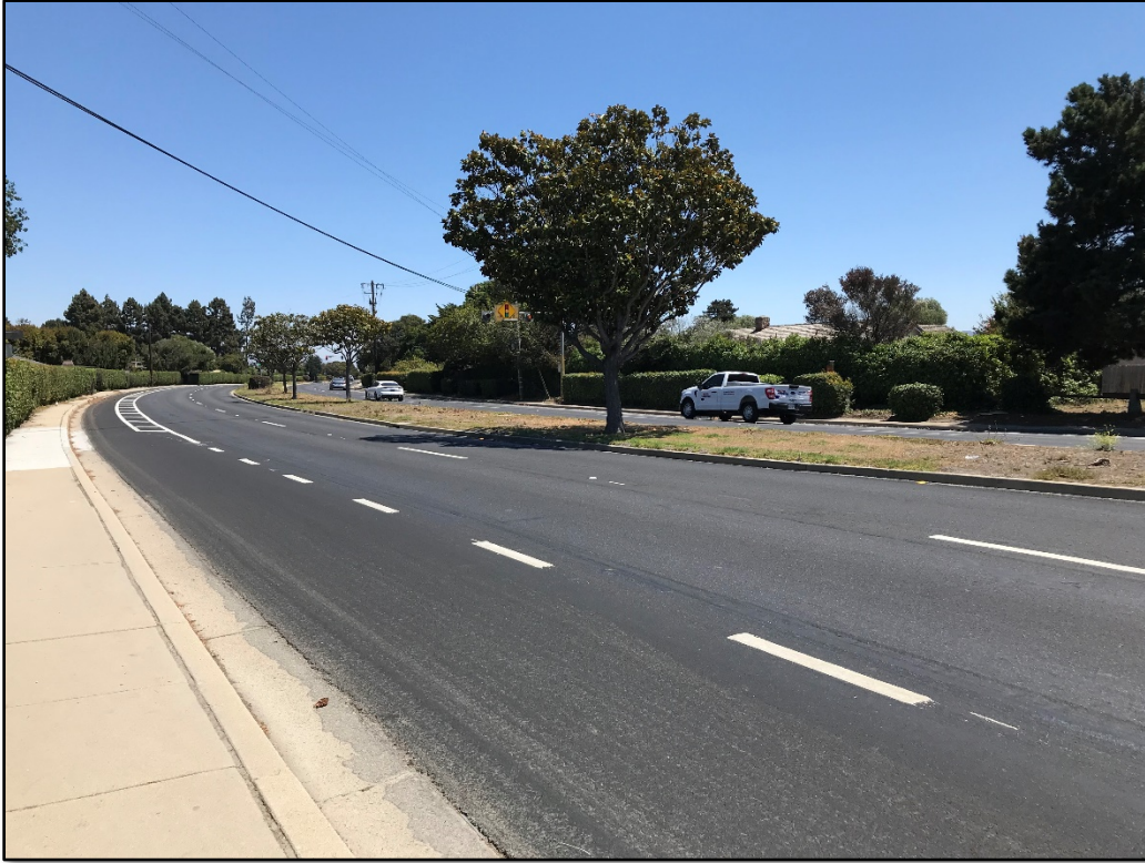
After photo of W Blanco Rd.
