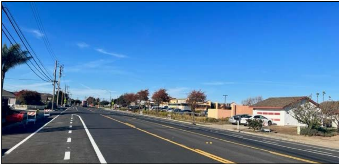
After: Bardin Road @ Afton Road South Bound facing South
