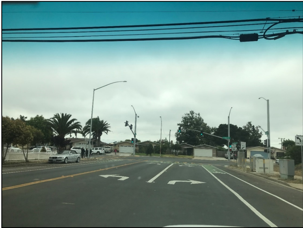
After Construction – New Signal at Alvin Drive and El Dorado Dr
