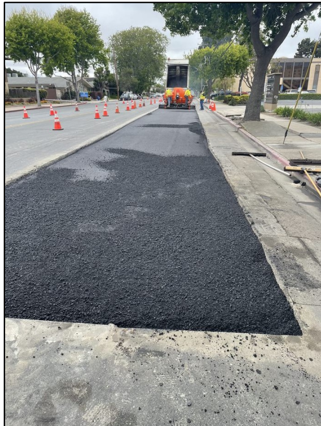
Pavement maintenance at E. Romie Lane
