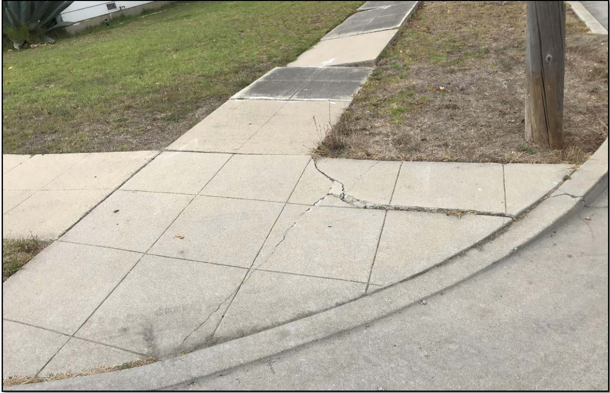
Before photo of Polk St JOC Sidewalk Repair
