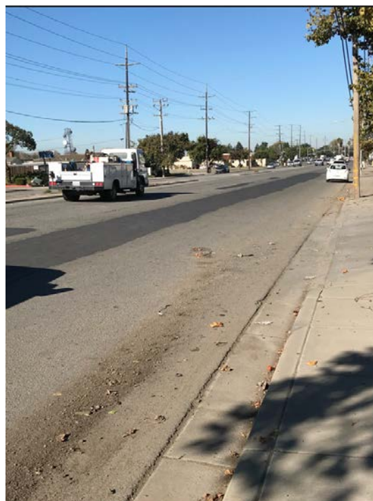
AfterPhoto: Patch and repair work at Abbott Street
