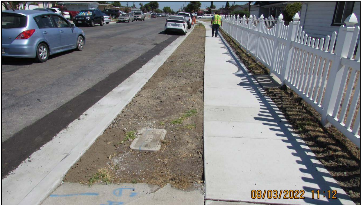
After photo of S Filice St JOC Sidewalk Repair
