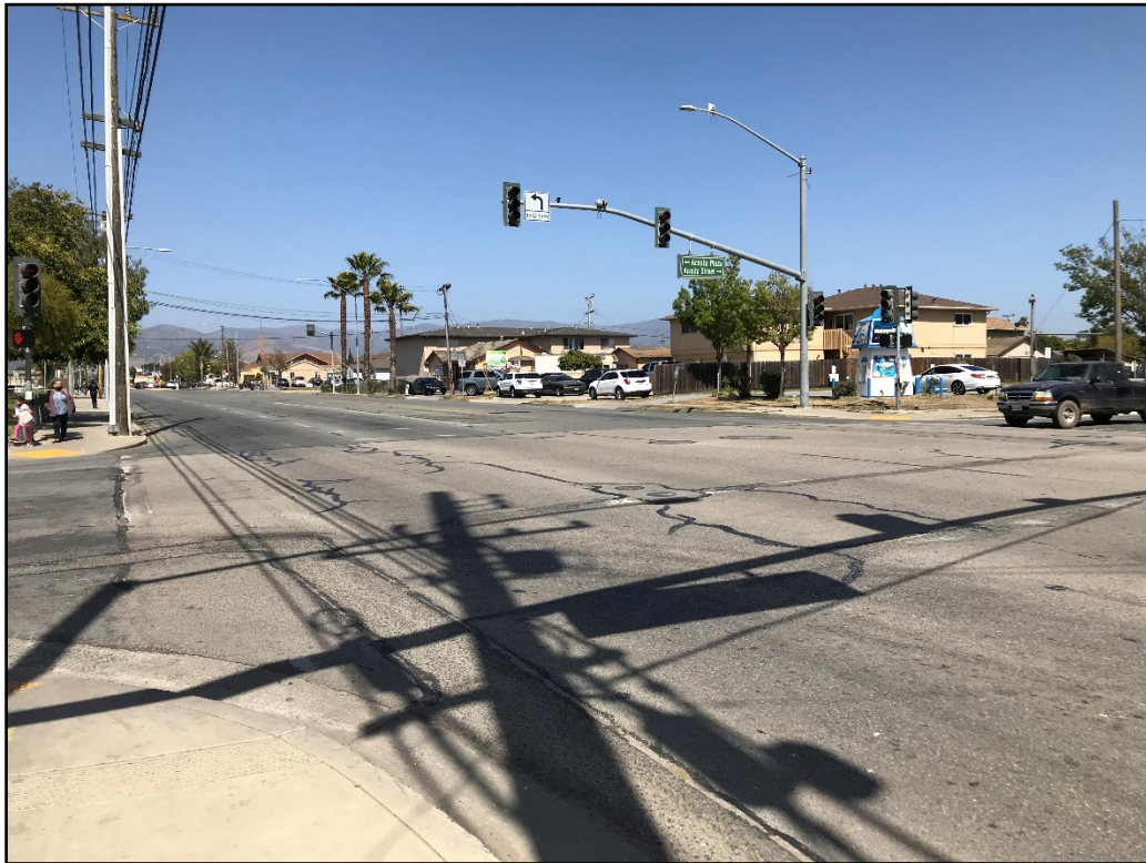
Before photo of N. Sanborn Rd at Acosta Plaza
