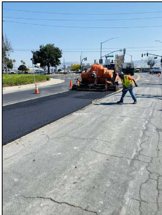
Pavement maintenance at E. Romie Lane near Abbott Street
