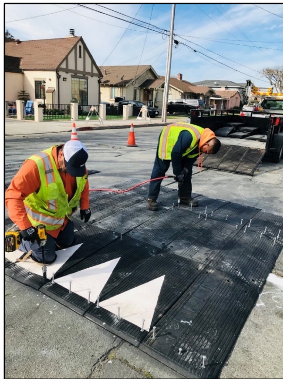
Construction Photo: Geil Street traffic calming installation
