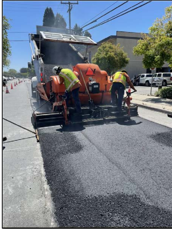
Pavement maintenance at E. Romie Lane near San Marino Way
