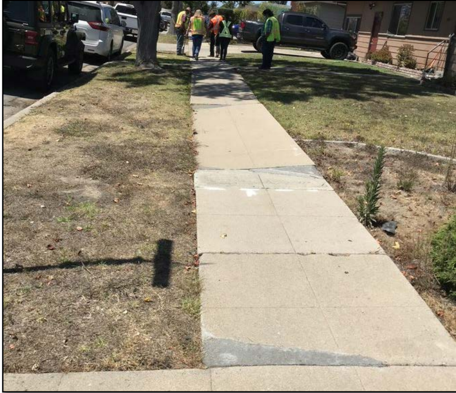
Before photo of Polk St JOC Sidewalk Repair
