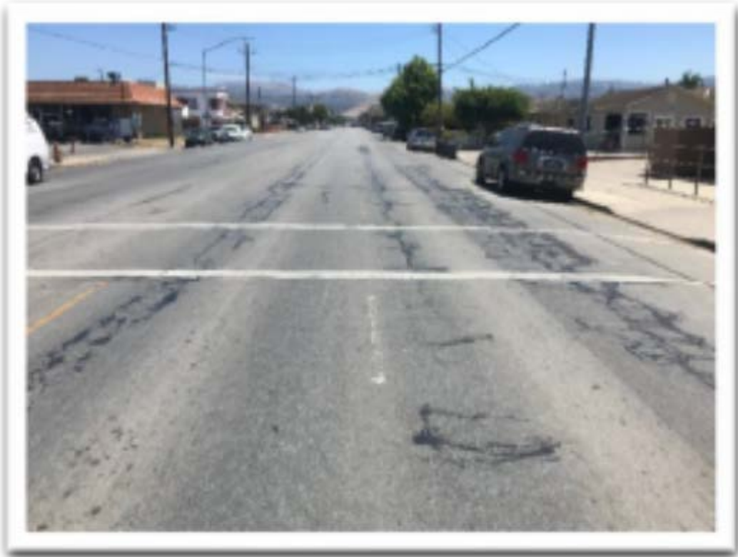
Williams Road @ Grandhaven Street East Bound facing East
