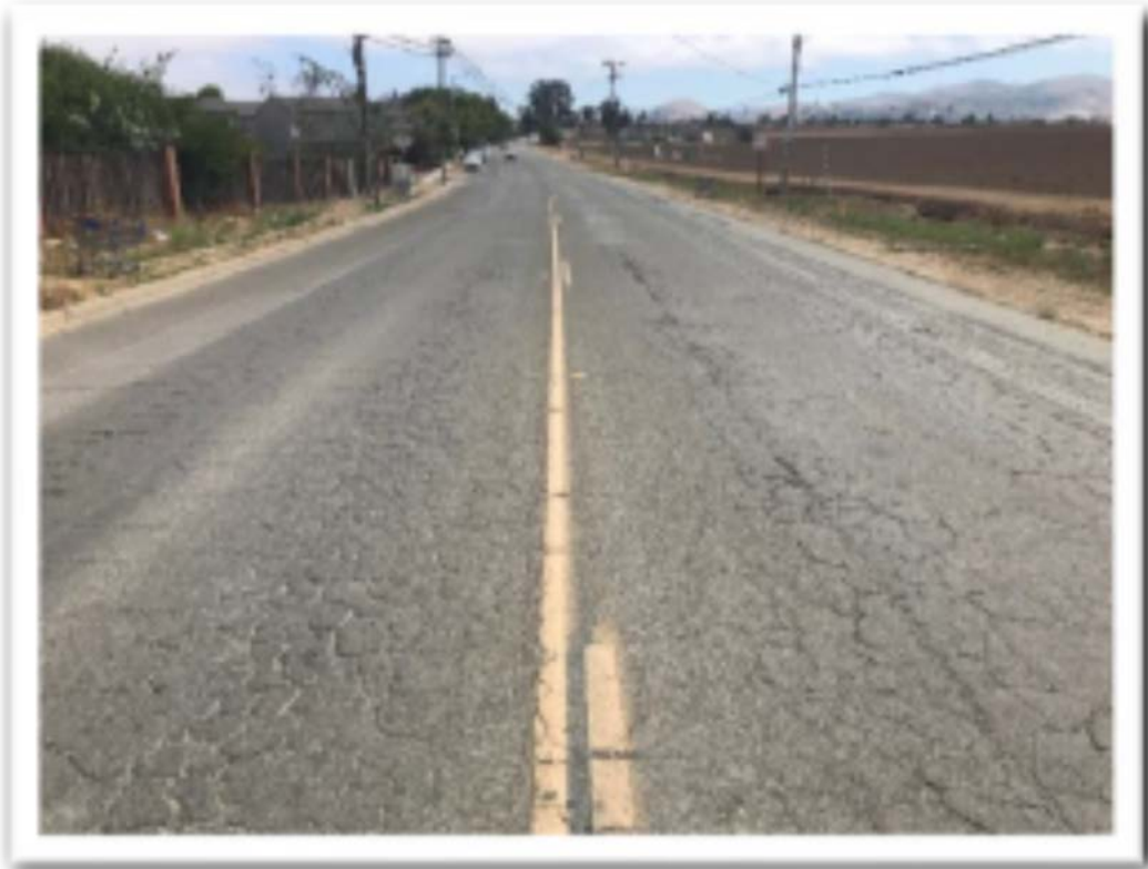
San Juan Grade Road @ Van Buren Avenue facing North
