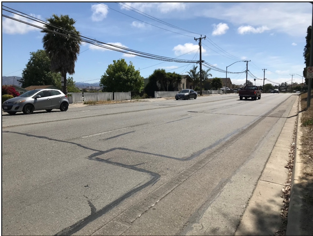
Before photo of East Bernal Rd.
