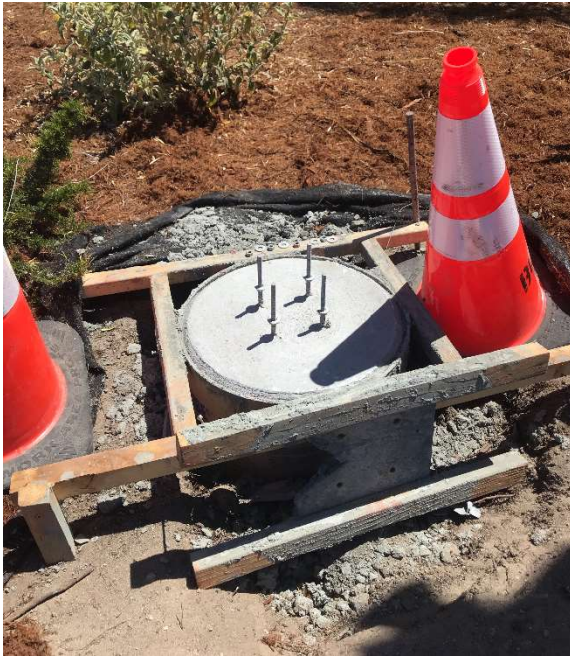
Wayfinding sign foundation construction
