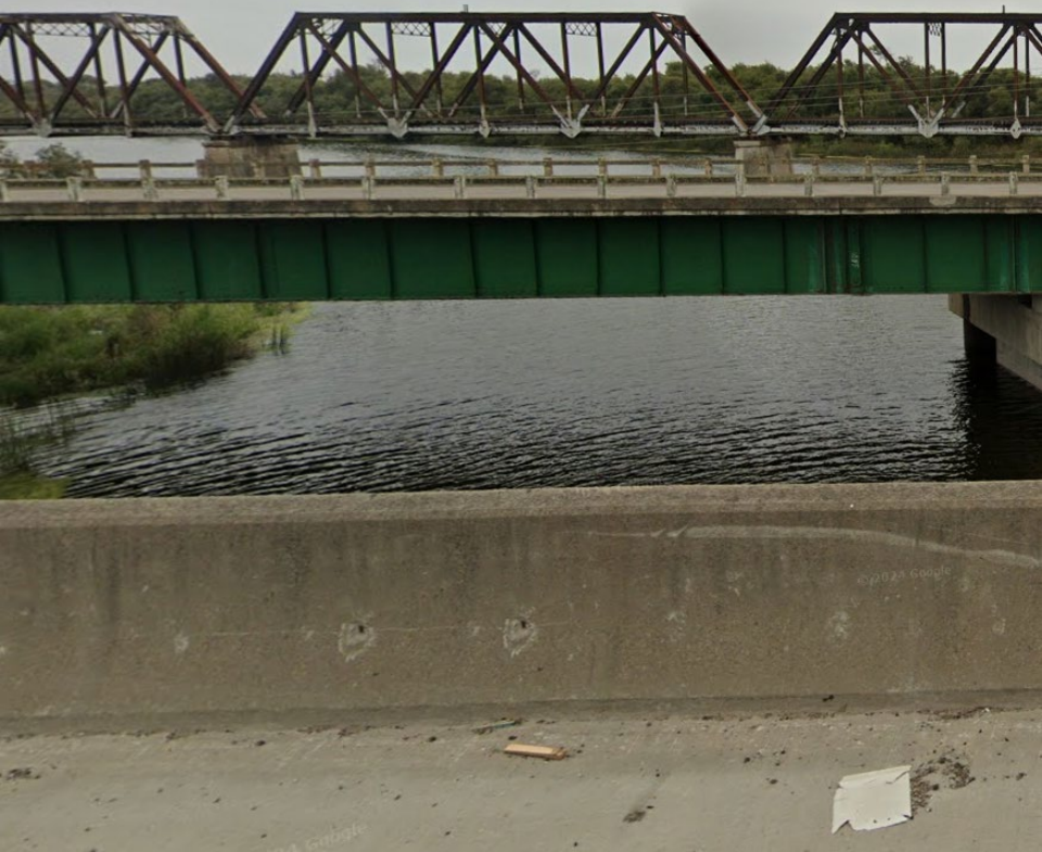
Salinas River Bridge Replacement Phase 2
