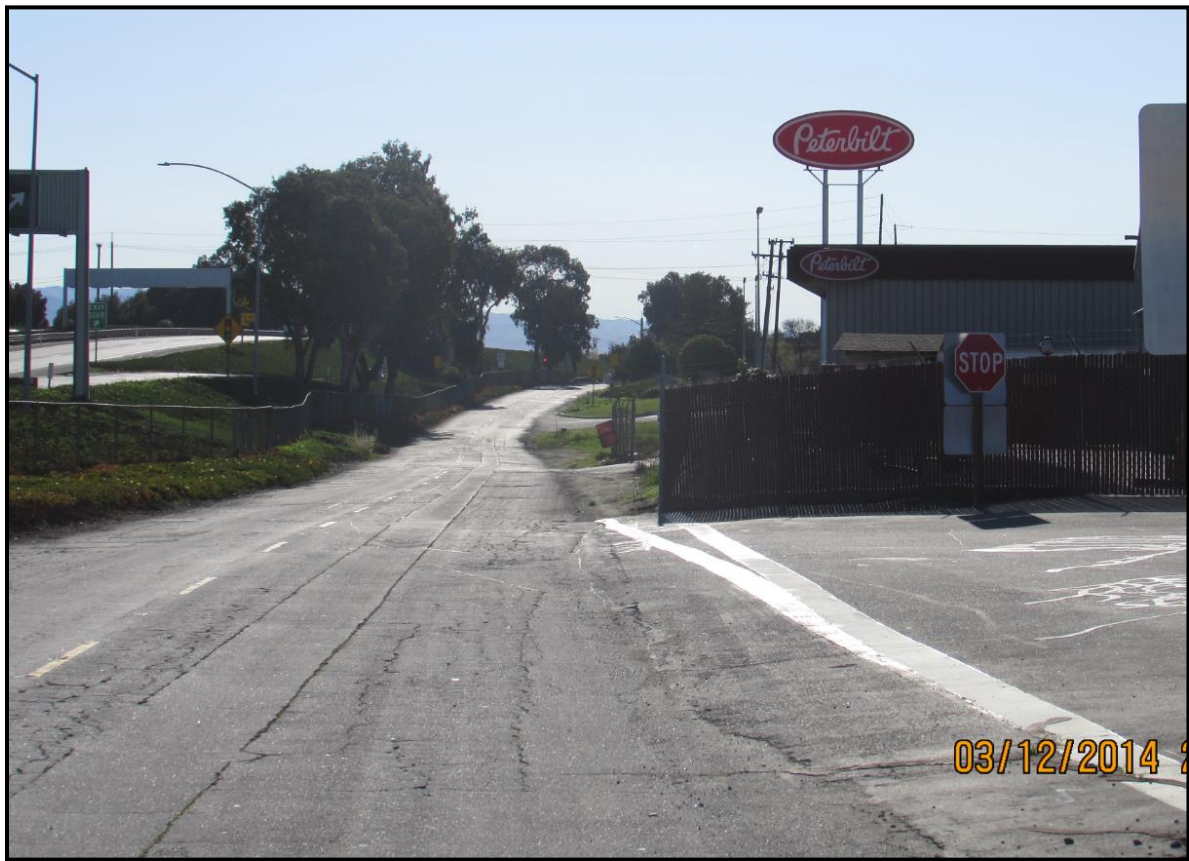
Elvee Drive Before Widening
