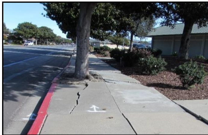
Before photo of San Felipe JOC Sidewalk Repair
