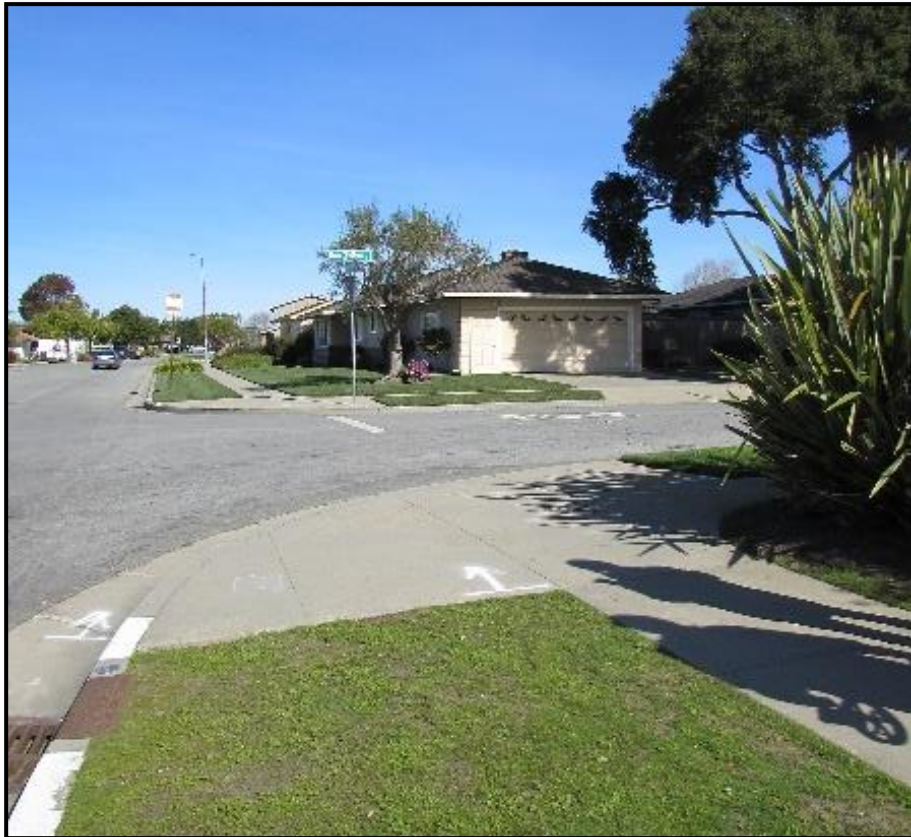
Before ADA Ped Ramp at Sierra Madre Dr and San Felipe St (southwest side)
