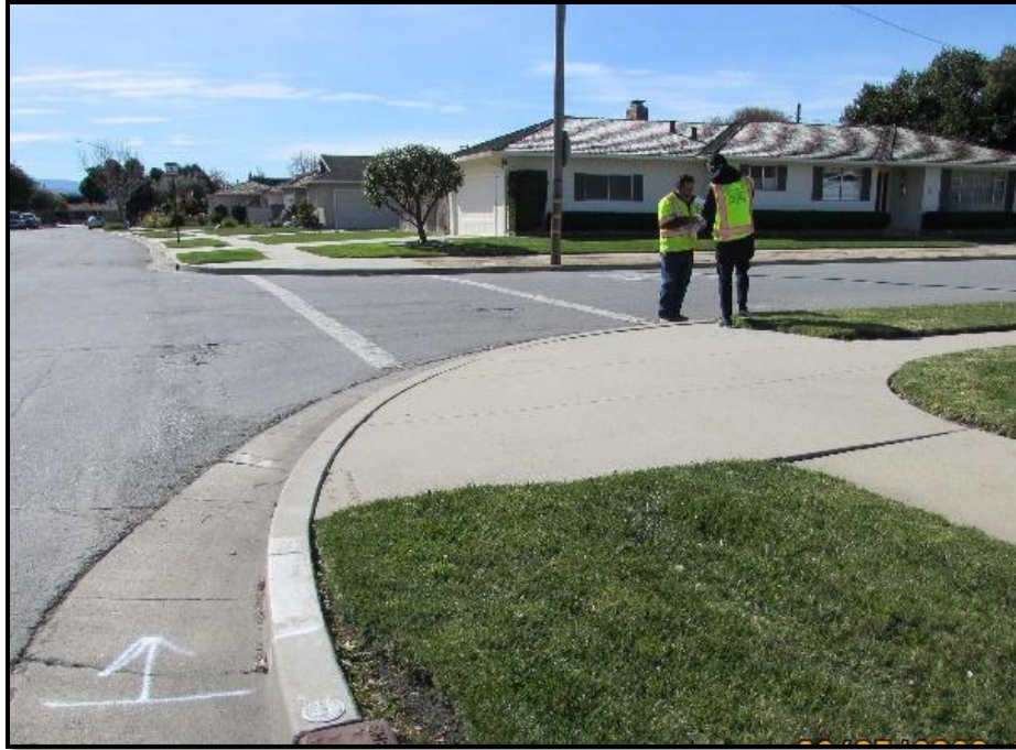
Before ADA Ped Ramp at Sierra Madre Dr and San Felipe St (northeast-northwest side)
