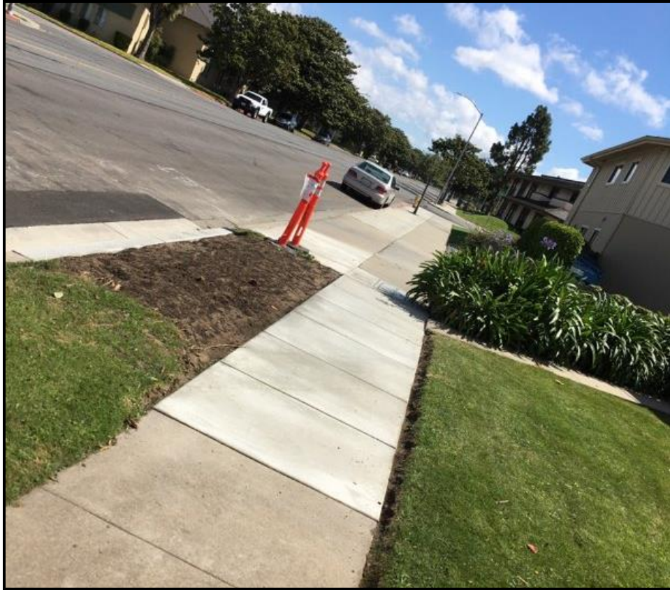
After photos of San Felipe JOC Sidewalk Repair
