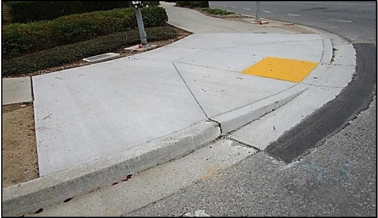
Before and after photo of ADA Pedestrian Ramp at N Sanborn Rd and Freedom Pkwy
