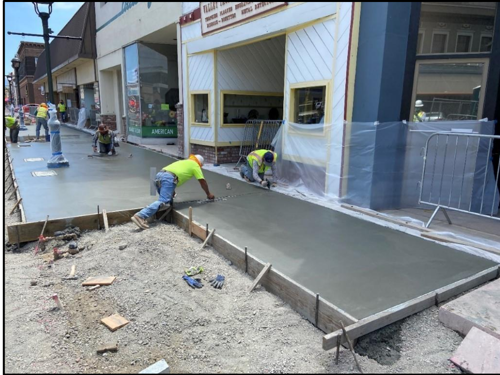
Construction Photo: New Sidewalks Fronting Businesses
