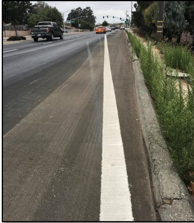
E Laurel Dr Westbound at Sanborn Rd. & at St Edwards Ave - No Sidewalk
