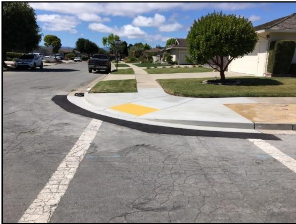
After ADA Ped Ramp at Sierra Madre Dr and San Felipe St (northwest side)
