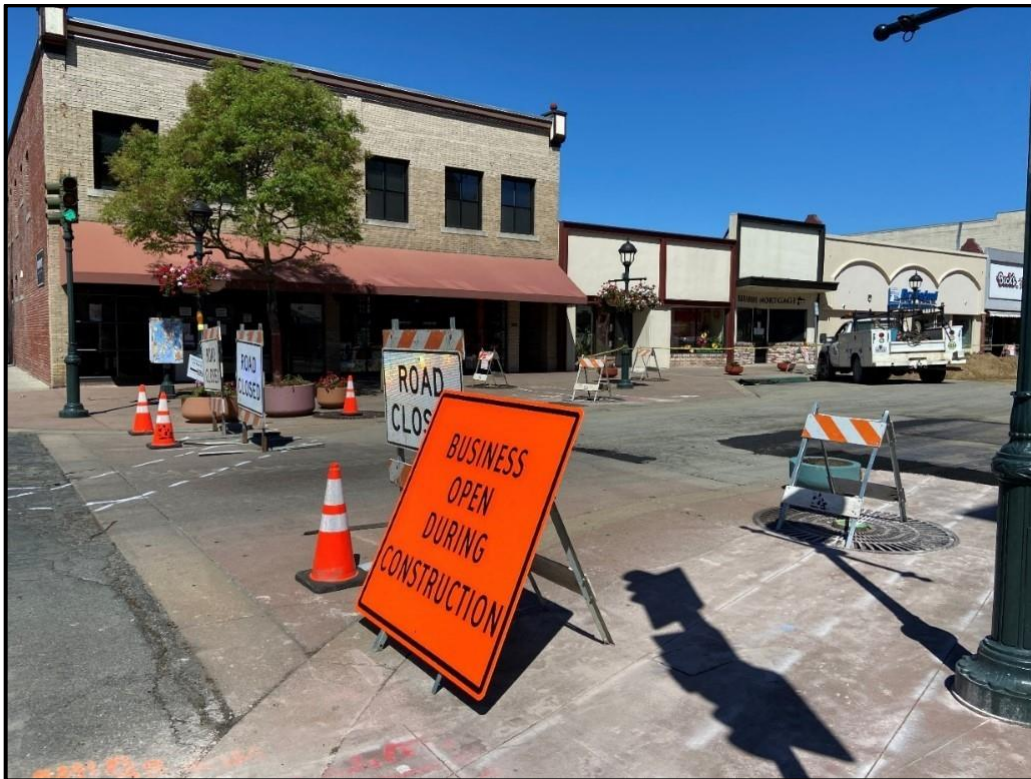
Construction Photo: Businesses Open During Construction
