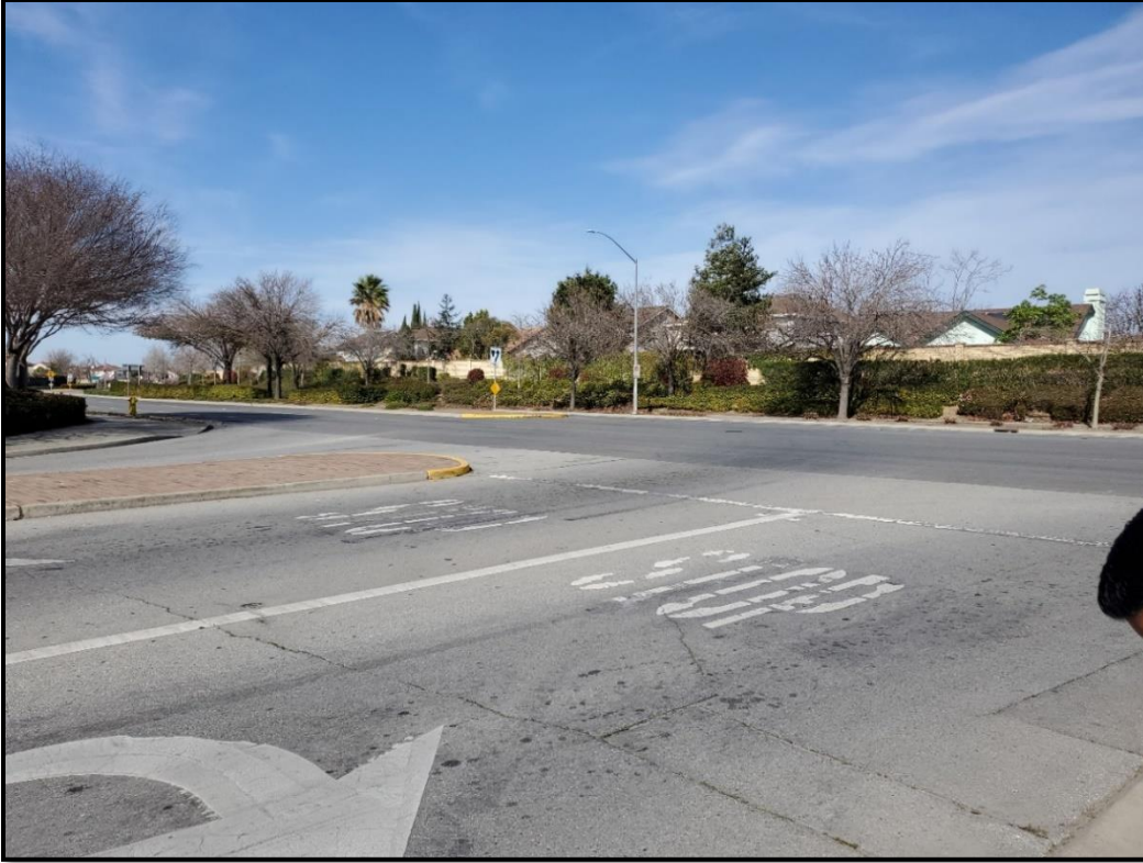
Before Photo: Las Casitas Drive at Constitution Boulevard facing Northbound (CIP 9227)
