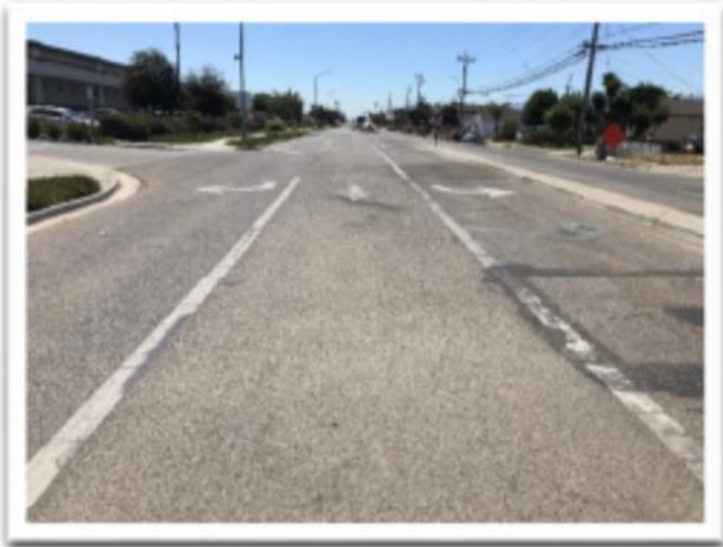
Bardin Road @ Williams Road North Bound facing South
