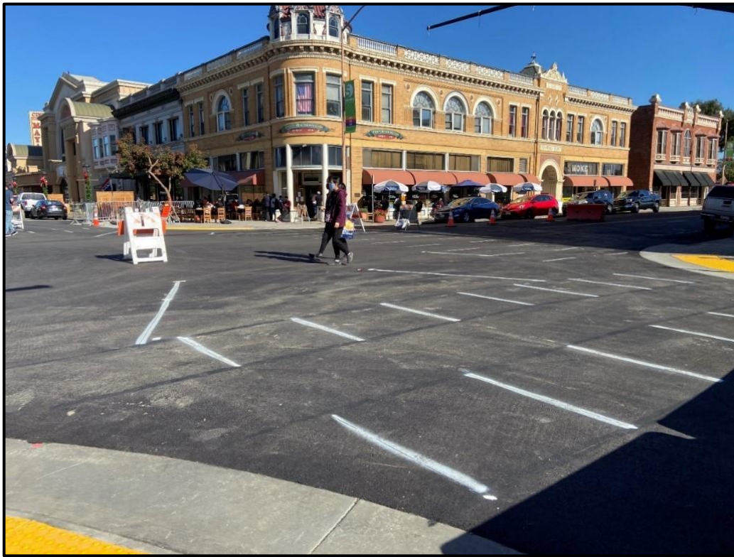
Construction Photo Preparing for Pedestrian Scramble Crosswalk
