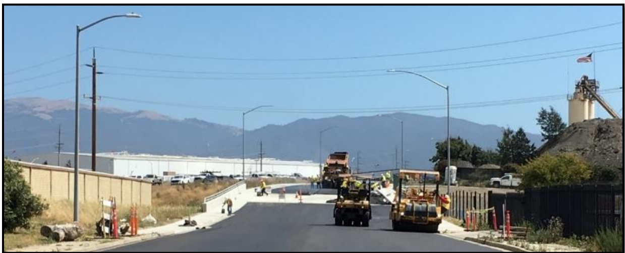
Elvee Drive near bridge construction
