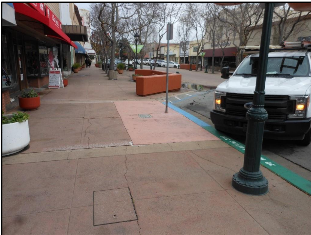
Before Photo: 300 Block Facing Southbound
