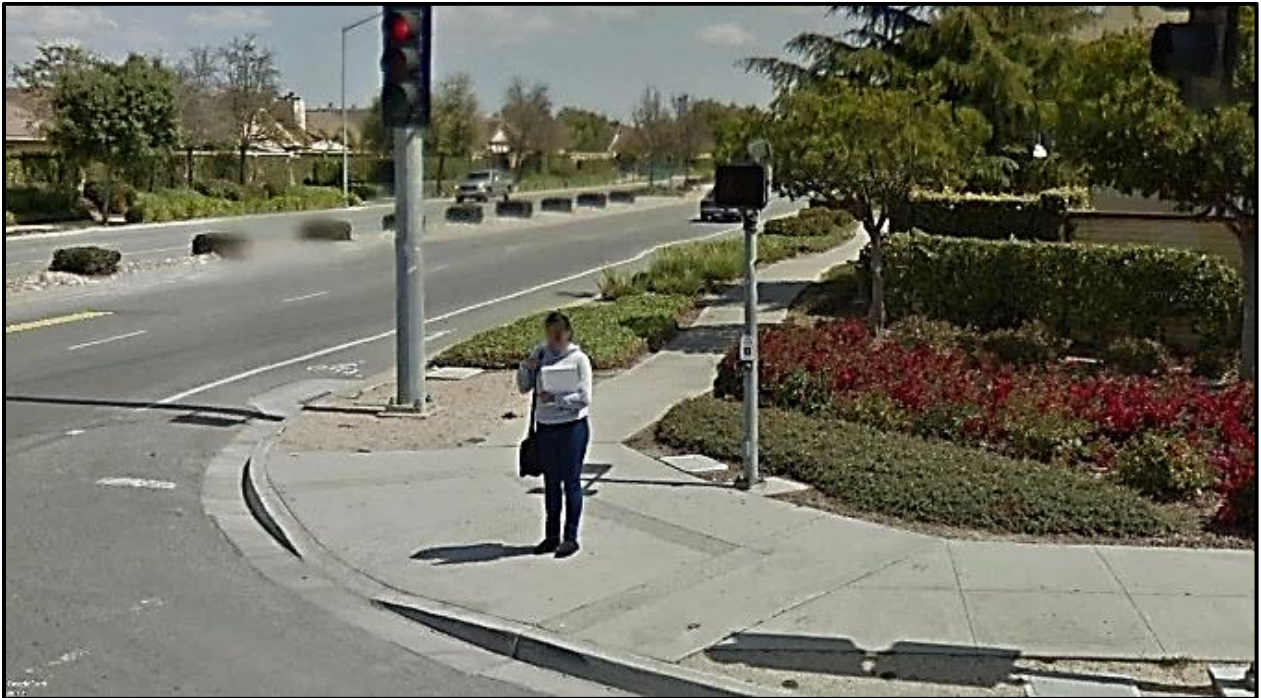
Before photo of ADA Pedestrian Ramp at N Sanborn Rd and Freedom Pkwy
