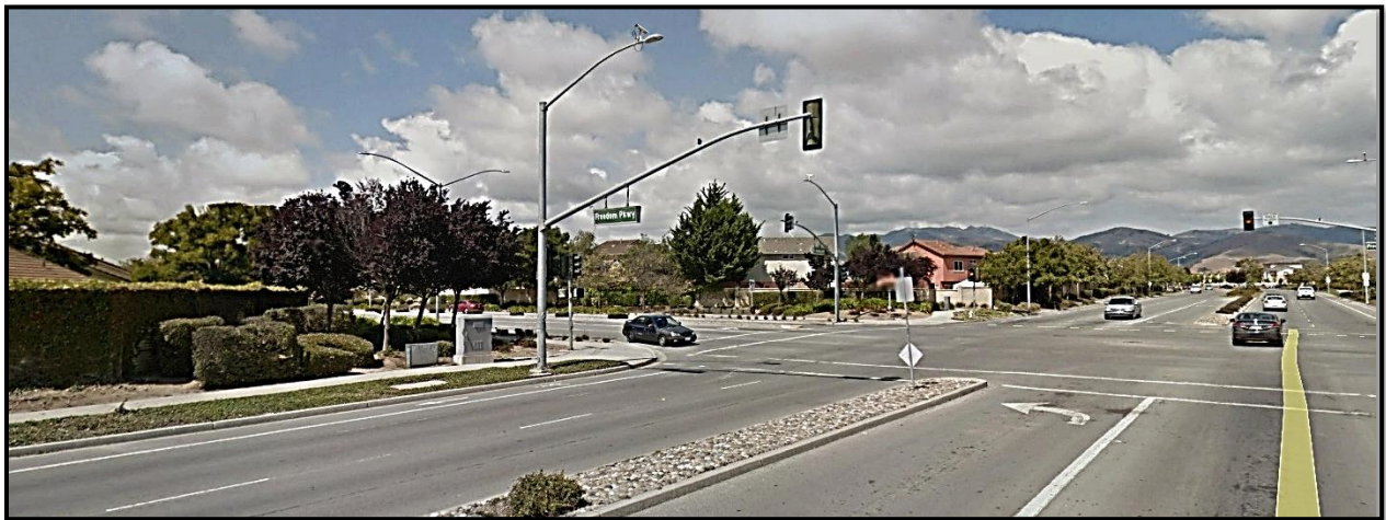
(Before) New Traffic Signal at N Sanborn Rd at Freedom Pkwy (Protected Left-Turn)
