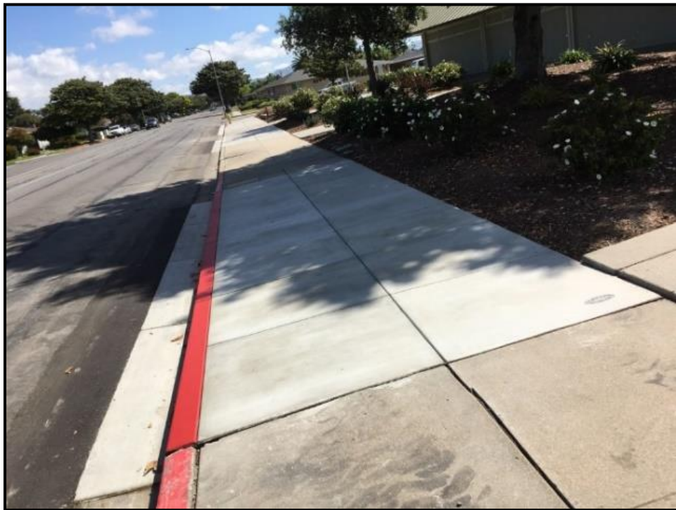
After photo of San Felipe JOC Sidewalk Repair
