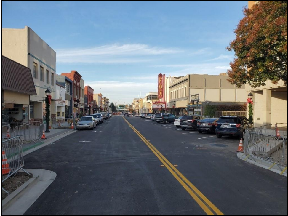
Construction Photo: 200 Block Opening up to 2-way traffic
