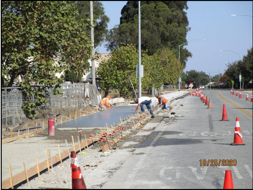
Construction Photo: New Sidewalk on Maryal Drive
