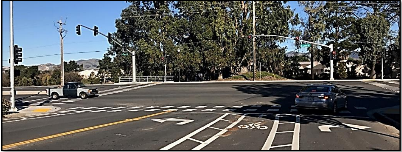
St. Edwards Dr. at E. Laurel Dr. after traffic signal installation.
