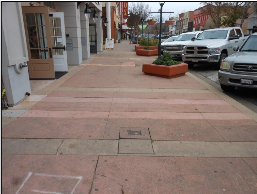
Before Photo: 200 Block Sidewalk Facing Southbound
