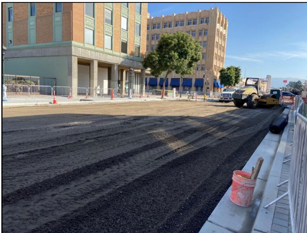
Construction Photo: Grading for a New Roadway Pavement
