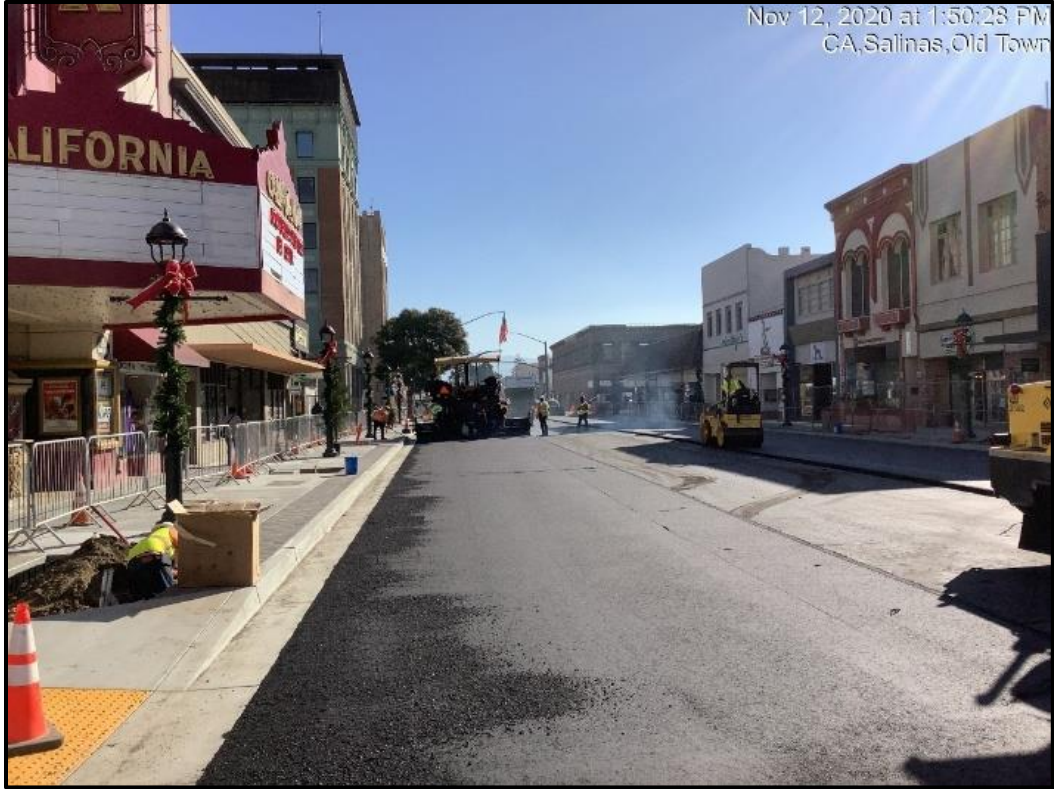
Construction Photo: 200 Block – Placing New Pavement
