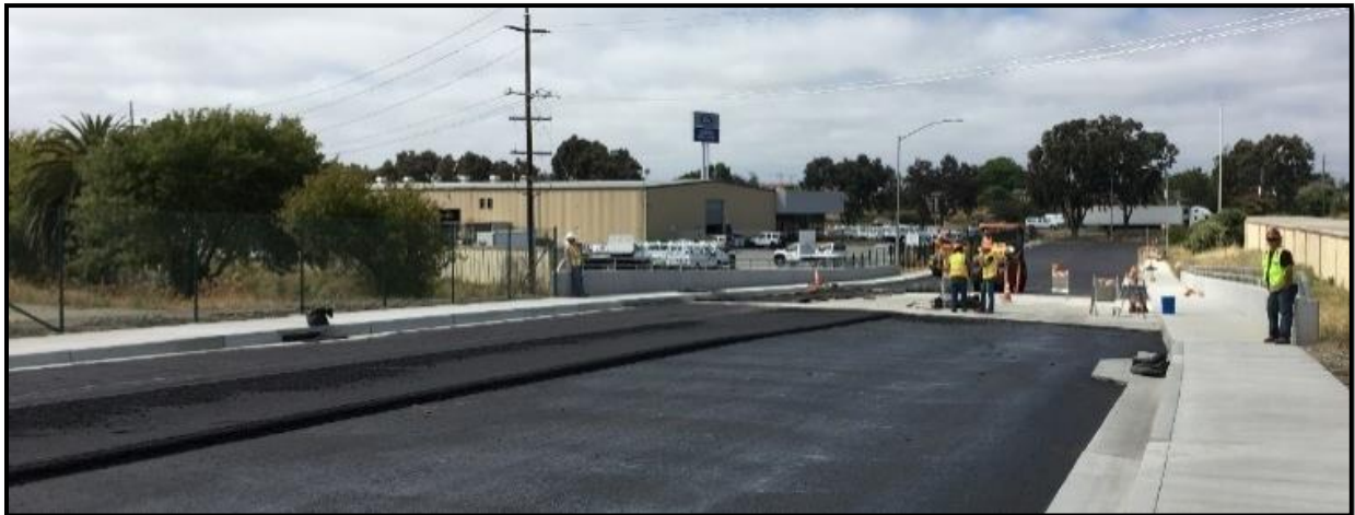
Elvee Drive near bridge construction
