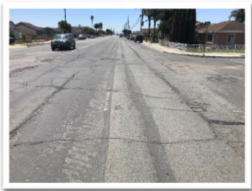
Bardin Road @ Afton Road South Bound facing South
