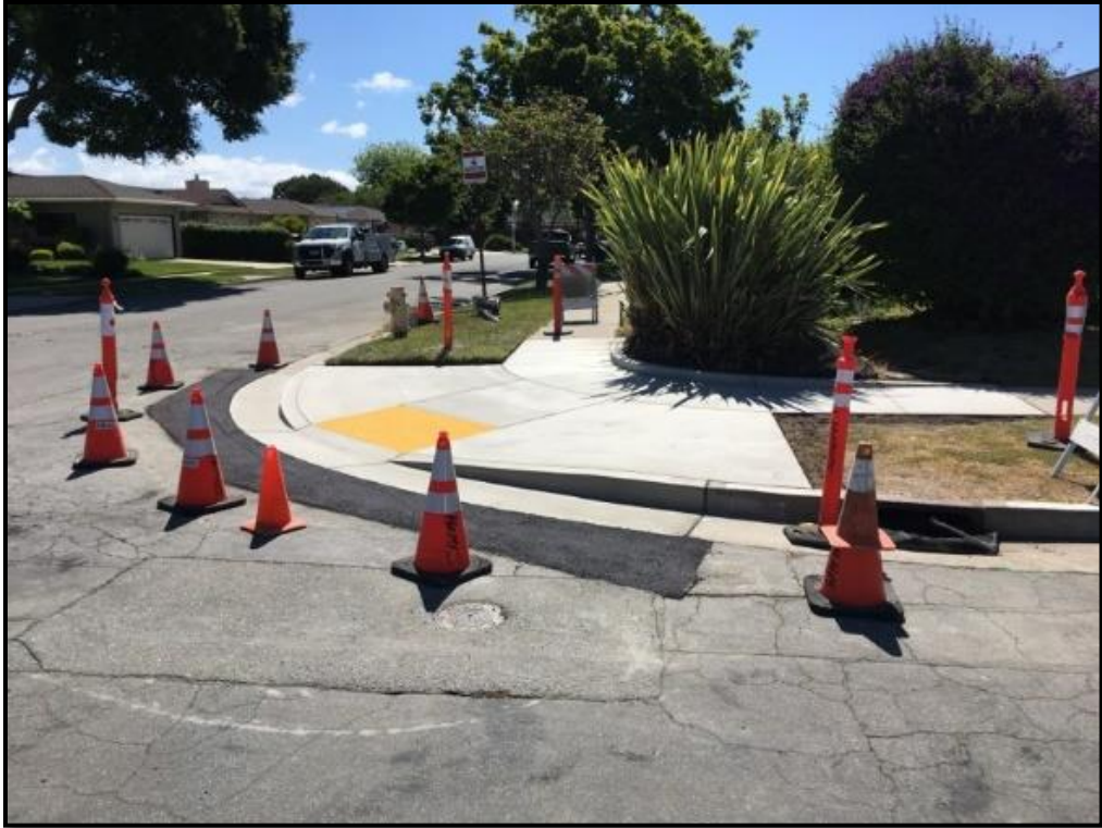
After ADA Ped Ramp at Sierra Madre Dr and San Felipe St (southwest side)
