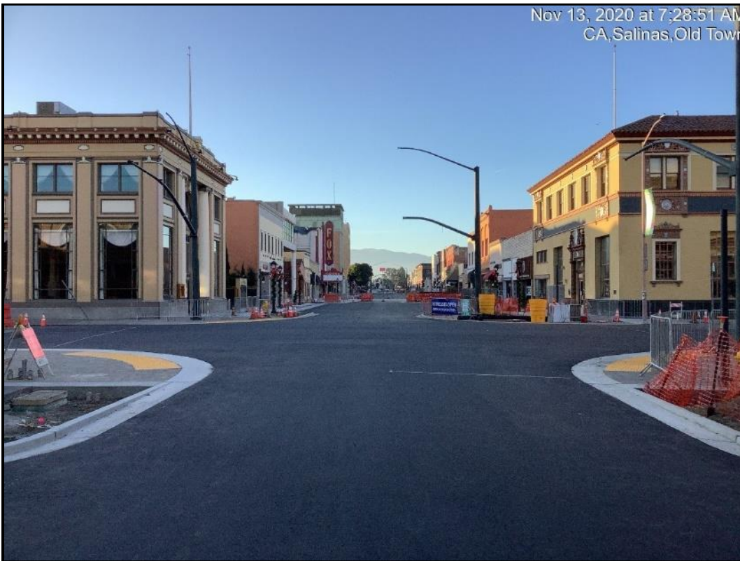
Construction Photo: Main St at Gabilan St – Completed Curb Returns and Paving
