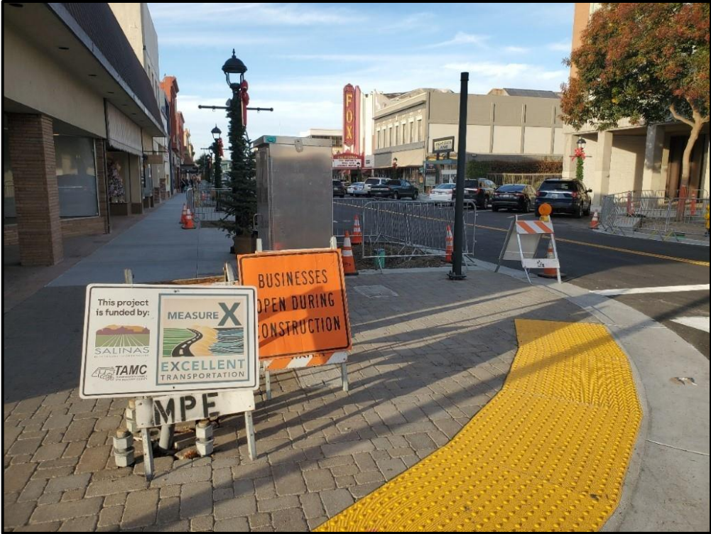
Construction Photo: Construction Signage and Holiday Preparations
