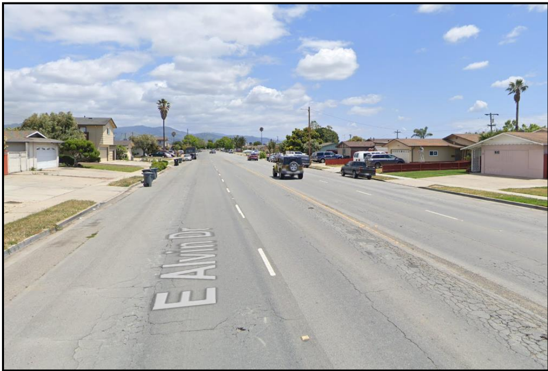
Before Photo at Alvin Drive (East of Linwood Drive)
