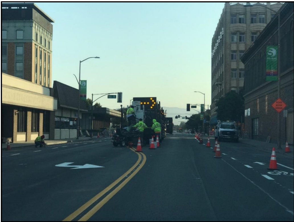
Construction Photo: Pavement Markings and Striping Installation
