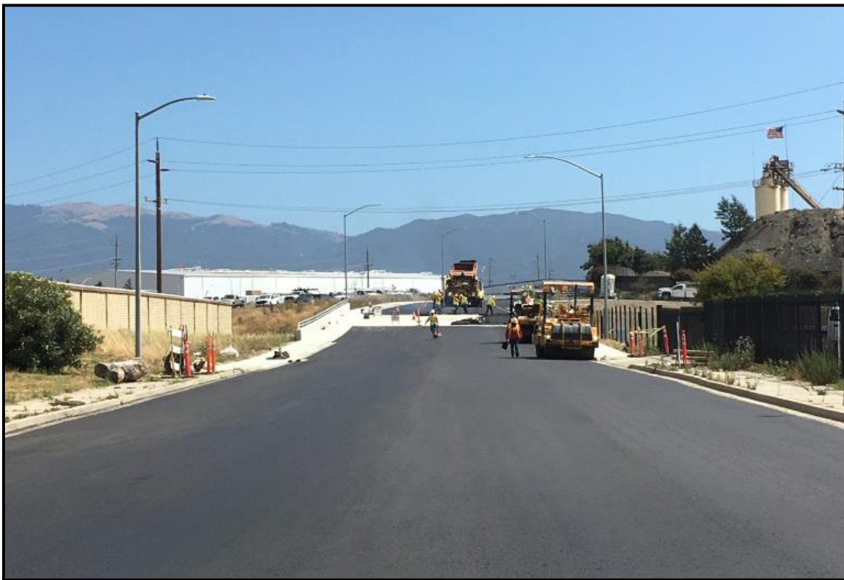
After Photo at Elvee Drive Extension and Bridge
