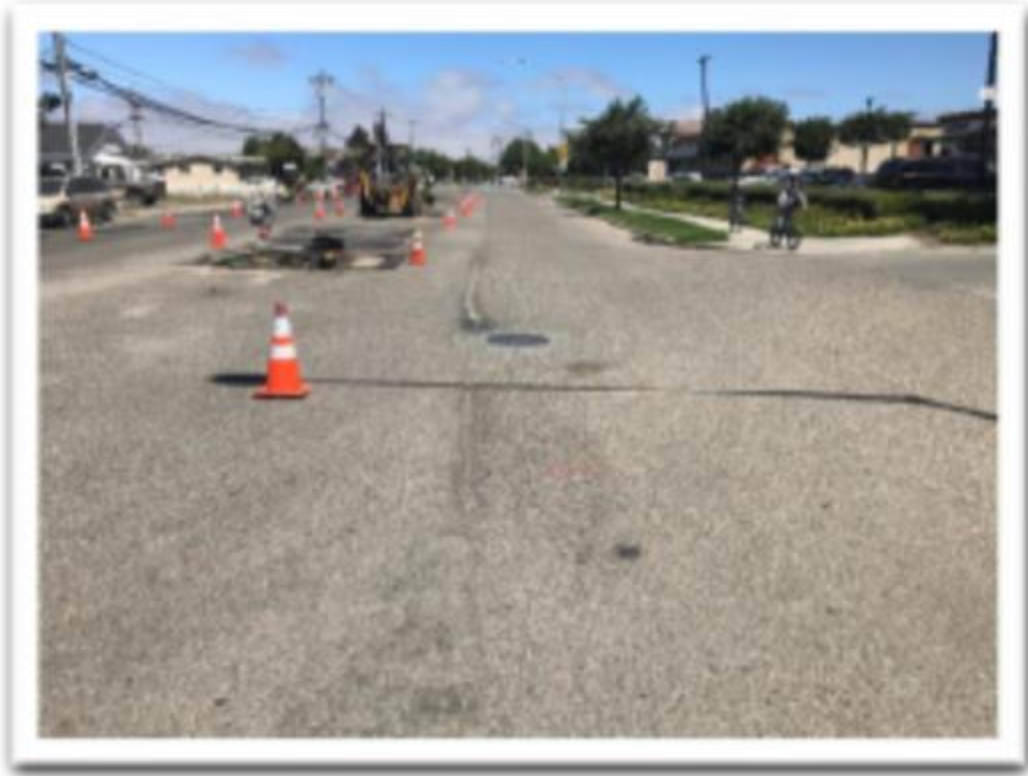
Bardin Road @ Toro Avenue North Bound facing North
