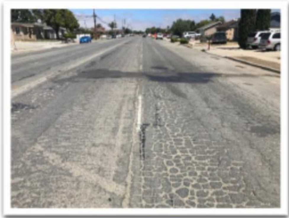
Bardin Road @ Afton Road North Bound facing North
