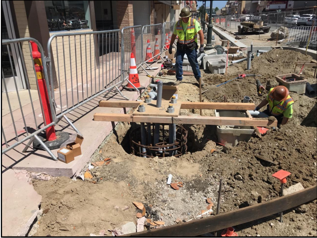
Construction Photo: New Signal Pole Foundation
