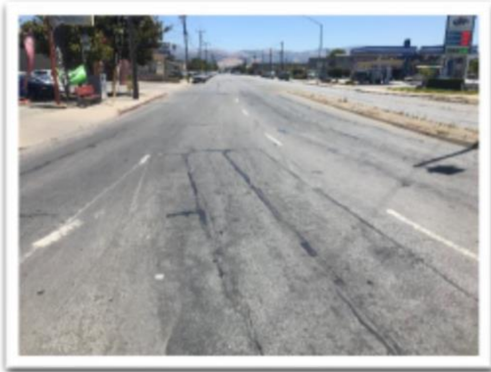
Williams Road @ E. Alisal Street West Bound facing East
