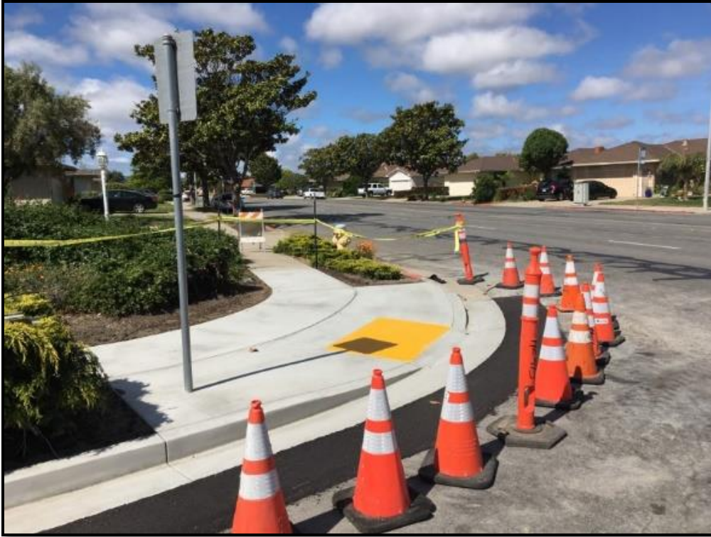
After ADA Ped Ramp at Walisal St and Ambrose Dr (southwest side)
