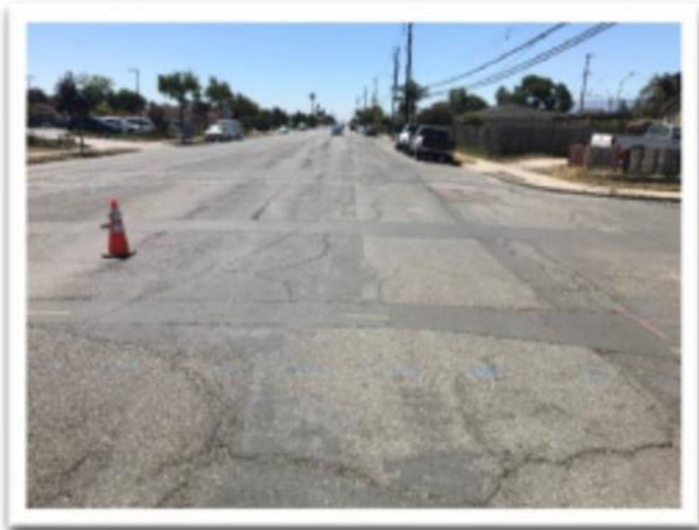
Bardin Road @ Toro Avenue South Bound facing South
