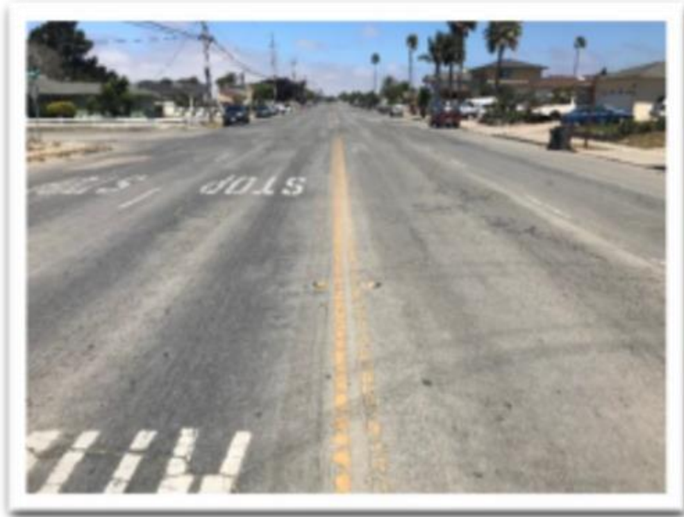
Bardin Road @ ~115' S/O Sycamore Road facing North
