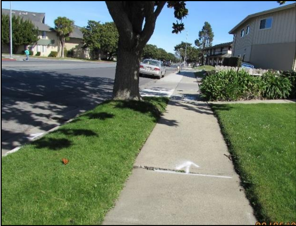
Before photo of San Felipe JOC Sidewalk Repair
