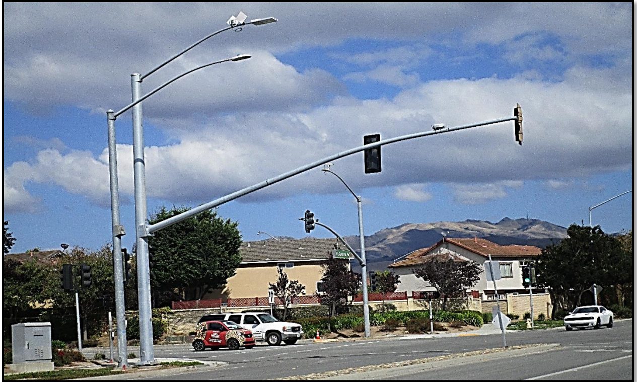
(After) New Traffic Signal with Protected Left-Turns at N Sanborn Rd and Freedom Pkwy
