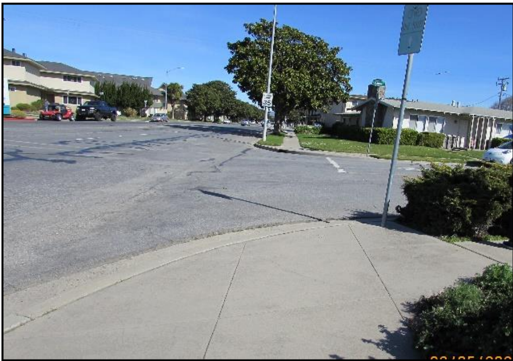
Before ADA Ped Ramp at Walisal St and Ambrose Dr (south side)
