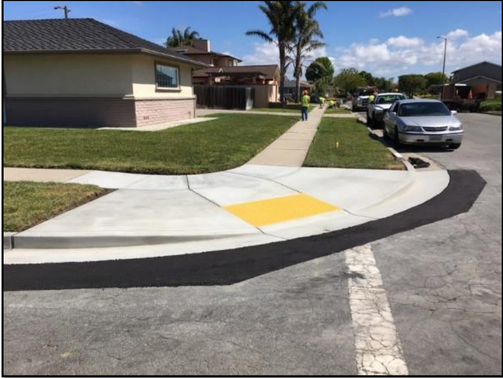
After ADA Ped Ramp at Sierra Madre Dr and San Felipe St (northeast side)
