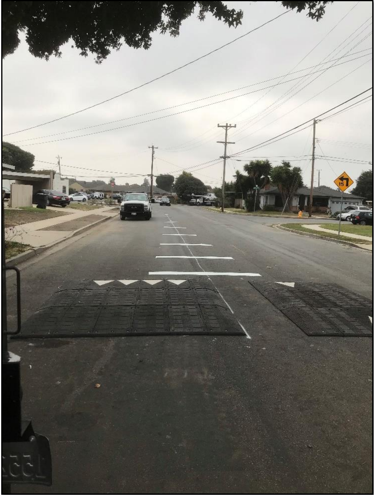
After Photo: Villa Street facing Southbound near Wilson Street
