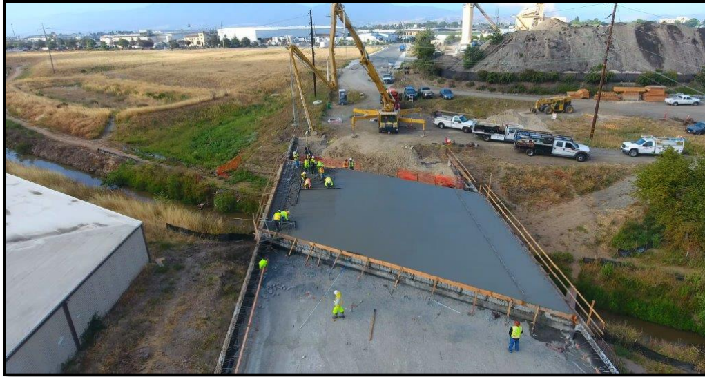
Construction of bridge at Elvee Drive
