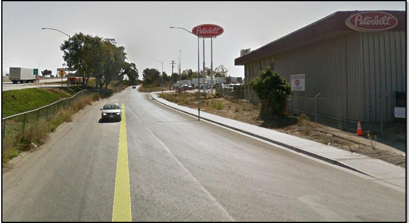
Elvee Drive After Widening
