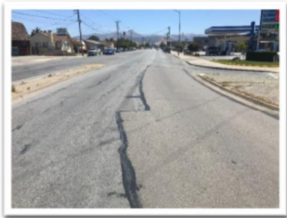
Williams Road @ E. Alisal Street East Bound facing East
