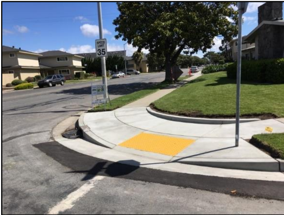
After ADA Ped Ramp at Walisal St and Ambrose Dr (southeast side)
