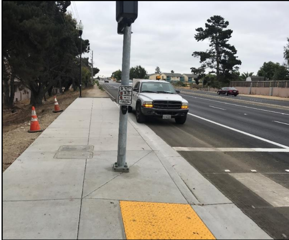
E Laurel Dr Westbound at Sanborn Rd. & at St Edwards Ave - No Sidewalk
