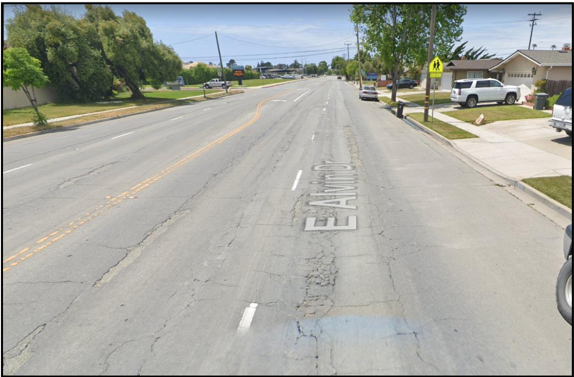
Before Photo at Alvin Drive (West of Linwood Drive)
