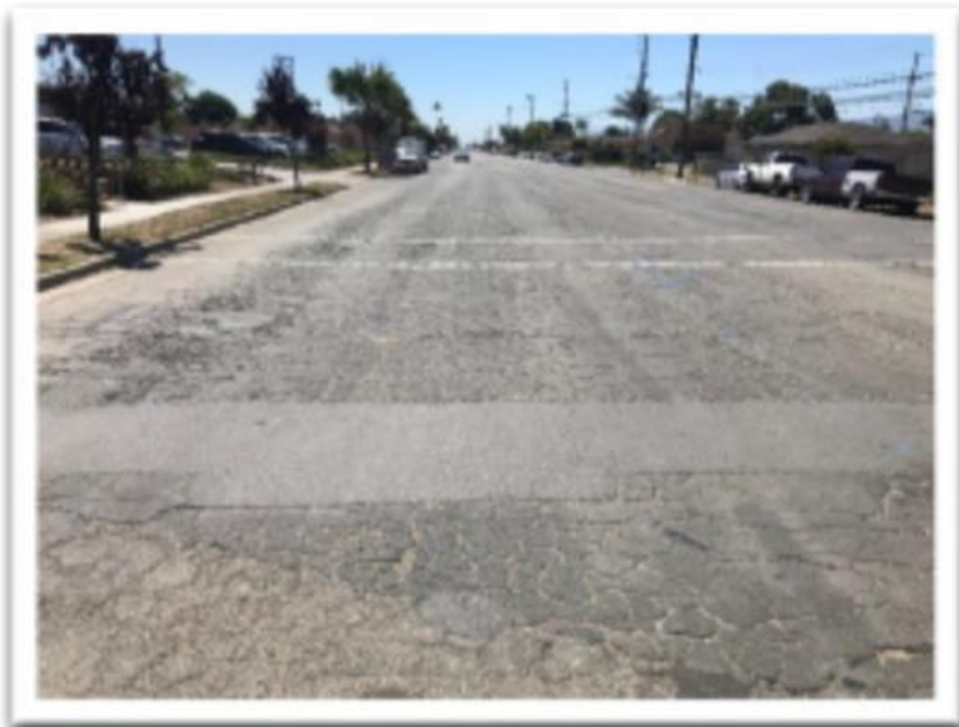
Bardin Road @ Toro Avenue North Bound facing South
