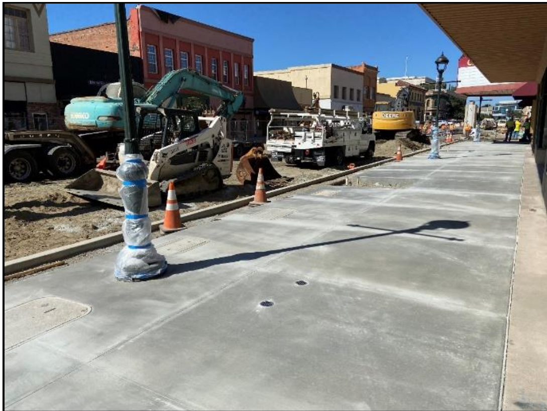
Construction Photo: New Sidewalk
