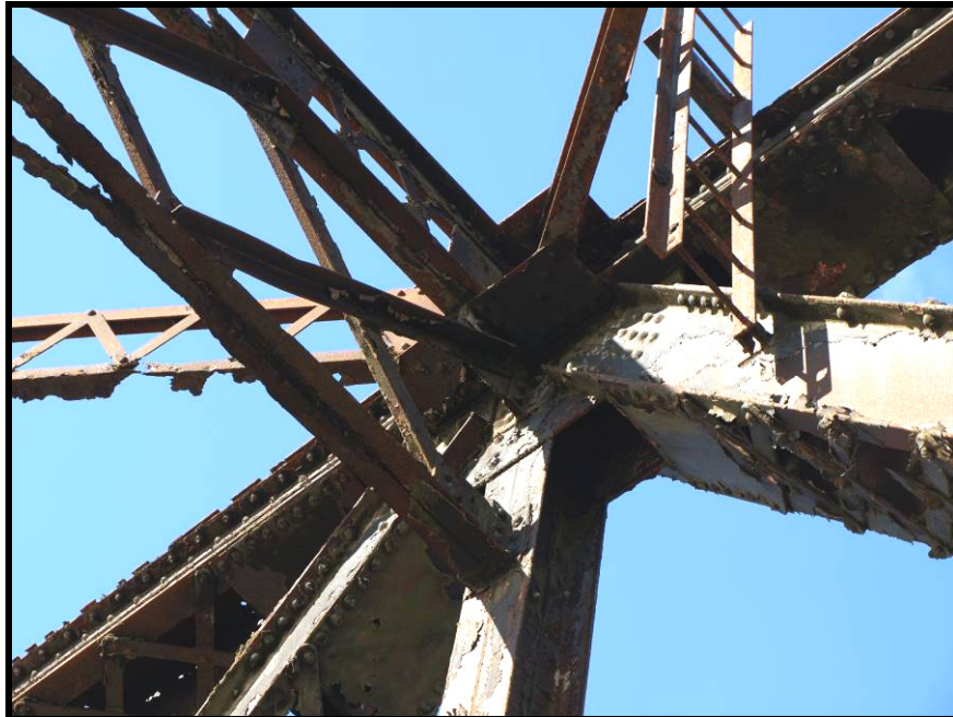
Photograph No. 13 – View shows section loss in top lateral brace & top sway brace at Panel Point L3L of Span 4.
