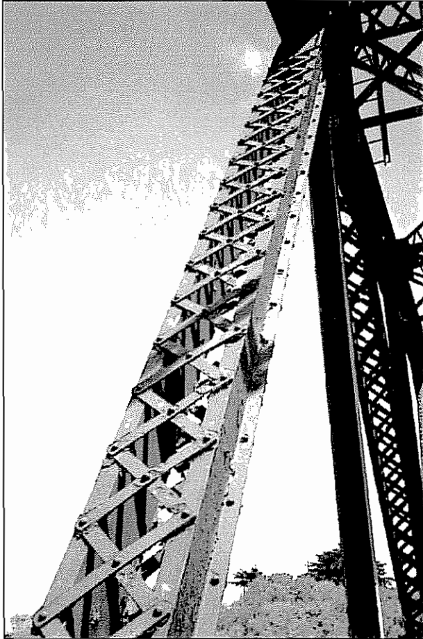
Photograph No. 4 (left) – View shows Diagonal U3-L4 of the right truss of Span 5. Note that there is very little paint remaining on the diagonal.
