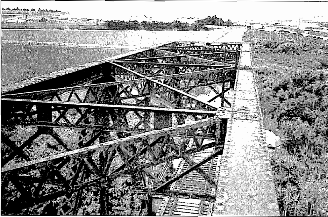
Photograph No. 6 – View shows the top chord and upper truss bracing of Span 5. Note that there is very little paint remaining on the visible surfaces.
