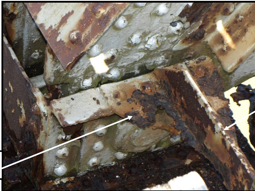
Photograph No. 18 – View shows corrosion and section loss in stringer strut & strut gusset plate at Panel Point L6R of Span 4
