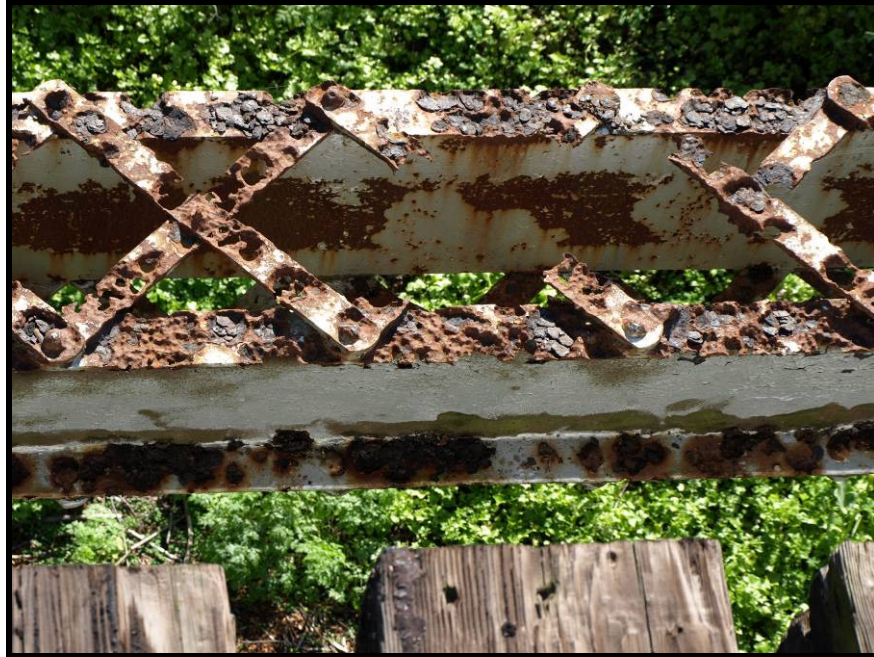
Photograph No. 5 – View shows corrosion and section loss of flanges of bottom chord in Panel 4 of Span 1, right side.
