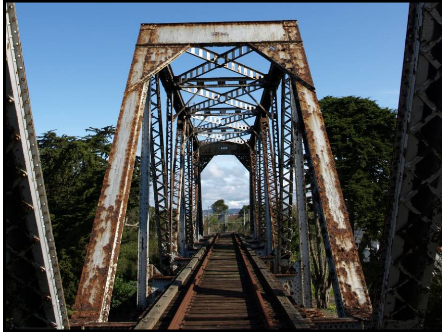
Photograph No. 3 –View of paint loss on various truss members of Span 1 looking North.
