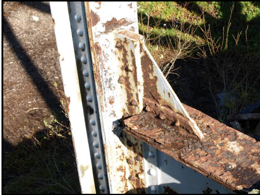
Photograph No. 17 – View shows the right floorbeam bracket of Floorbeam 5 of Span 1
