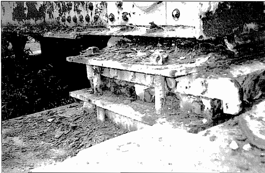
Photograph No. 12 – View of the truss expansion bearing of Span 1, right side. Note that the segmental roller at the right side of the photo is no longer under the upper bearing plate.
