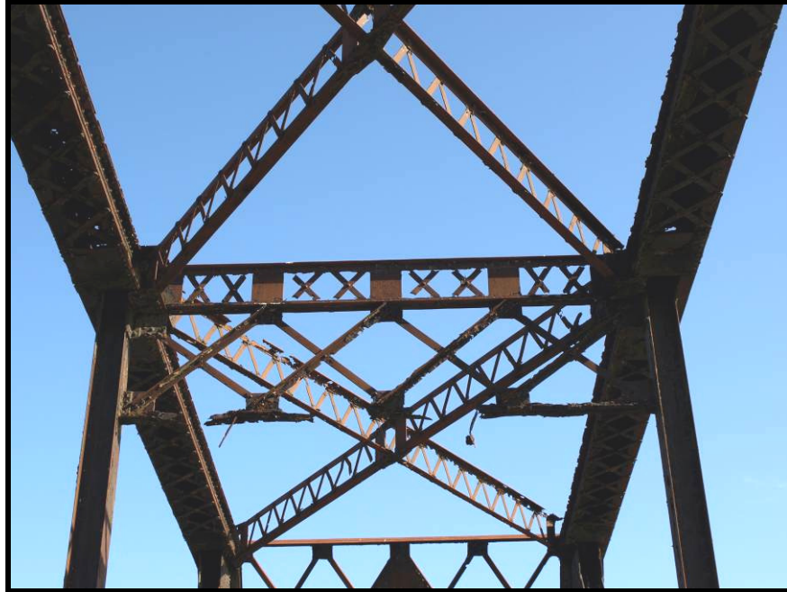
Photograph No. 12 – View shows section loss in top sway and strut brace at Panel Point L2L of Span 5.
