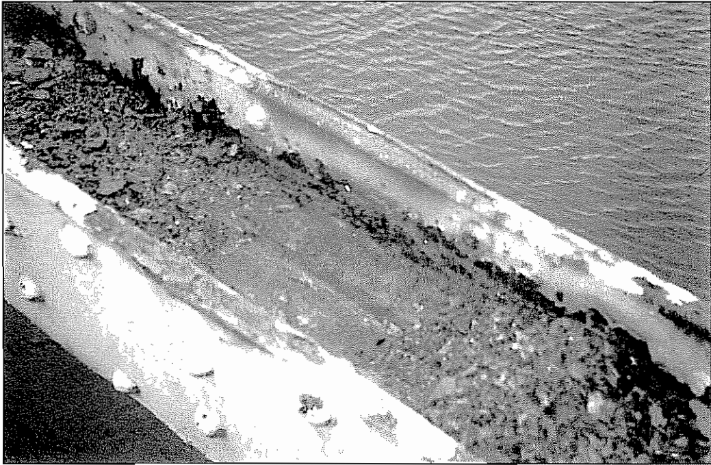
Photograph No. 8 – View shows corrosion and minor section loss at the web plate and Outboard flange of the bottom chord in Panel 4 of Span 4, right side. Also note minor section loss and spreading at the flanges due to crevice corrosion.
