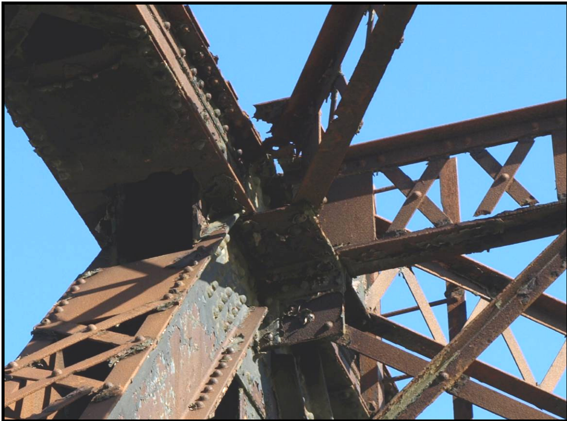
Photograph No. 11 – View shows section loss in top lateral brace connection plate at Panel Point L3L of Span 5.
