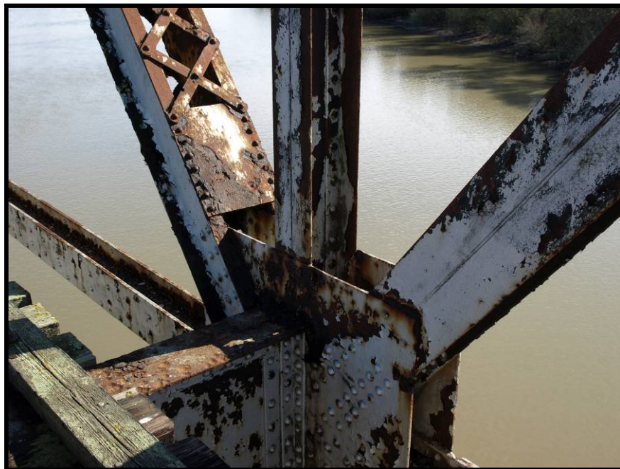
Photograph No. 2 – View of paint loss at Panel Point L4L of Span 5.
