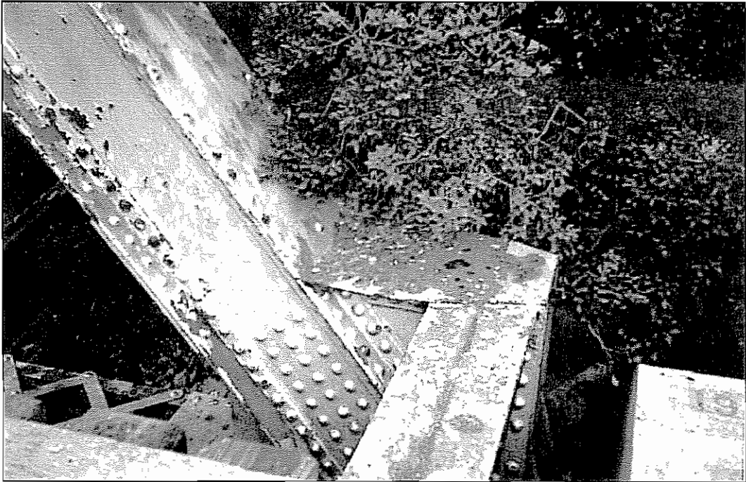
Photograph No. 19 – View of the end post-to-floorbeam connection plate of Span 1 at L0, right side. Note the holes in the plate, which has 70% section loss overall.
