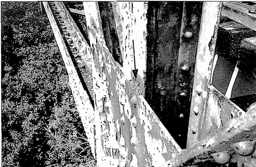
Photograph No. 9 – View shows an isolated area of section loss in the outboard flange of the post at Panel Point L4L of Span 2 (arrow).
