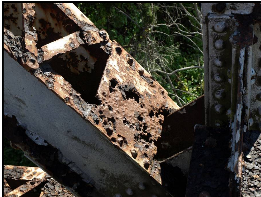
Photograph No. 6 – View shows corrosion and section loss on flanges of diagonal U1-L2 in Panel 2 of Span 1, right side.
