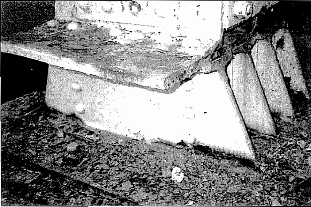
Photograph No. 14 – View of the truss fixed bearing of Span 3, left side. Note corrosion and section loss along the bottom of the webs of the bearing pedestal I-beams.
