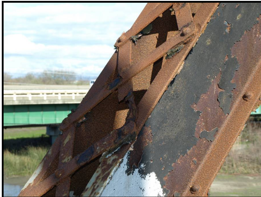
Photograph No. 4 – View of paint deterioration of Diagonal U3-L4 of the right truss of Span 4.
