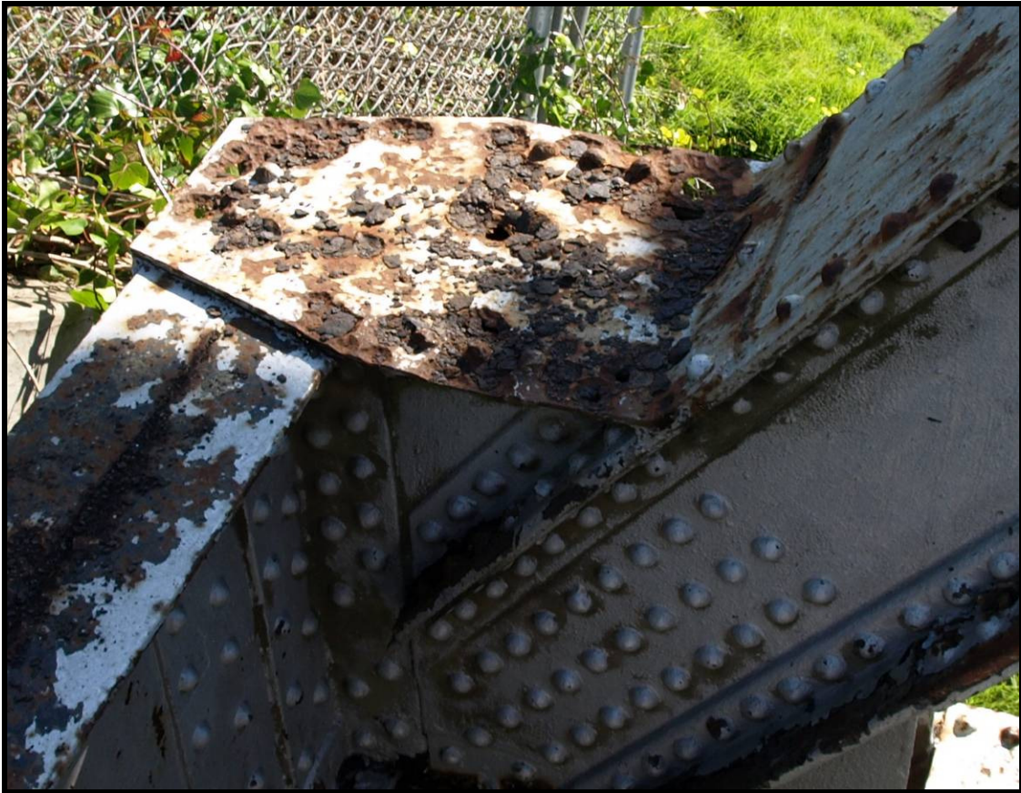
Photograph No. 16 – View of the end post-to-floorbeam connection plate of span 1 at LOL.
