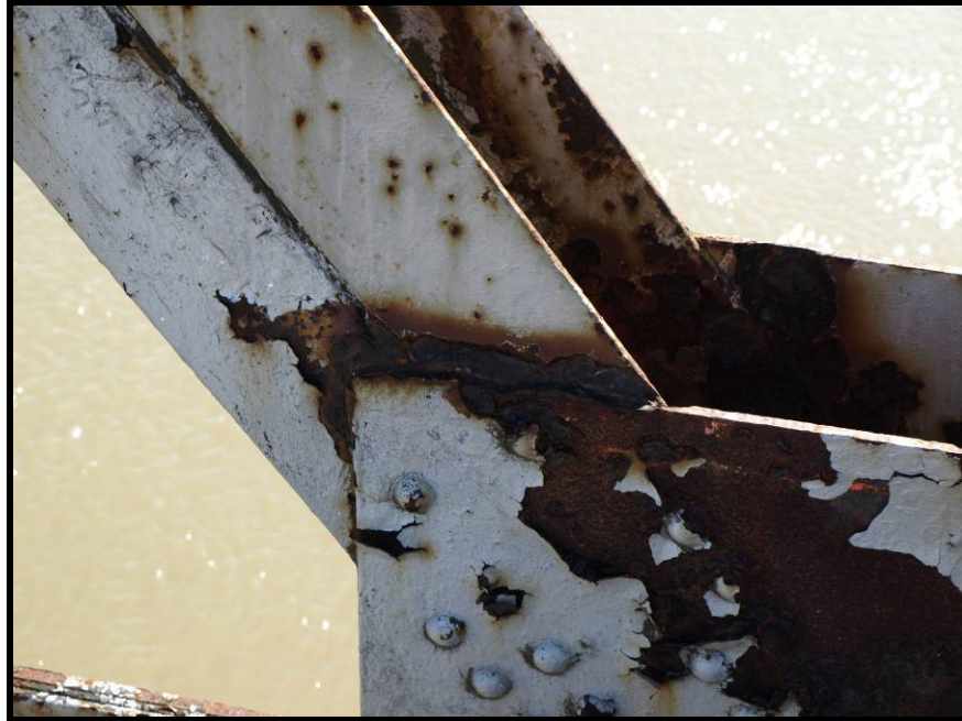
Photograph No. 9 – View shows corrosion and section loss of inboard flanges of diagonal L4-U5 of the left truss of Span 4.
