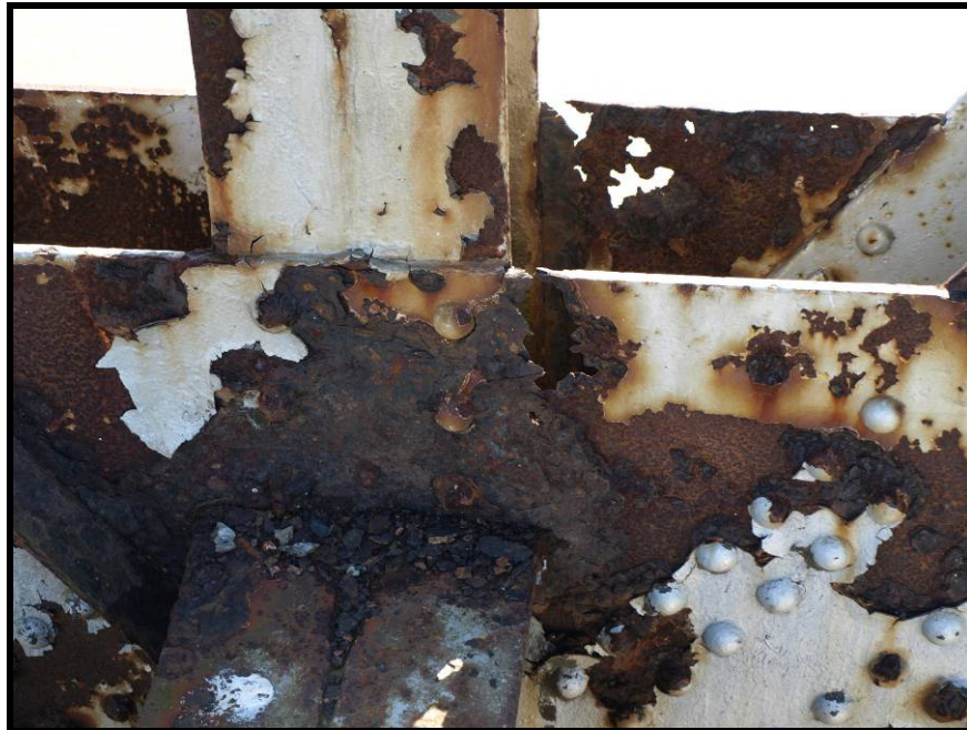
Photograph No. 10 – View shows corrosion and section loss of inboard and outboard gusset plates at Span 4, Panel Point L2L.
