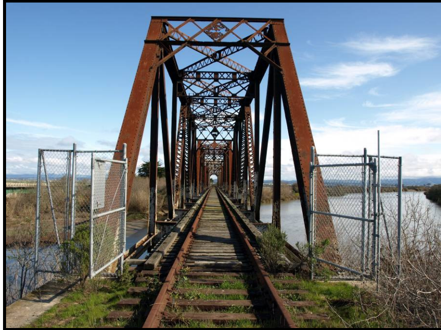
Photograph No. 1 – View of paint loss on various members beginning at Span 5 and looking North.
