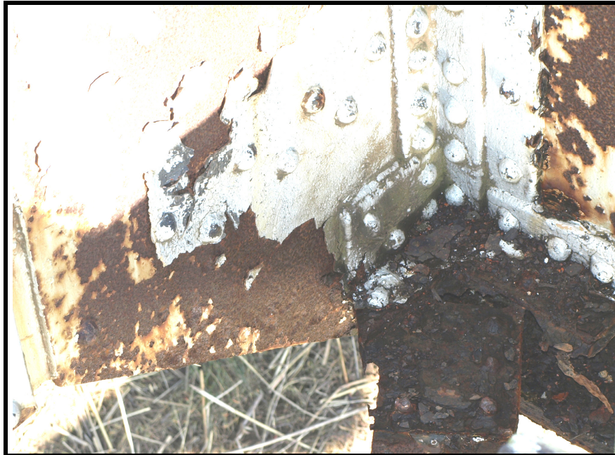
Photograph No. 15 – View shows section loss in bottom lateral brace gusset plate at Panel Point L4R of Span 3.
