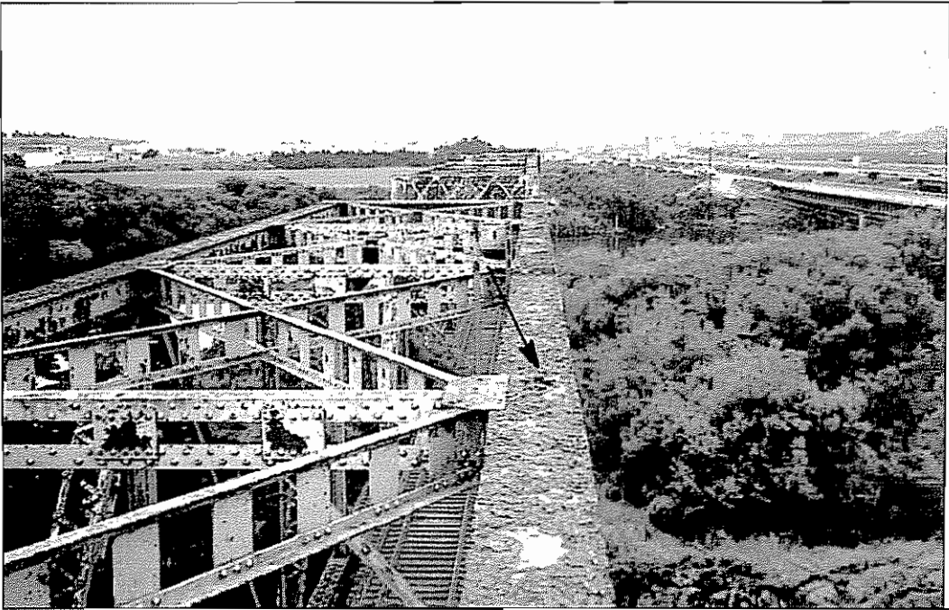
Photograph No. 7 – View of the top chord of Span 1 from Panel Point U1R. Note extensive corrosion and section loss of the cover plate, including holes at U2R (arrow).
