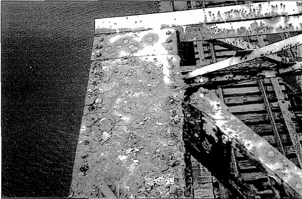
Photograph No. 10 – View shows 100% section loss of the upper connection plate of the top lateral, at Panel Point U5L of Span 3.
