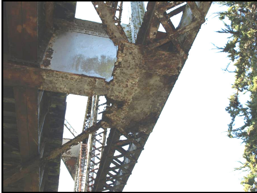
Photograph No. 14 – View shows section loss in bottom lateral brace & gusset plate at Panel Point L3L of Span 1.
