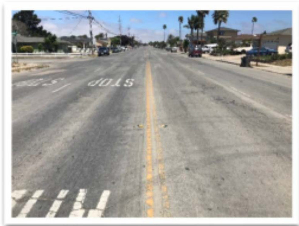
Bardin Road @ ~115' S/O Sycamore Road facing North
