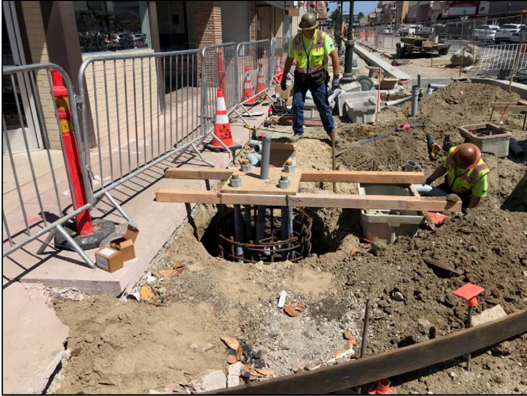
Construction Photo: New Signal Pole Foundation
