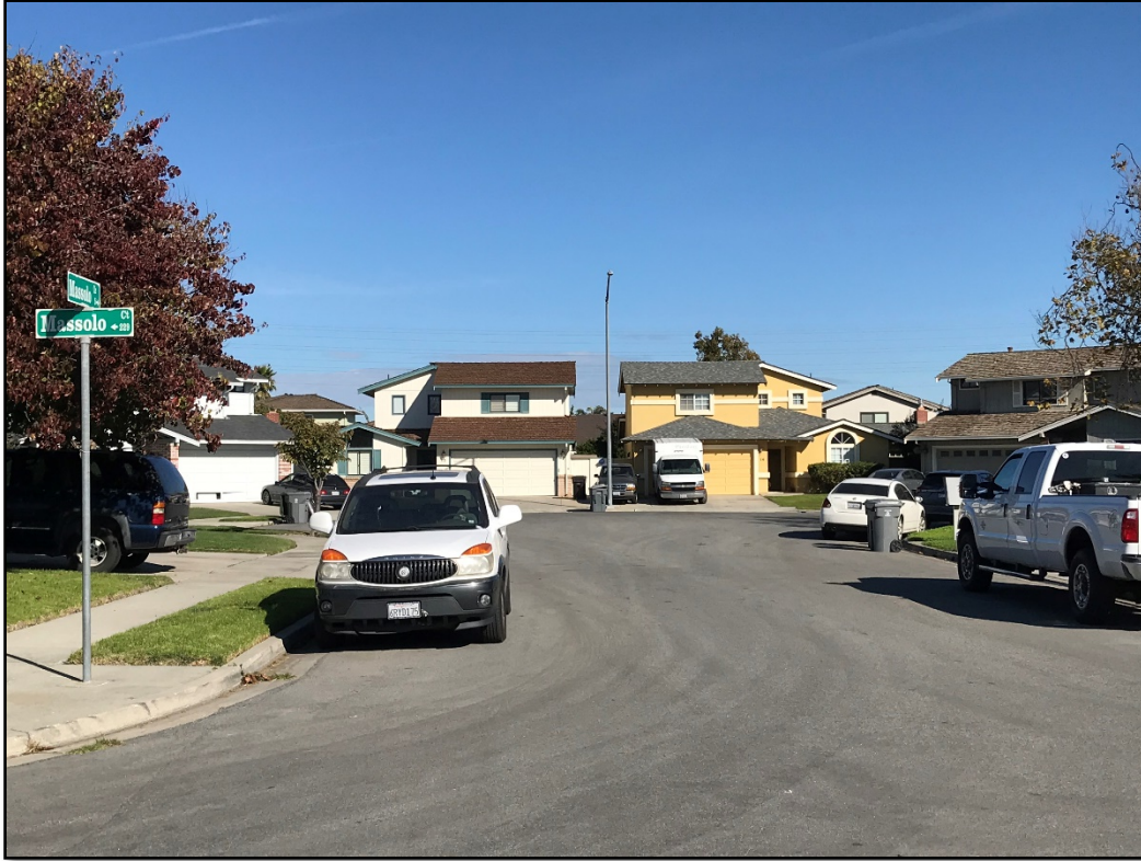
Before photo at Massolo Circle
