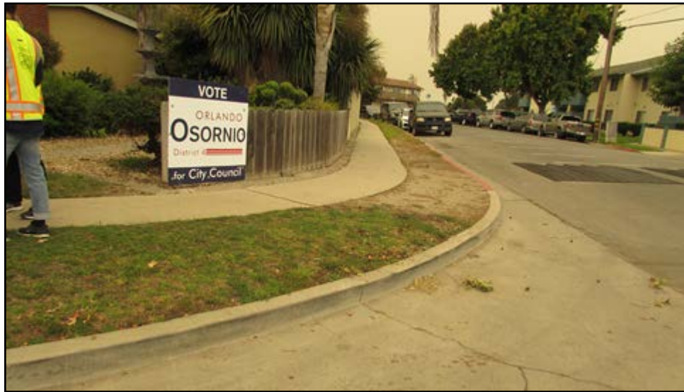
Before ADA Ped Ramp at 1296 Hilltop Dr
