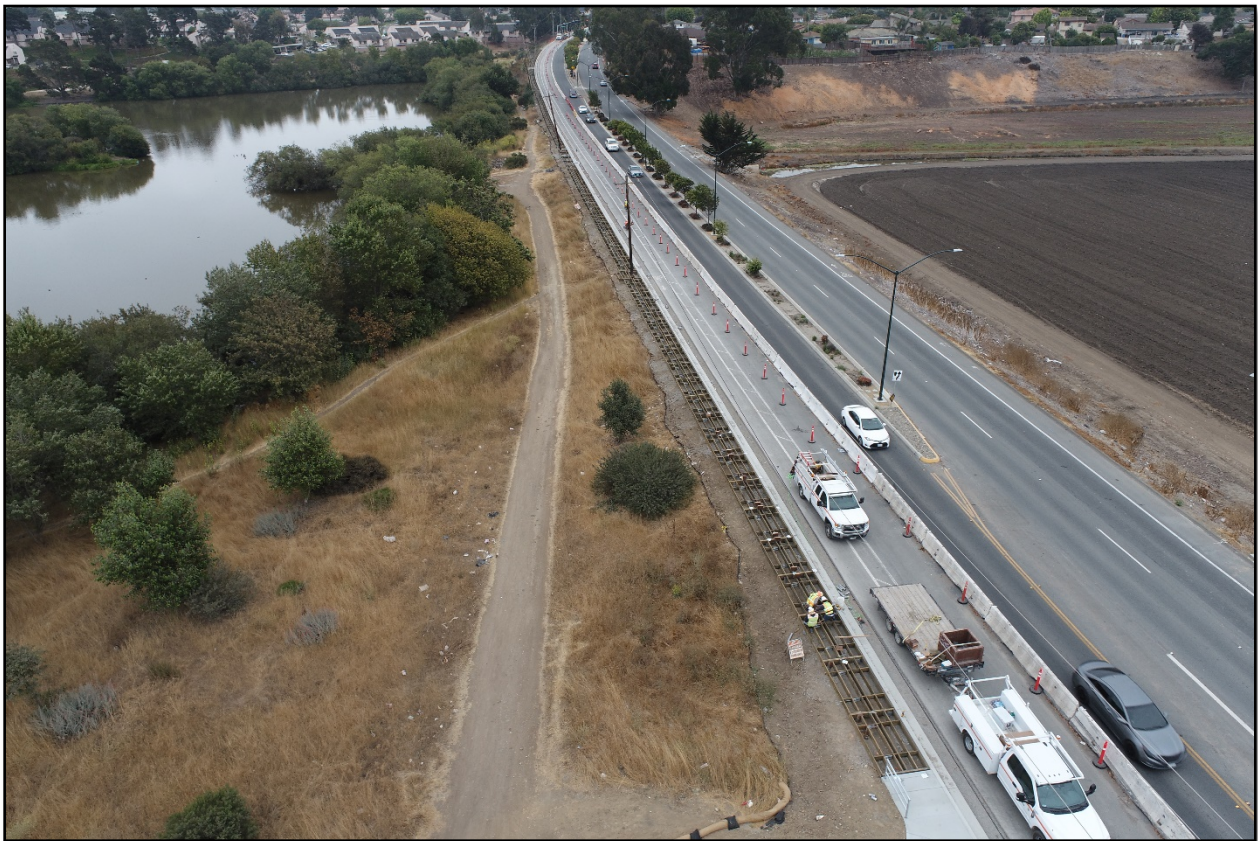
Laurel Boardwalk construction
