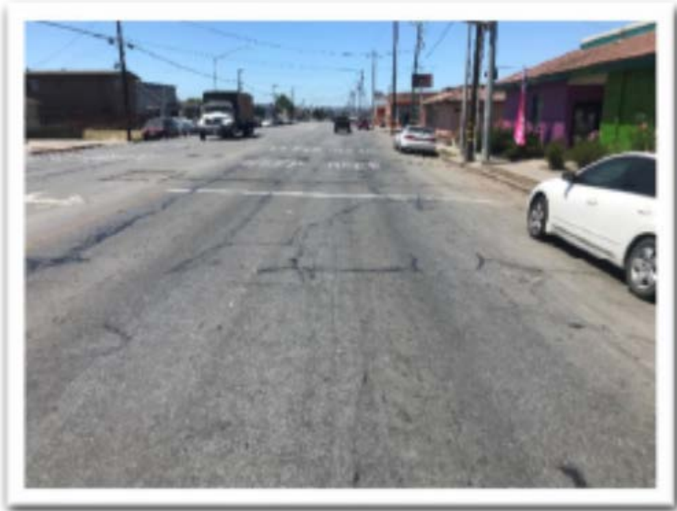
Williams Road @ Grandhaven Street West Bound facing West
