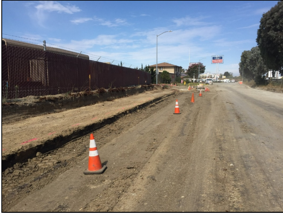
Photo of Elvee Drive near Sanborn Road During Construction
