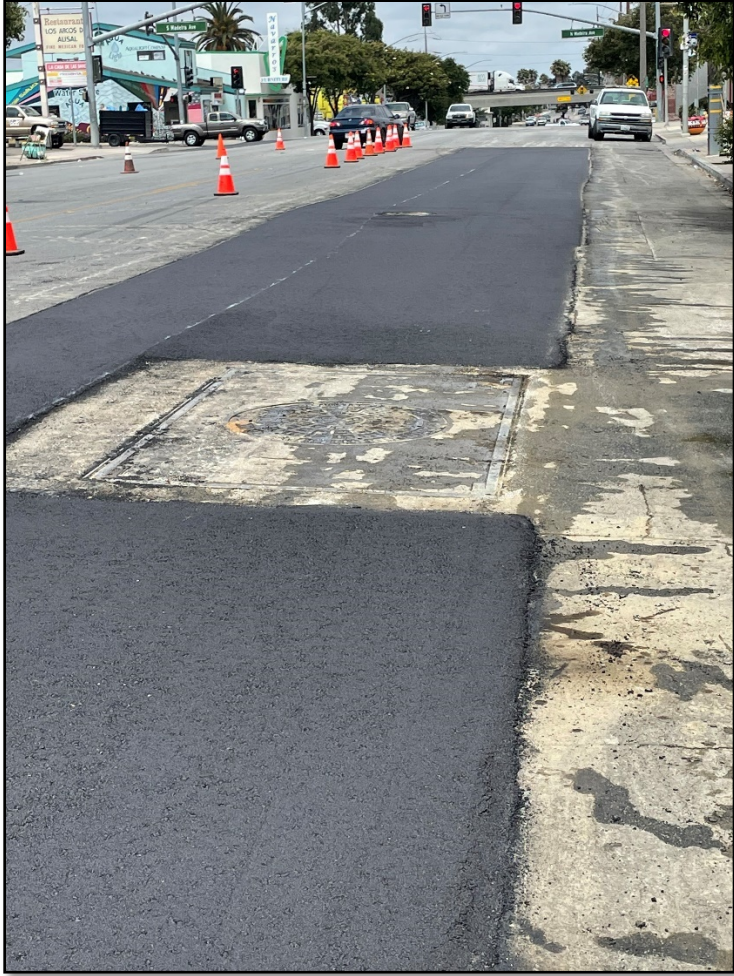
Pavement maintenance at E Alisal St and N Madeira Ave
