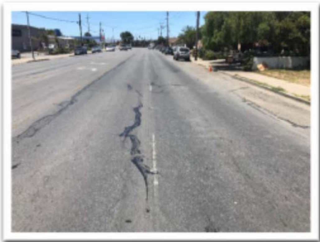
Williams Road @ Quilla Street West Bound facing West
