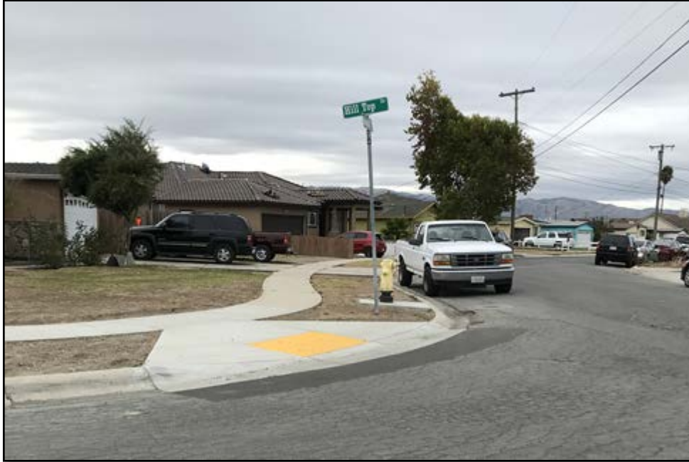
After ADA Ped Ramp at 1279 Summit Dr
