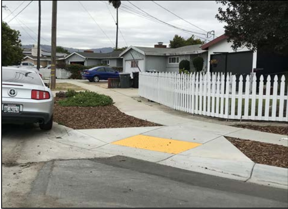
After ADA Ped Ramp at 1231 Summit Dr
