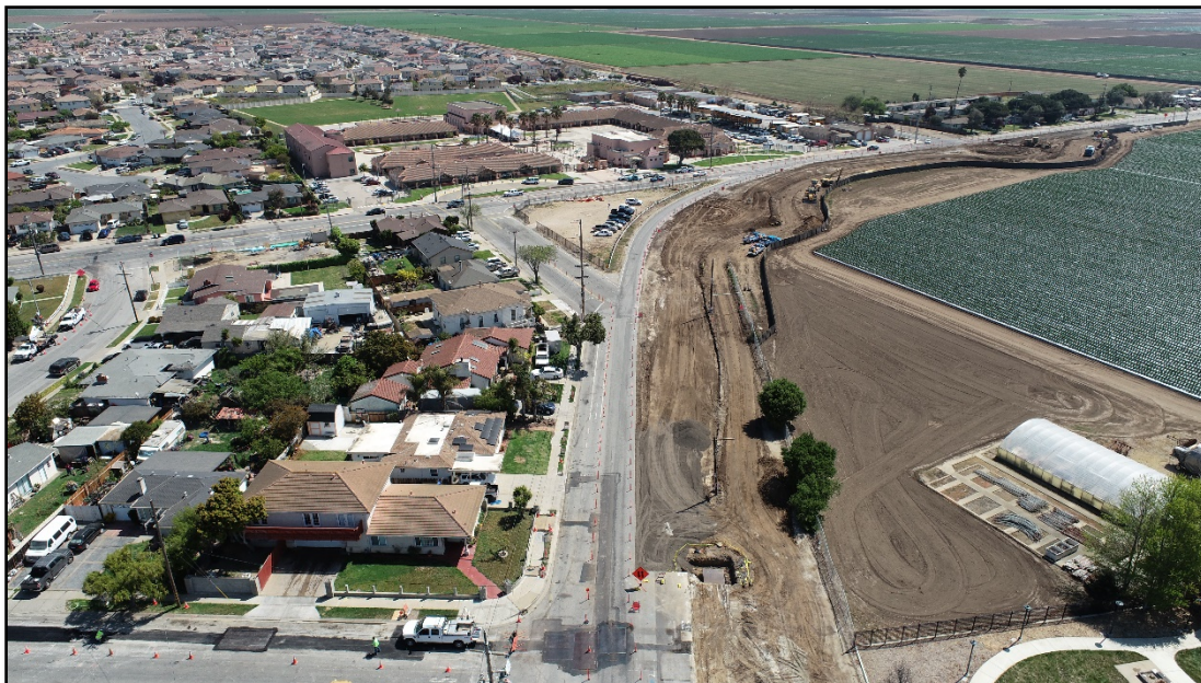
Aerial view of Bardin Road/Alisal St/Alisal Road intersection April 2021
