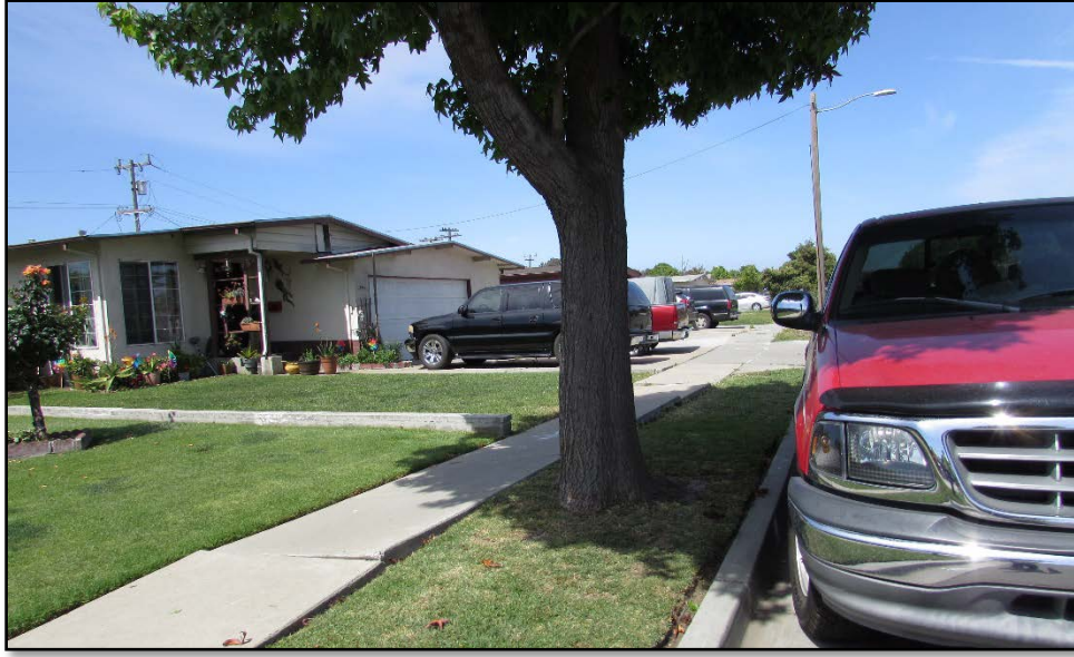
Before photo of John St JOC Sidewalk Repair
