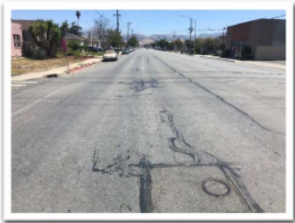
Williams Road @ Quilla Street West Bound facing East
