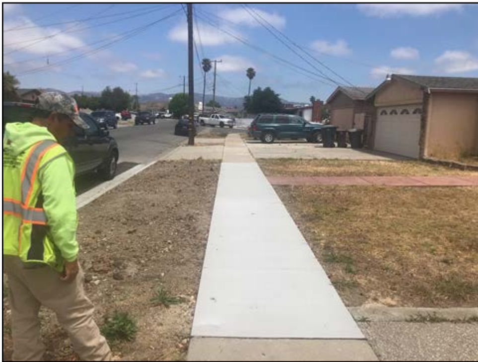
After photos of Summit and Hilltop JOC Sidewalk Repair
