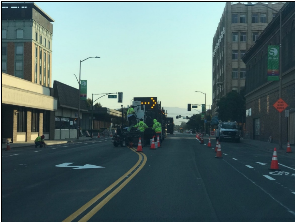
Construction Photo: Pavement Markings and Striping Installation
