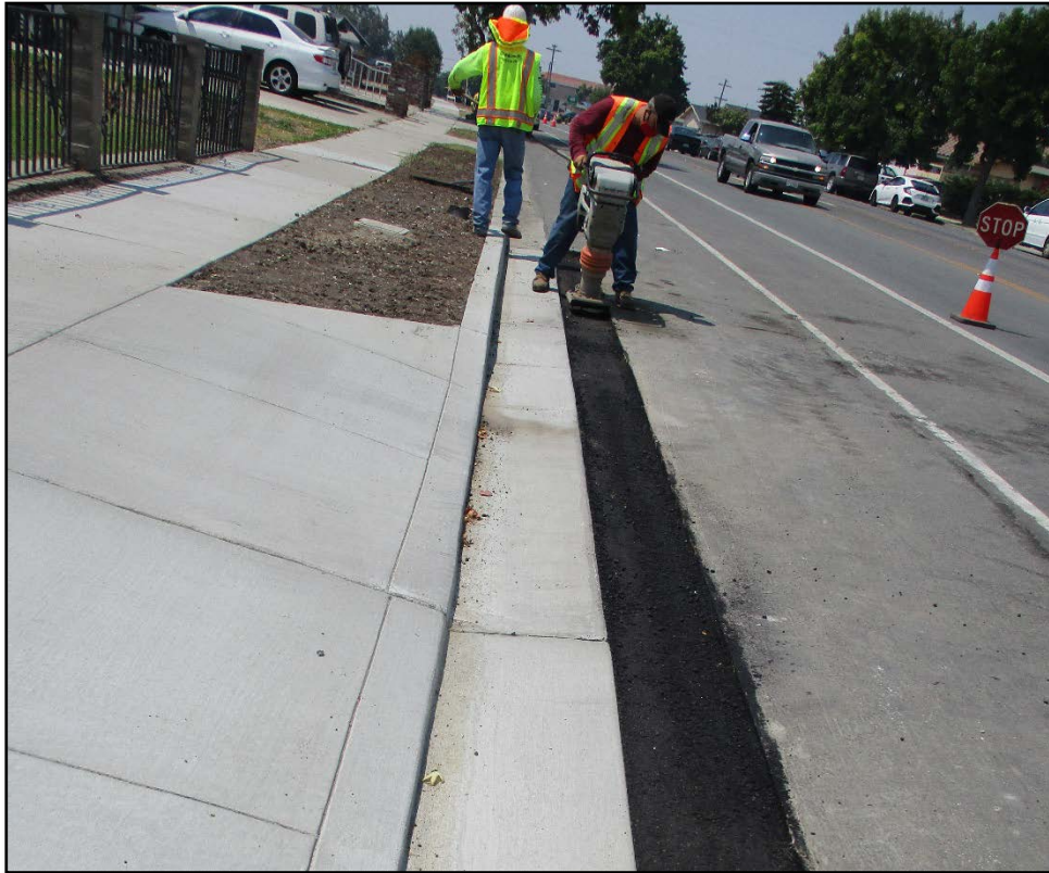
After photo of John St JOC Sidewalk Repair
