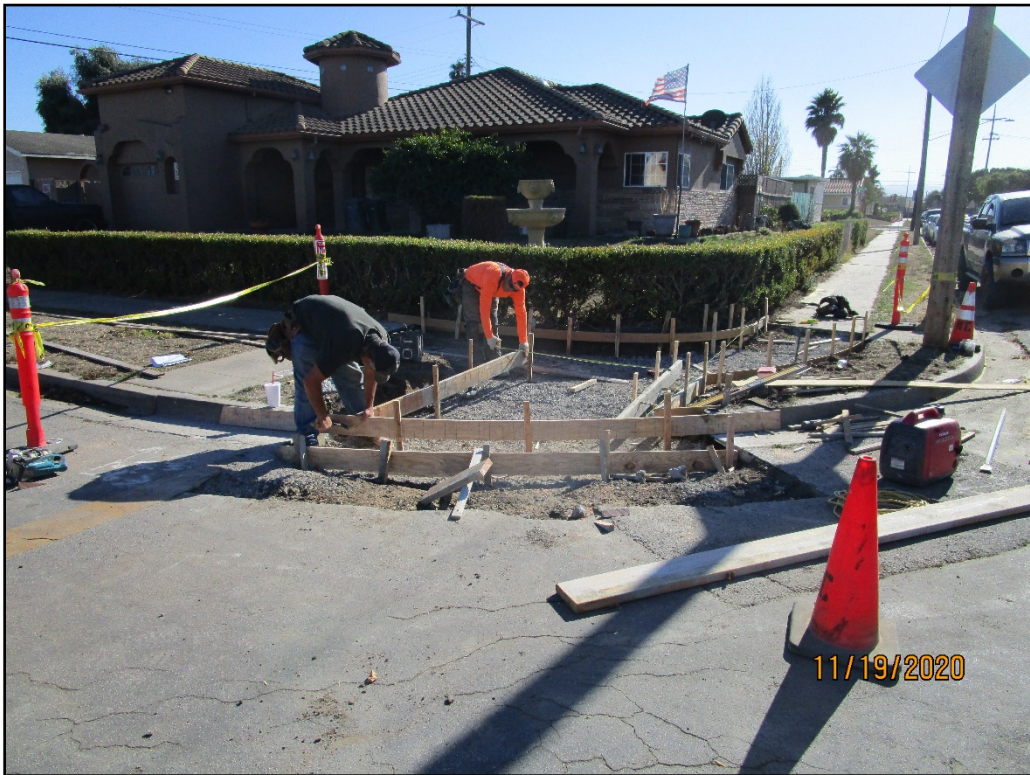
Construction Photo: New pedestrian access ramp on Linwood Drive
