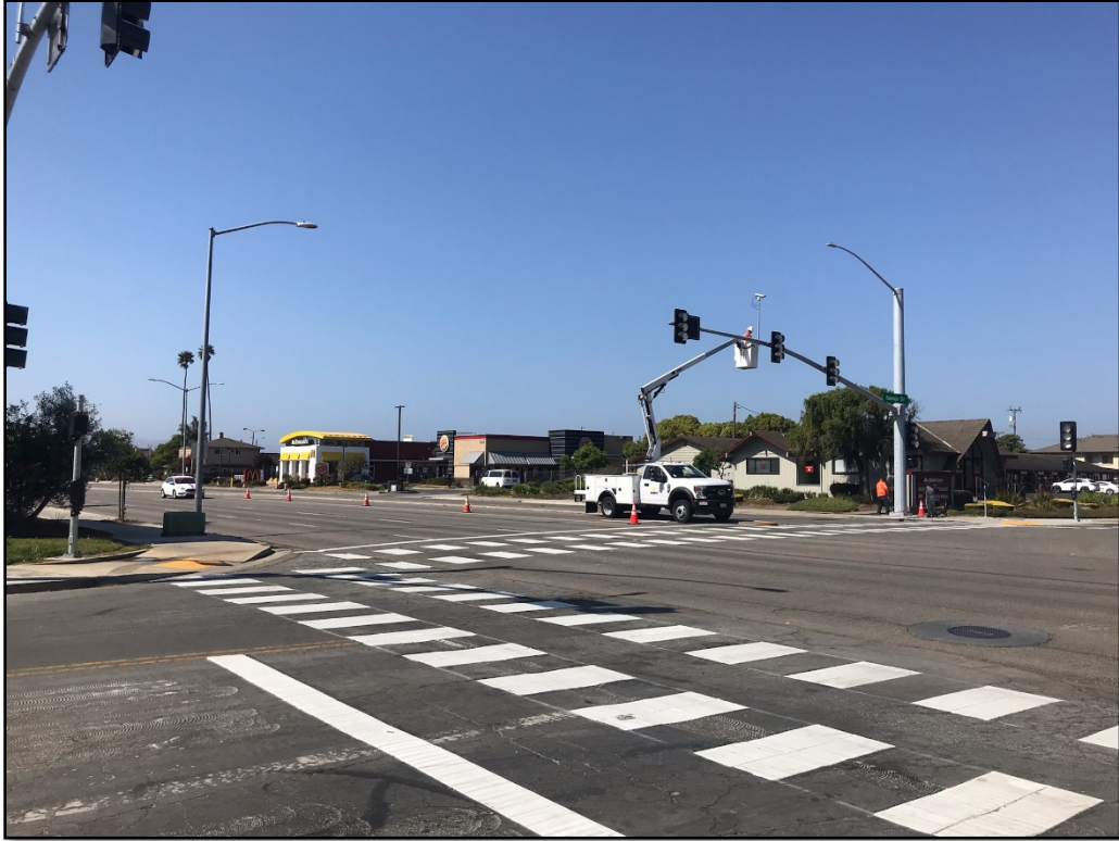
Construction Photo: Installing the Video Detection Cameras
