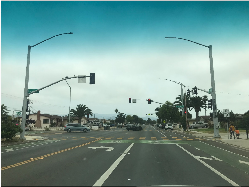
After Construction – New striping and signal on Alvin Dr at El Dorado Dr
