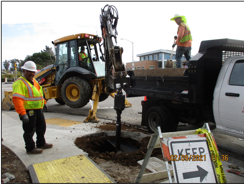
Construction Photo: Augering Pole Foundations
