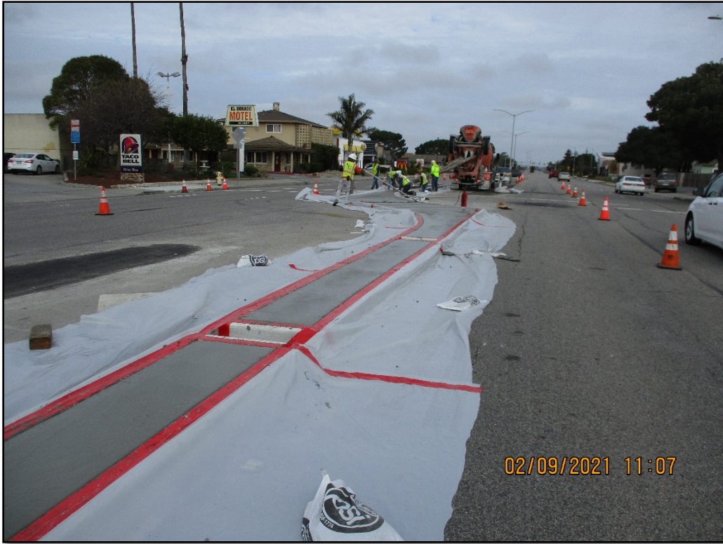
Construction Photo: Pouring the Worm Median Island
