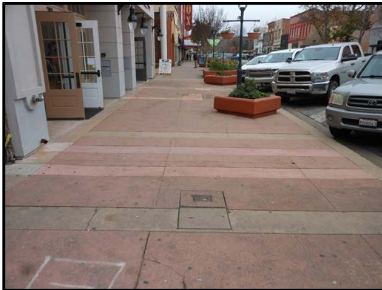
Before: 200 Block Sidewalk Facing South
