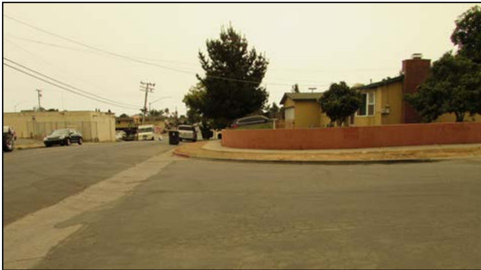
Before ADA Ped Ramp at 990 N Madeira Ave
