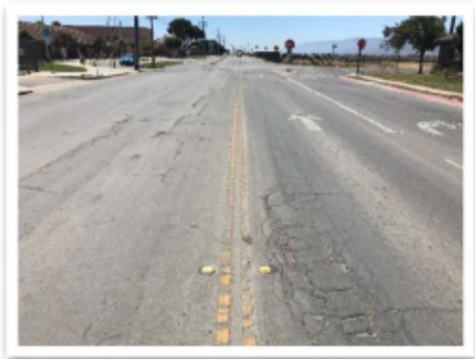
Bardin Road @ ~115' S/O Sycamore Road facing South
