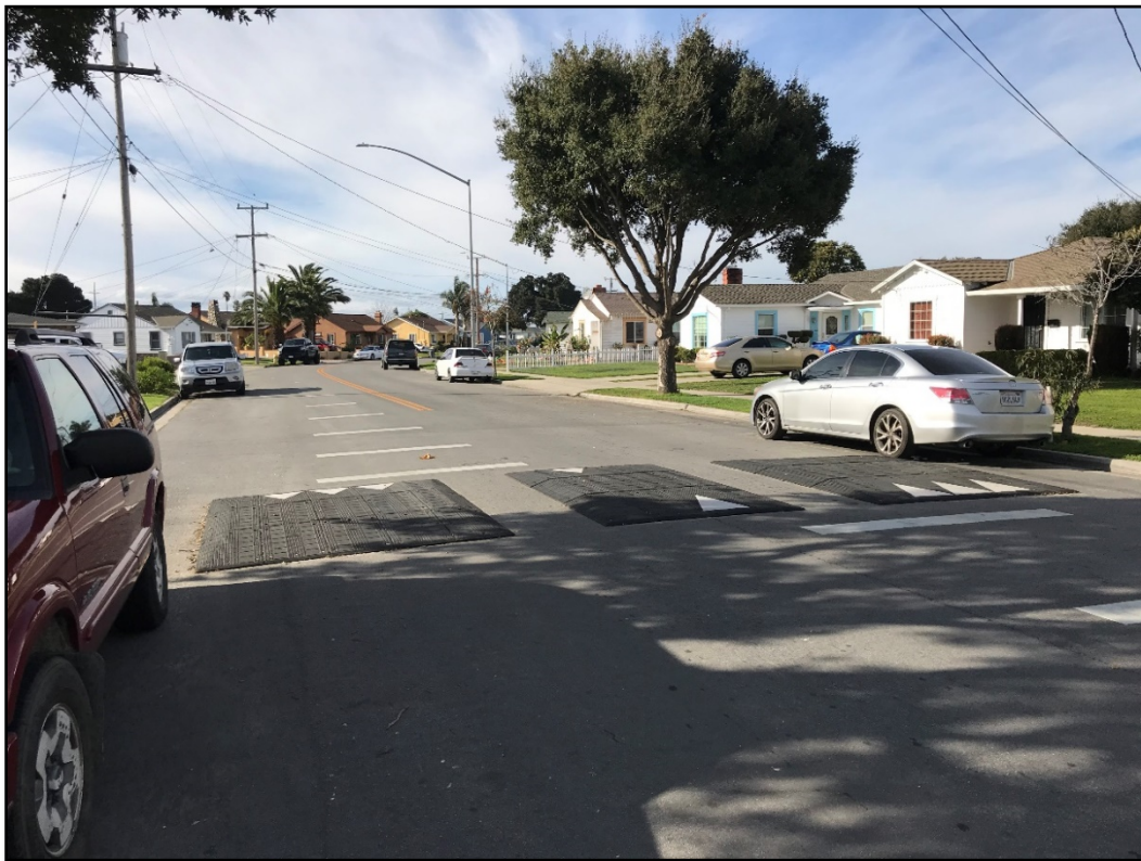
After Photo: First Ave
