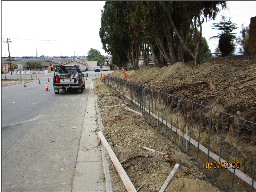
Construction Photo: Maryal Dr Retaining Wall and Sidewalk Work
