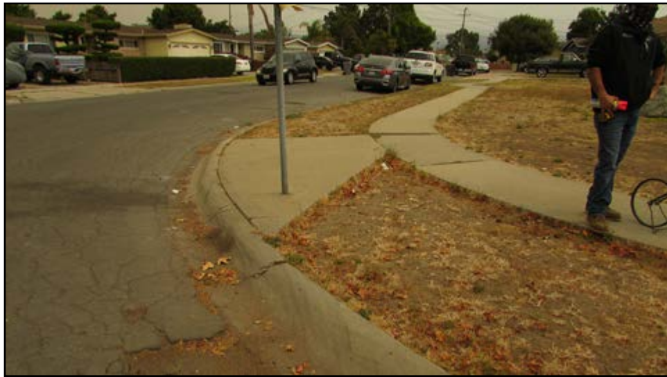
Before ADA Ped Ramp at 1279 Summit Dr
