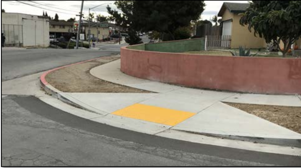
After ADA Ped Ramp at 990 N Madeira Ave
