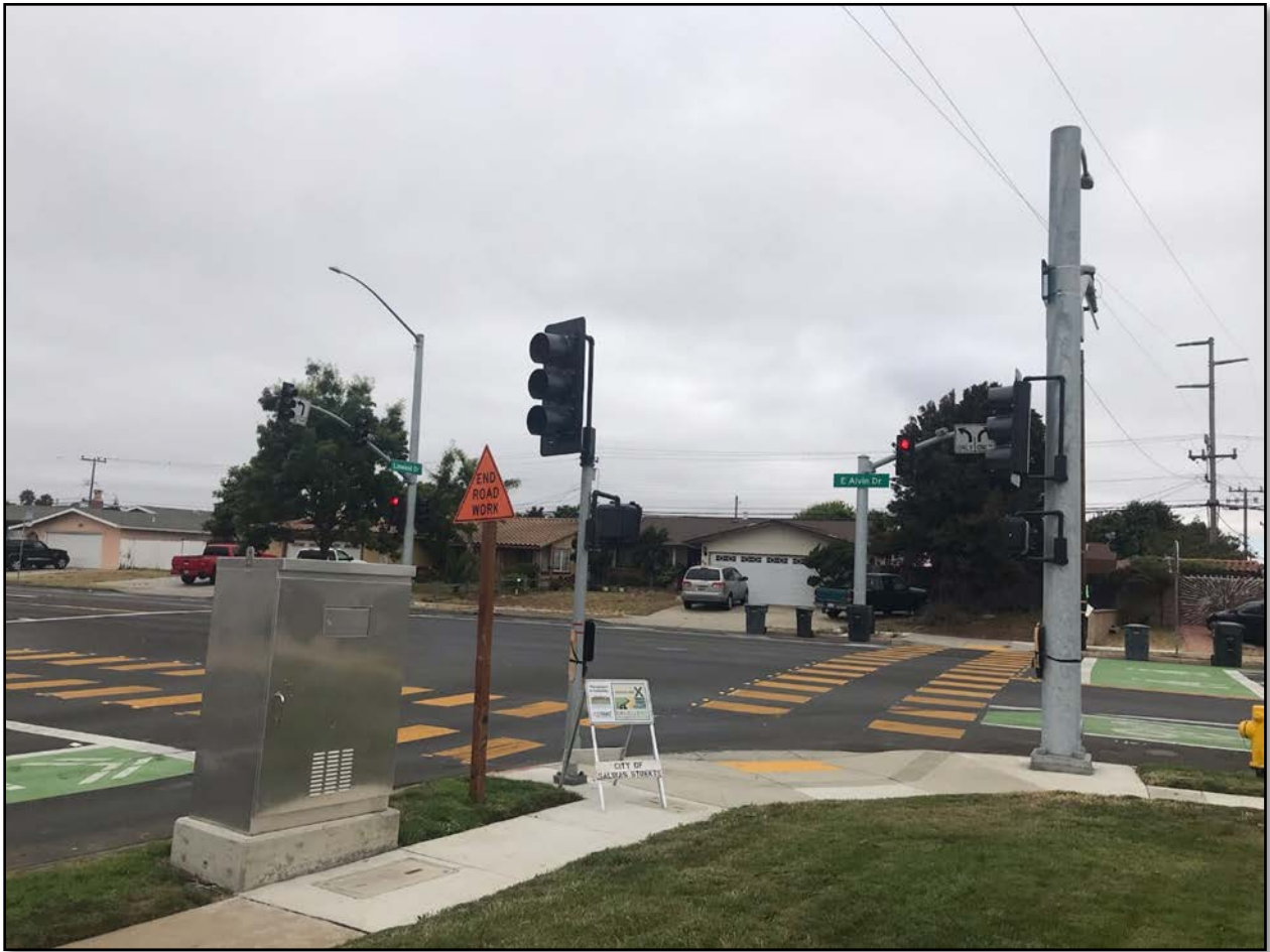
Construction Photo: Nearly Complete Signal at Alvin and Linwood with measure x signage
