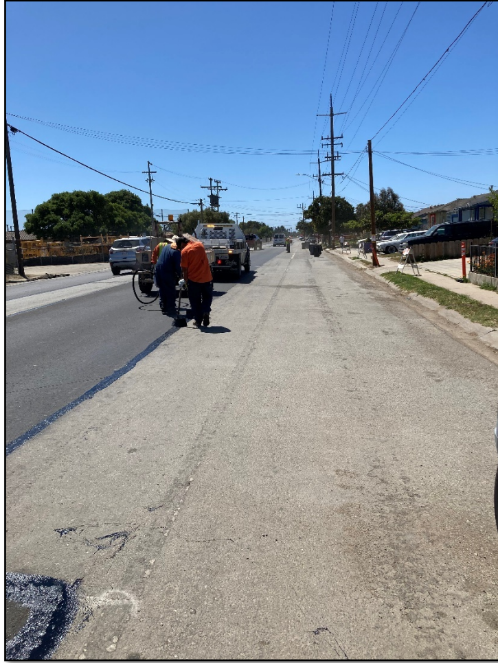
Crack seal work performed at E Alisal St
