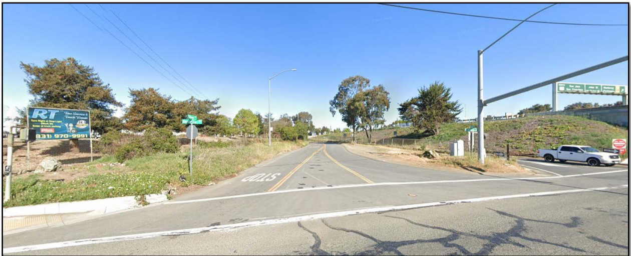
Postconstruction Photo of Sanborn Road/Elvee Drive
