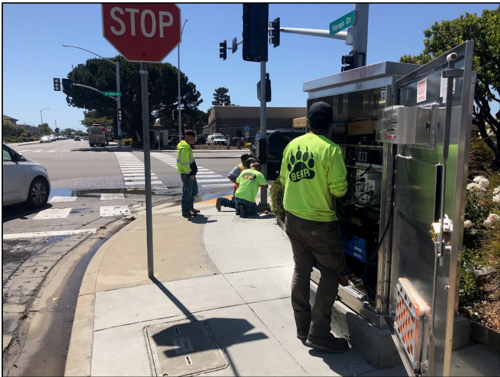
Construction Photo: Cabinet work and Inspection
