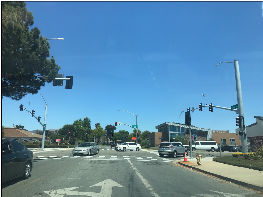
After Construction Photo: New Signal Facing Eastbound
