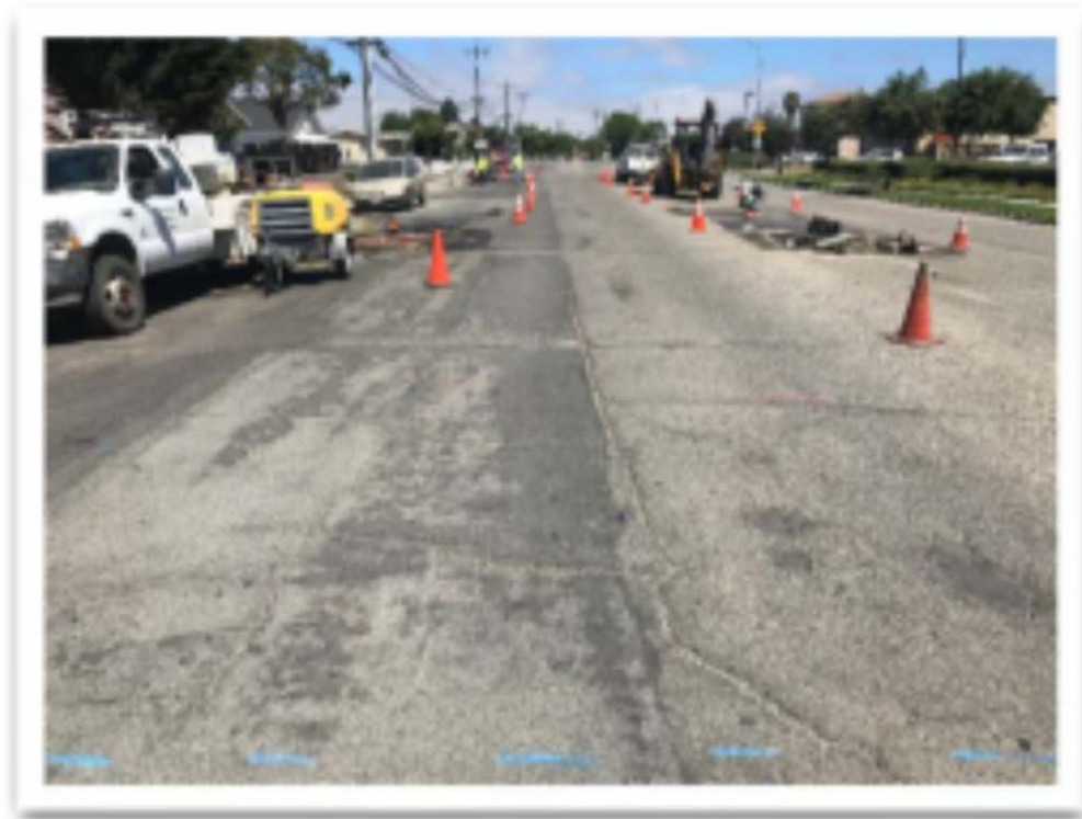
Bardin Road @ Toro Avenue South Bound facing North
