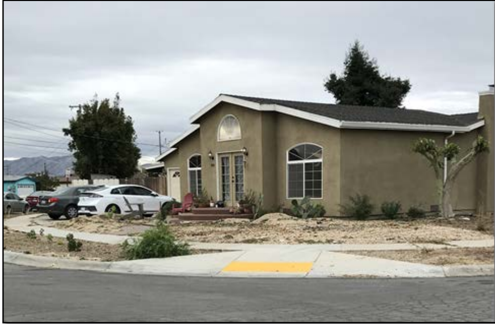
After ADA Ped Ramp at 1274 Summit Dr
