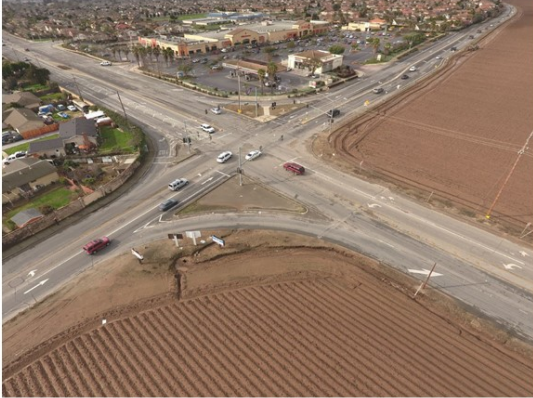
Existing Natividad/Boronda Intersection
