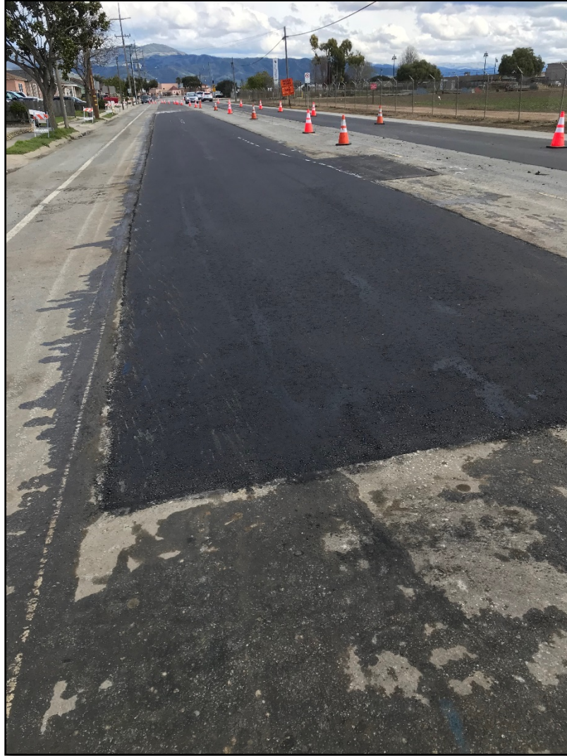
Completed pavement repair at E Alisal St
