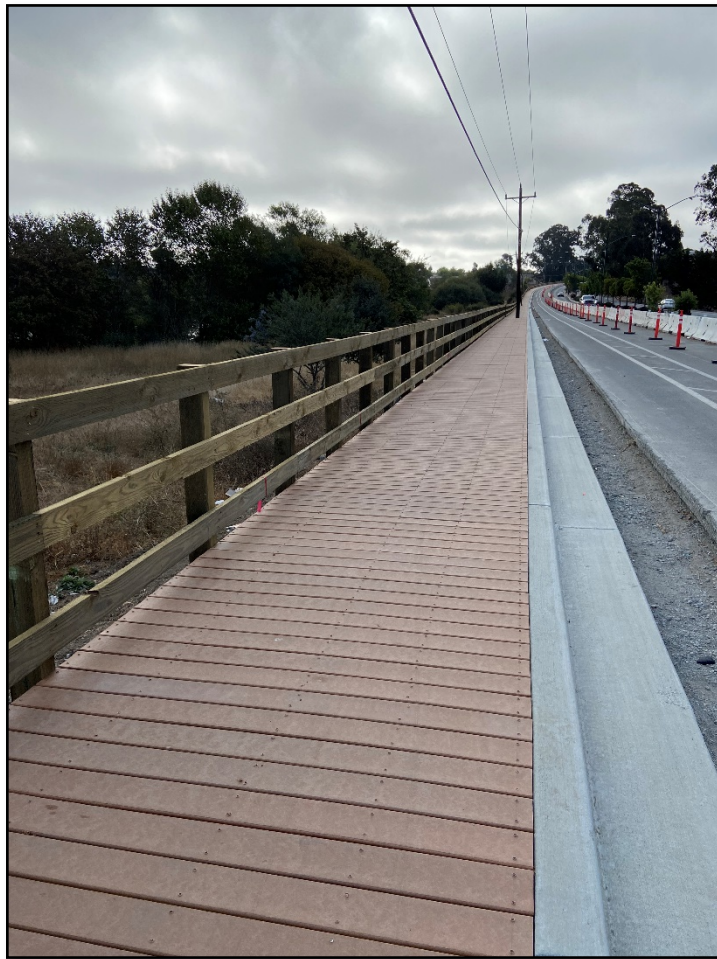
Pedestrian boardwalk completed.
