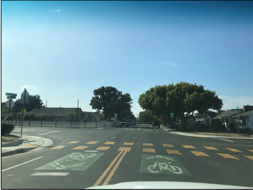
After Construction – New Striping on Maryal Dr
