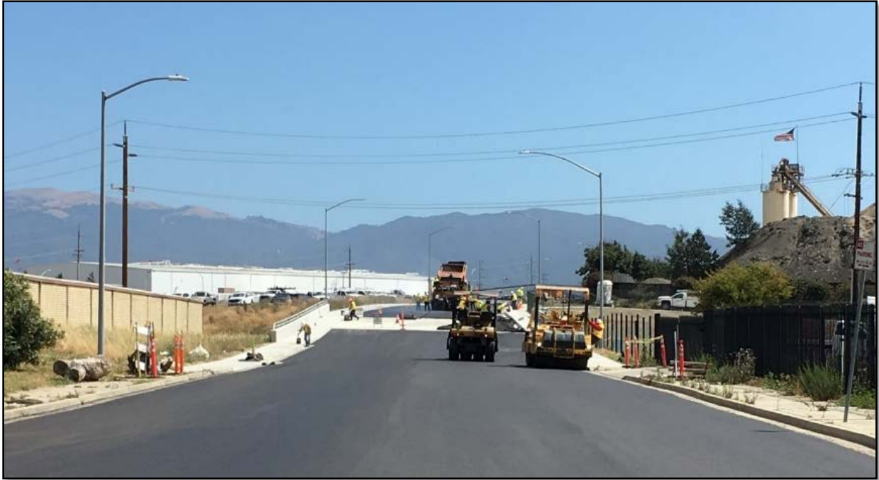
Construction of Elvee Drive Near New Bridge
