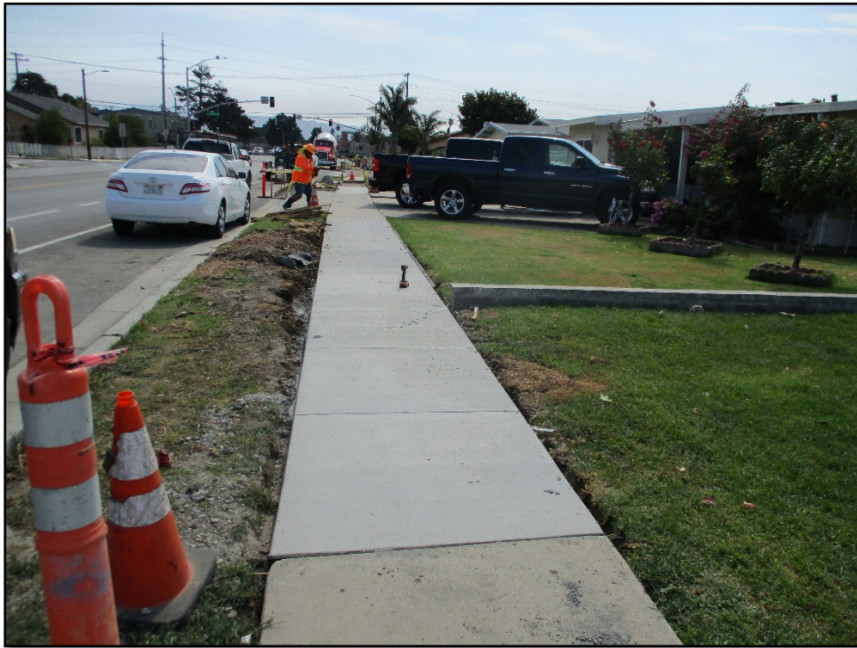
After photo of John St JOC Sidewalk Repair
