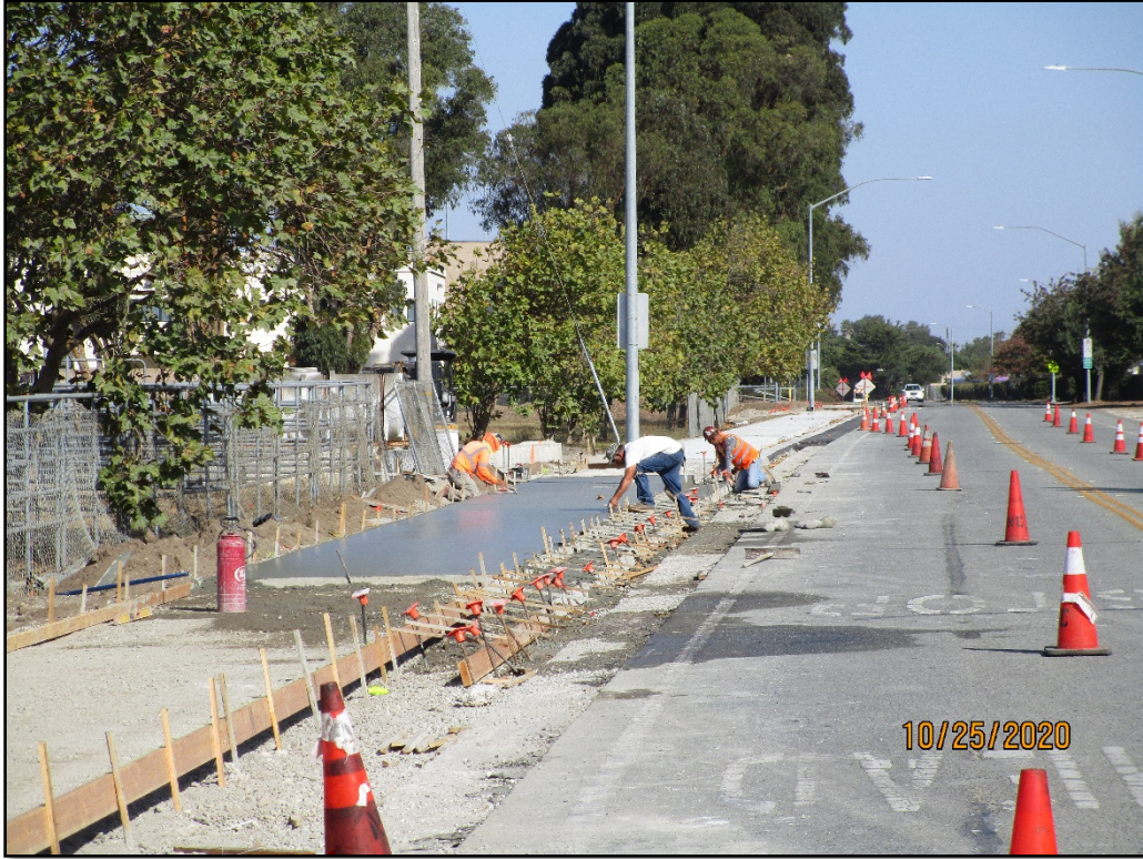
Construction Photo: New Sidewalk on Maryal Drive
