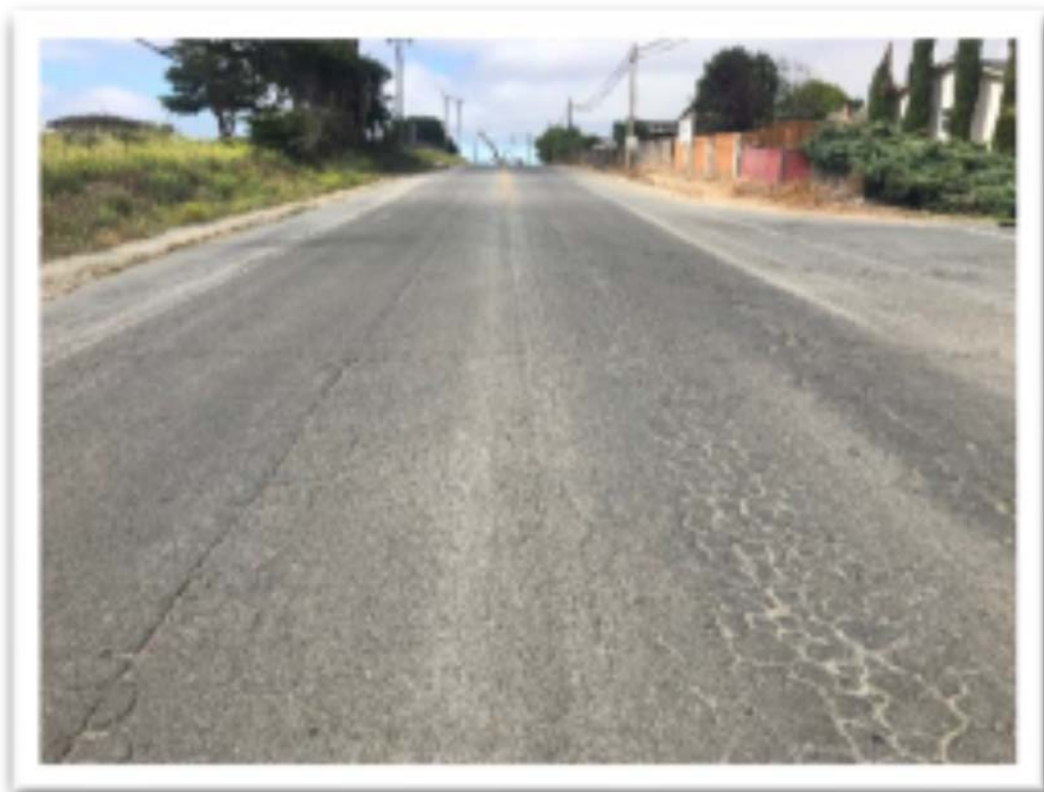
San Juan Grade Road @ Van Buren Avenue facing South
