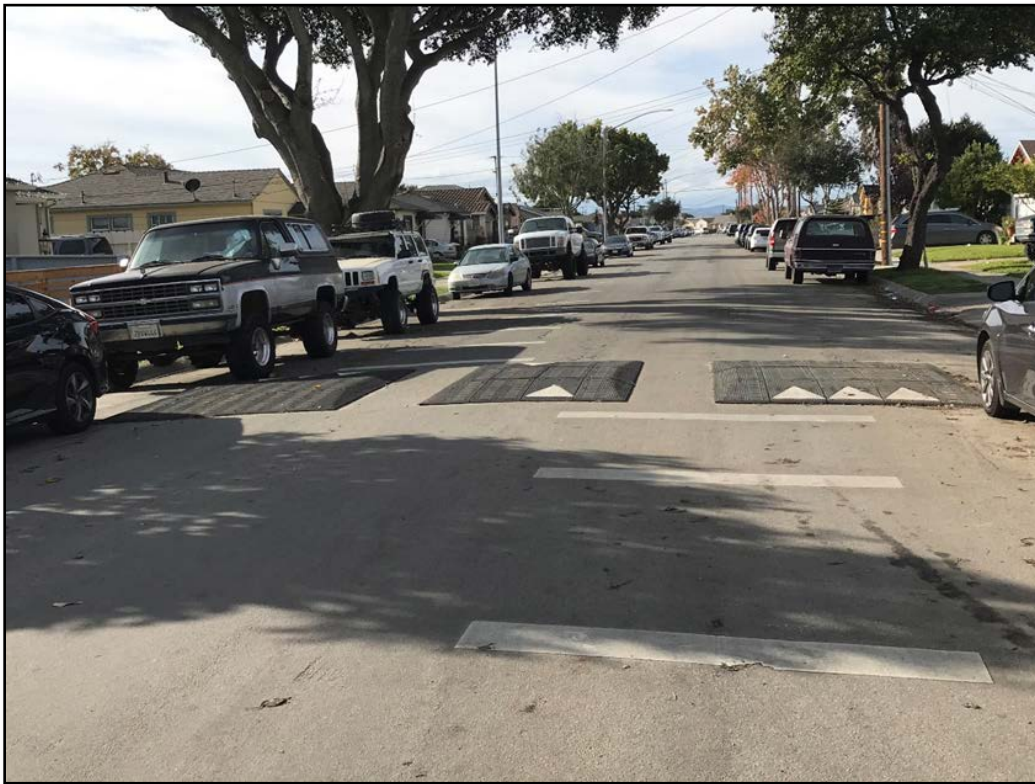
After Photo: First Ave
