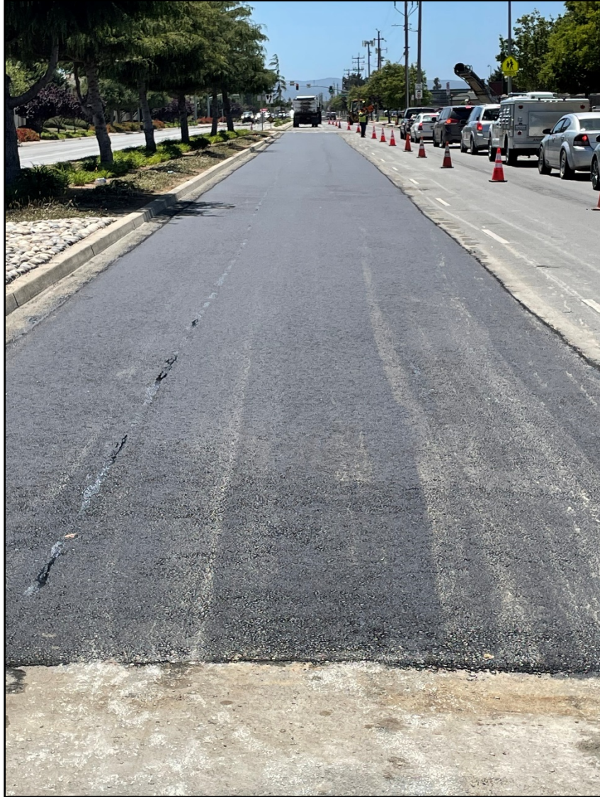
Completed pavement maintenance at Williams Rd
