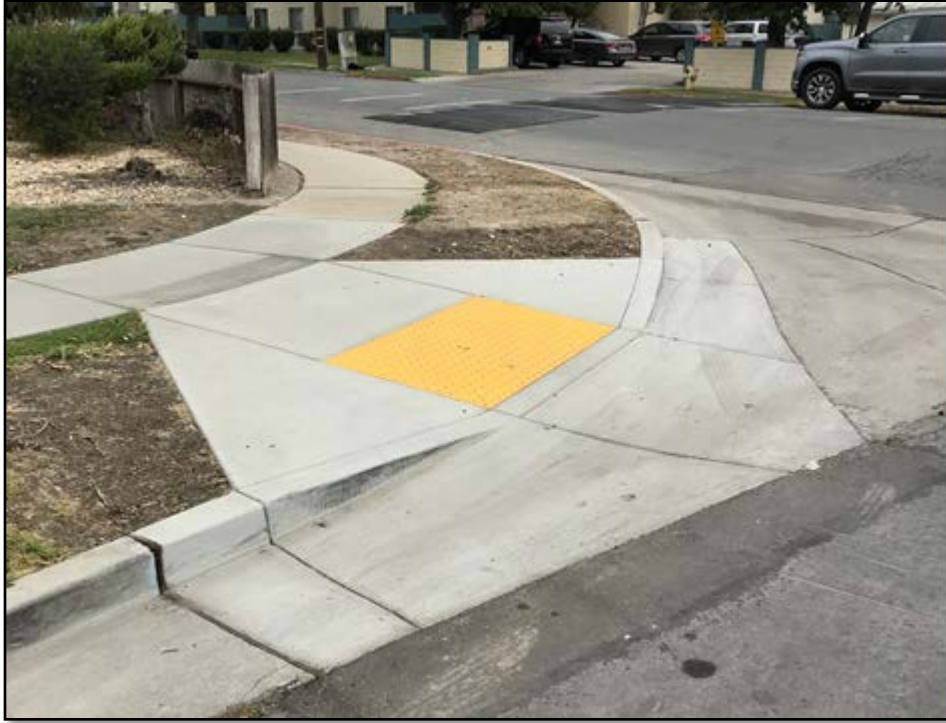
After ADA Ped Ramp at 1296 Hilltop Dr
