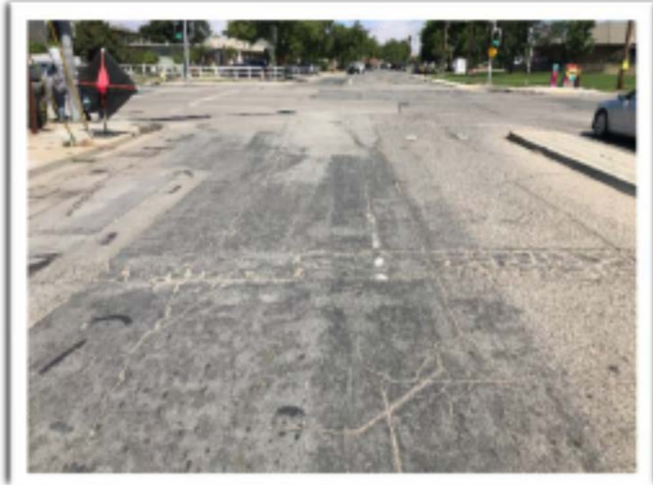
Bardin Road @ Williams Road South Bound facing North
