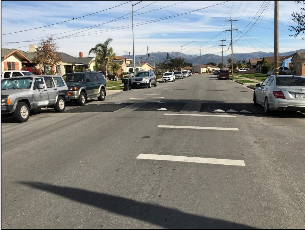
After Photo: First Ave
