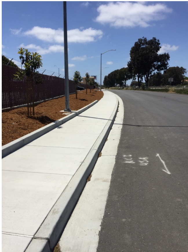
Postconstruction of Elvee Drive Near Sanborn Road
