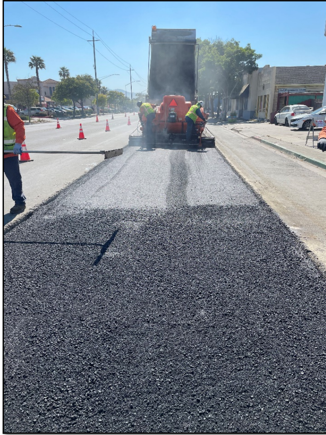
After photo of pavement maintenance work at E Alisal St
