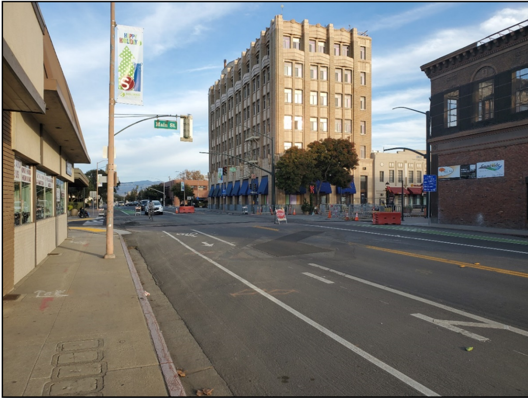
Construction Photo: New Striping and Signal Work at Alisal Street and Main Street
