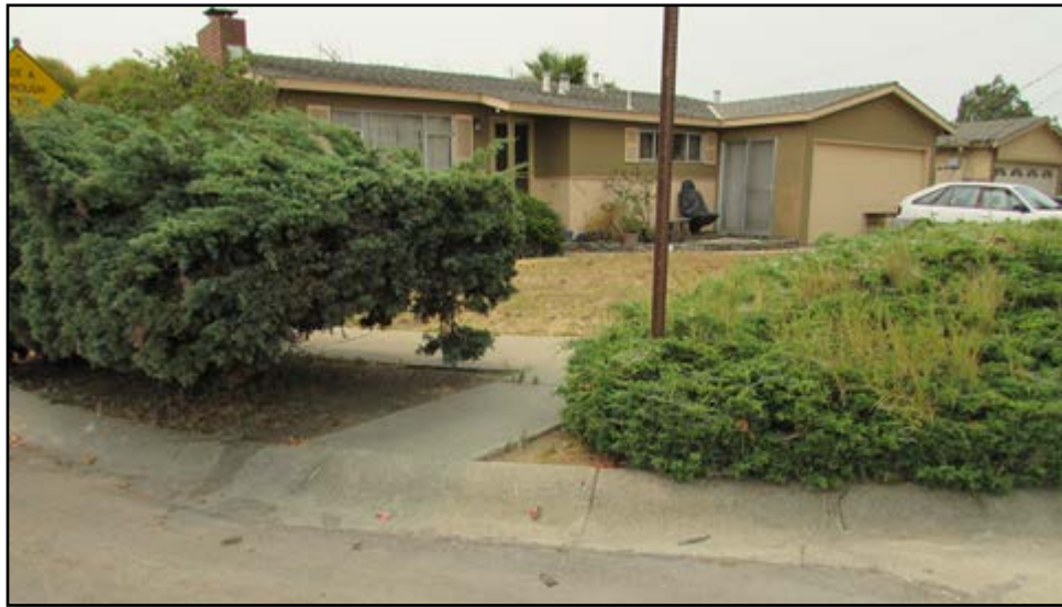
Before ADA Ped Ramp at 1223 Summit Dr
