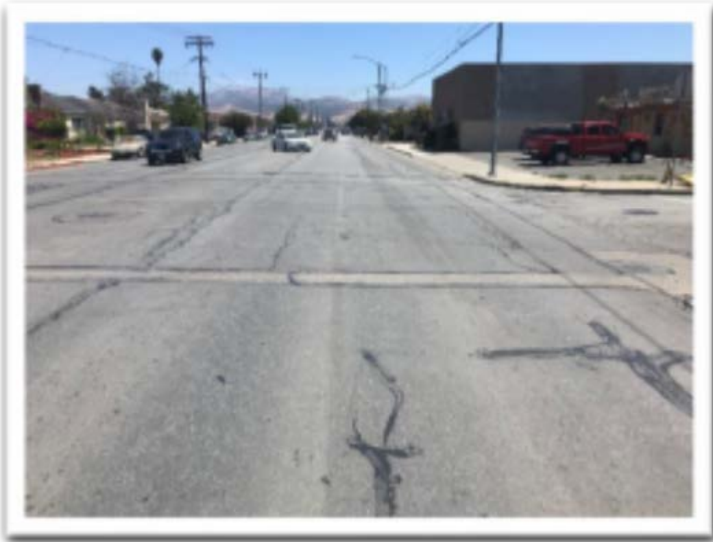
Williams Road @ Quilla Street East Bound facing East
