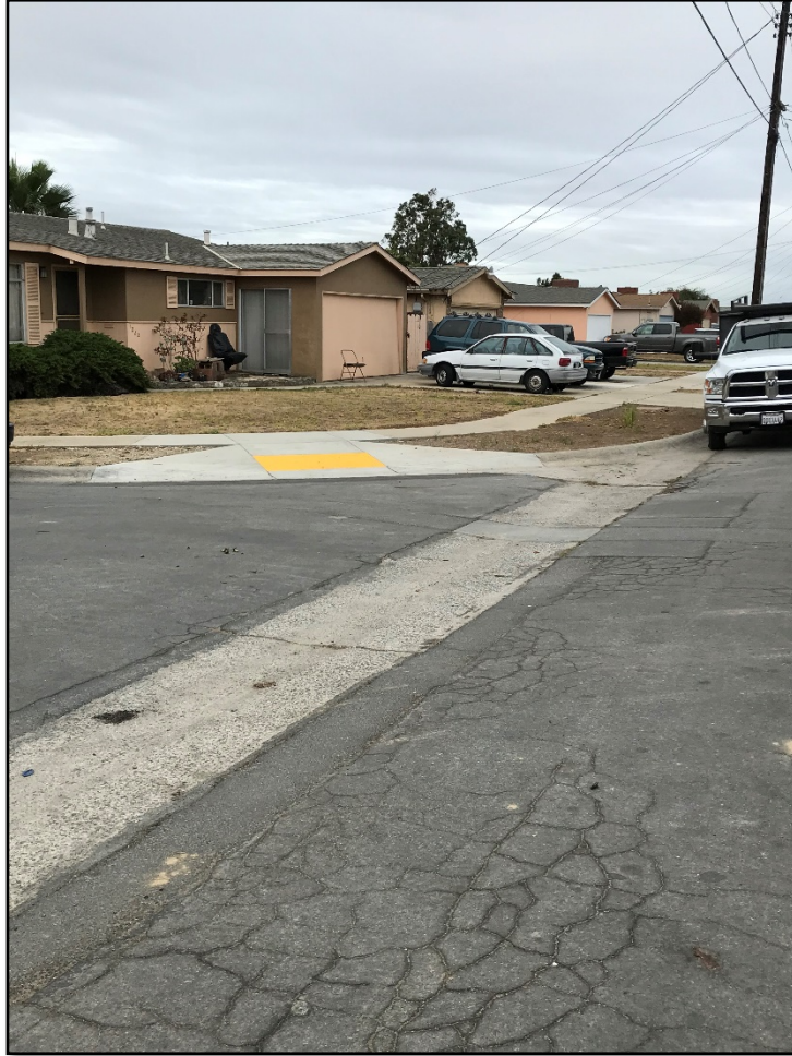
After ADA Ped Ramp at 1223 Summit Dr
