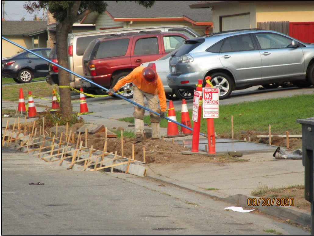
Construction Photo: Sidewalk Repair on East Alvin Drive
