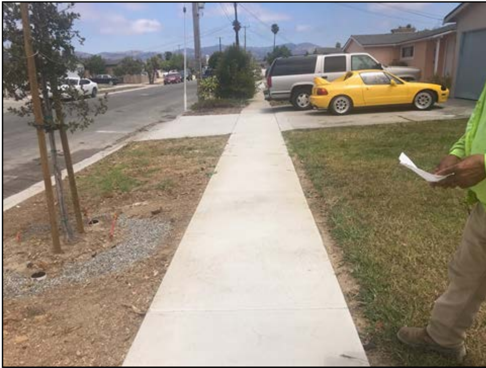
After photo of Summit and Hilltop JOC Sidewalk Repair
