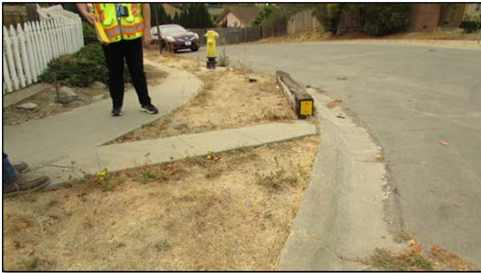
Before ADA Ped Ramp at 1231 Summit Dr
