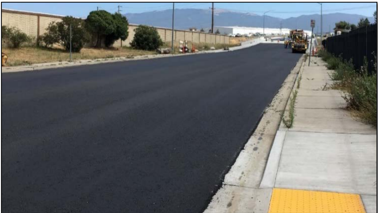
Construction Photo of Elvee Drive Near Work Street
