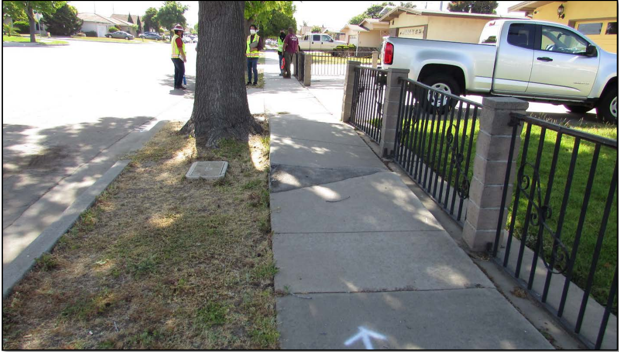
Before photo of John St JOC Sidewalk Repair
