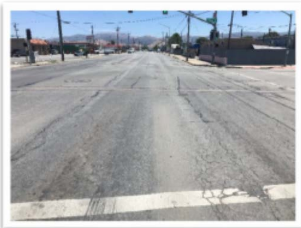
Williams Road @ E. Market Street East Bound facing East
