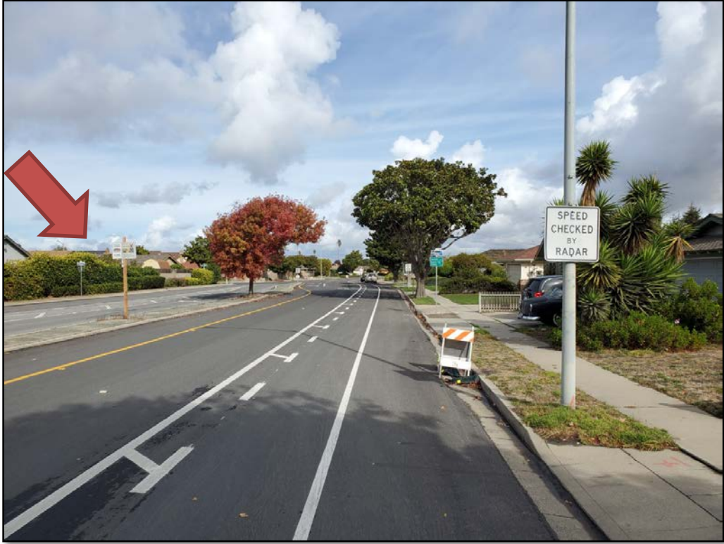
Construction Photo: Final Striping Installation, with Measure X Sign Displayed
