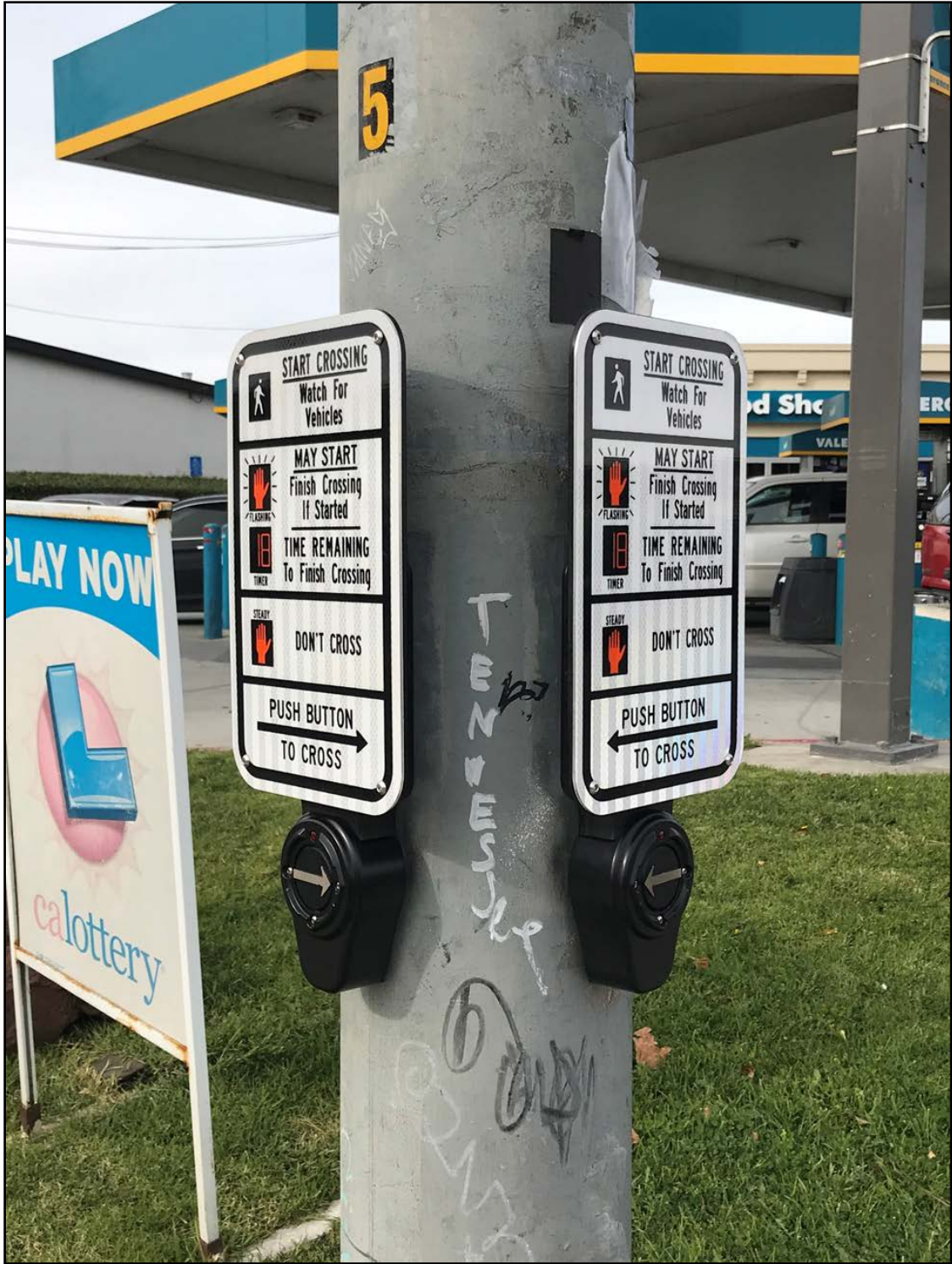
After Photo: Accessible Pedestrian Push Button at Laurel Drive and Main Street
