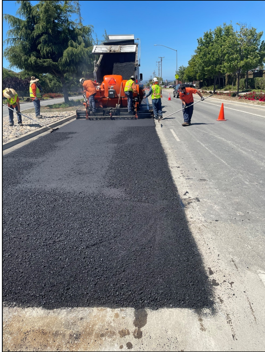
Pavement maintenance work at Williams Rd
