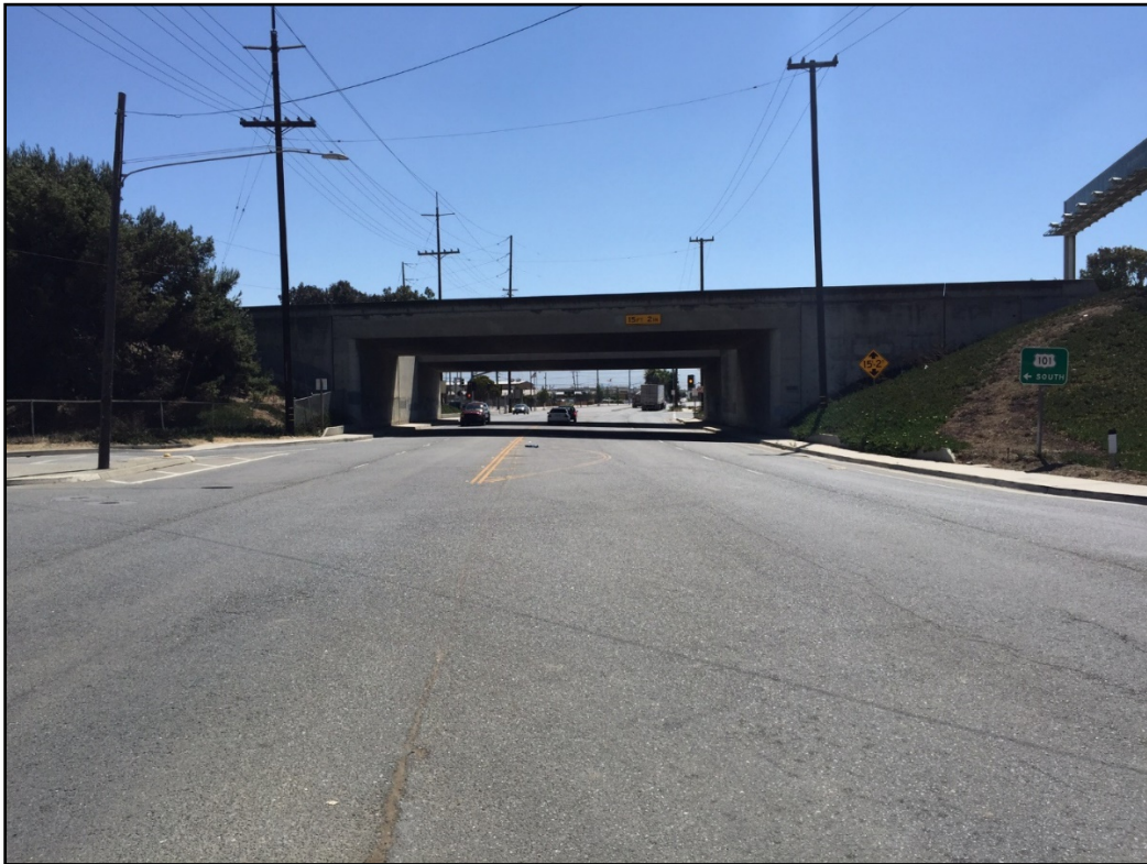
Preconstruction Photo of Sanborn Road near Fairview Avenue
