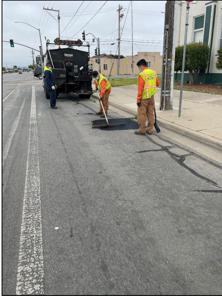
Patch repair work performed at Williams Rd
