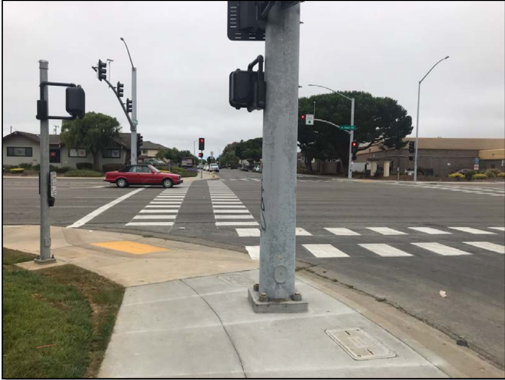
After Construction Photo: New Signal facing Westbound
