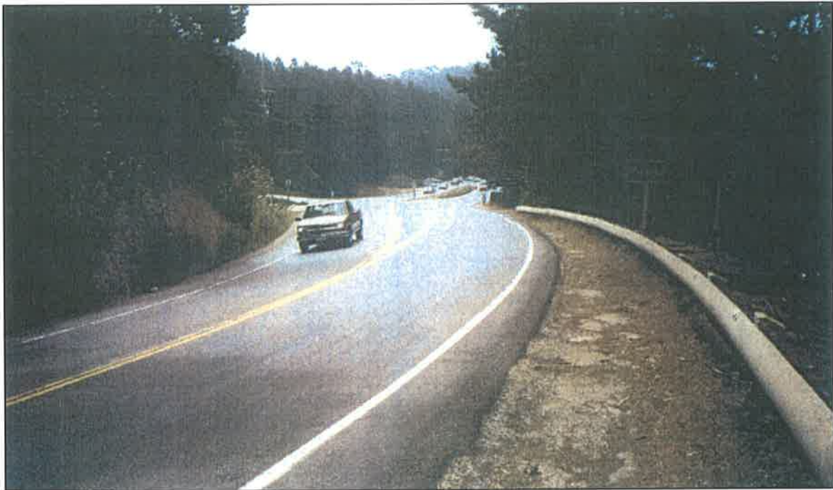
Figure 5-4. Viewpoint 3 - SR 68 Eastbound, View to the East
