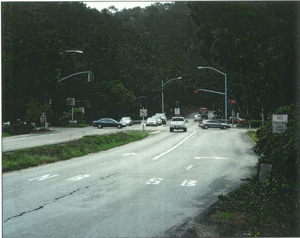
Figure 5-2. Viewpoint 1 – SR 68/SR 1 Southbound Ramp Intersection, View to the East
